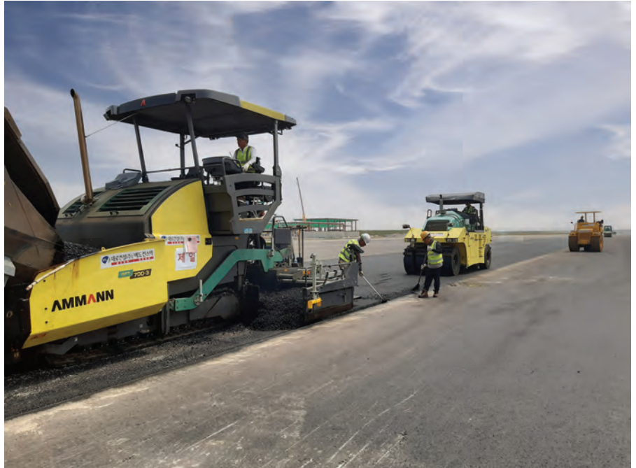
ALL IMAGES: Daero Construction recently carried out paving work on a road in Seosan City, 120-km south of Seoul. To help deliver the job, the company opted for an Ammann AFT 700-3 large premium tracked paver.
