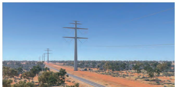
Another component of the project is a high voltage direct current (HVDC) overhead transmission line (OHTL) from the solar farm to Darwin.
