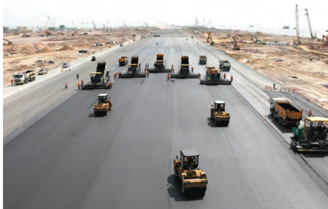
TOP: The three-runway system reclamation works have been substantially completed.
