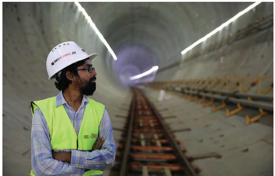
As this is the first tunnel in the country, SMEC is also training and developing the next generation of Bangladesh’s tunnel engineers.
