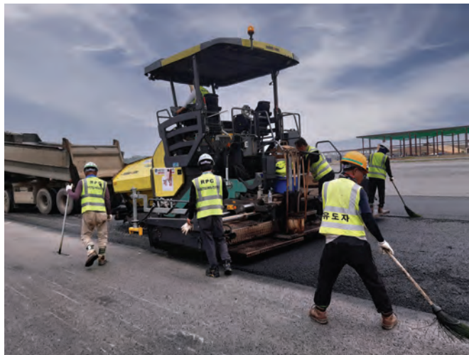
ALL IMAGES: Daero Construction recently carried out paving work on a road in Seosan City, 120-km south of Seoul. To help deliver the job, the company opted for an Ammann AFT 700-3 large premium tracked paver.
