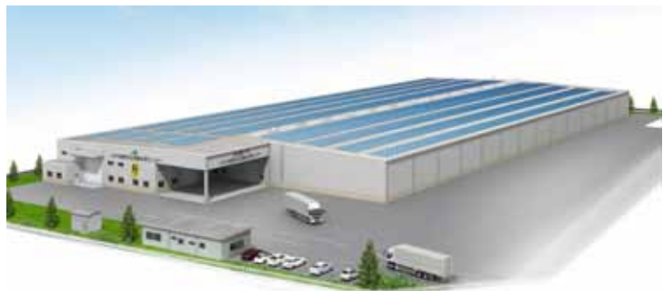
Image of a solar power generating system on a Zen-Noh Group logistics centre in Hanamaki, Iwate Pref., Japan (approx. 800kW).
