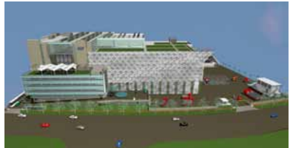
Artist's impression of SEF Group's first Integrated Construction and Precast Hub (ICPH) at Kaki Bukit. Image: © SEF Group Ltd
