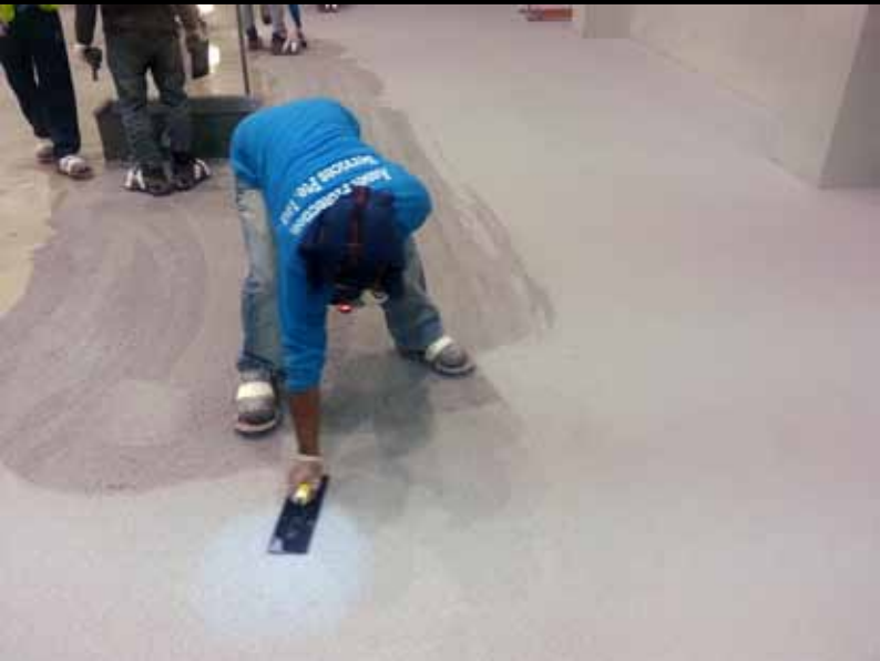
Application of Sika® DecoQuartz.
