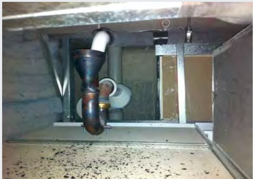
A view of the ceiling cavity, where the problem was located.
