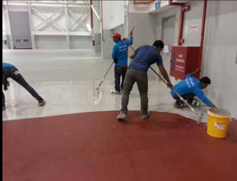
Application of Sikafloor® 81 EpoCem.
