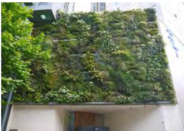
Fytogreen's green wall installation for Triptych apartments in Melbourne in 2010. Photo: © Fytogreen
