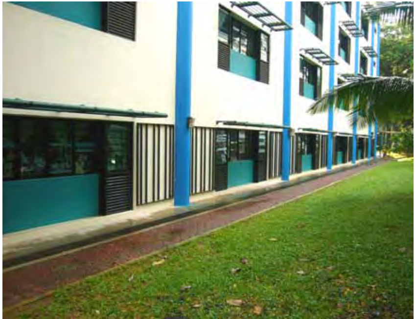
Before the green wall installation. Photo: © Prince's Landscape & Construction Pte Ltd
