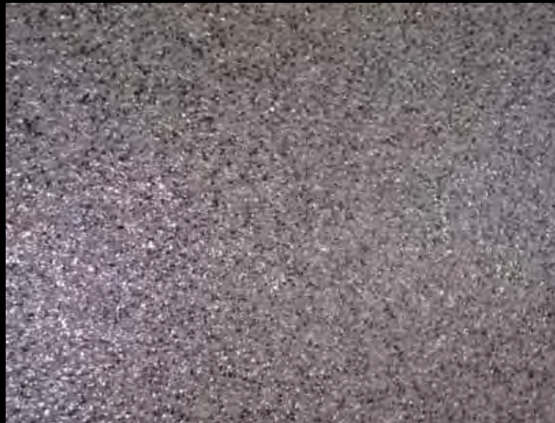
Image of the finished floor showing Sika® DecoQuartz.
