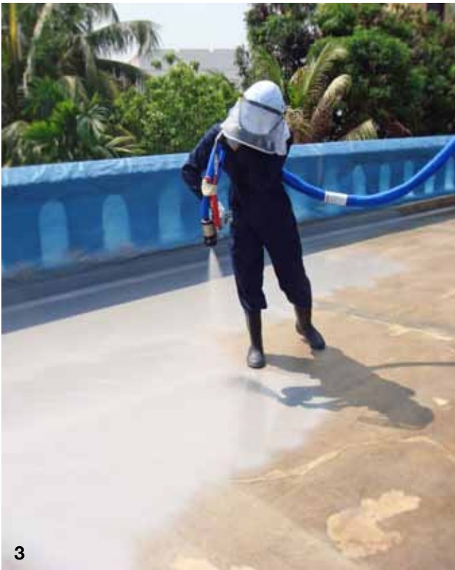
Photo 1: Roof deck ready for Purtop 400 M application after surface preparation, crack repairs and priming.
