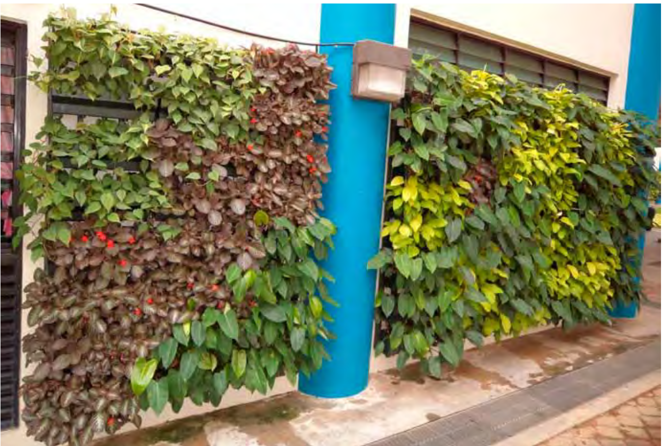
Green wall installation completed. Photos: © Prince's Landscape & Construction Pte Ltd
