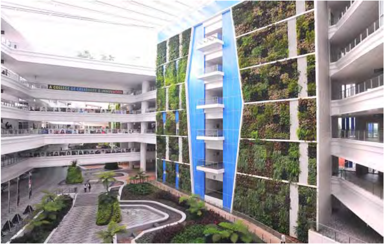
The Central Green Spine showcases extensive green walls.
