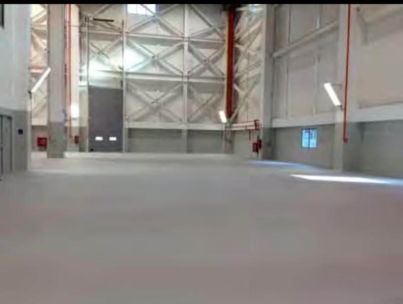
Finished floor at the preparation area and control block.
