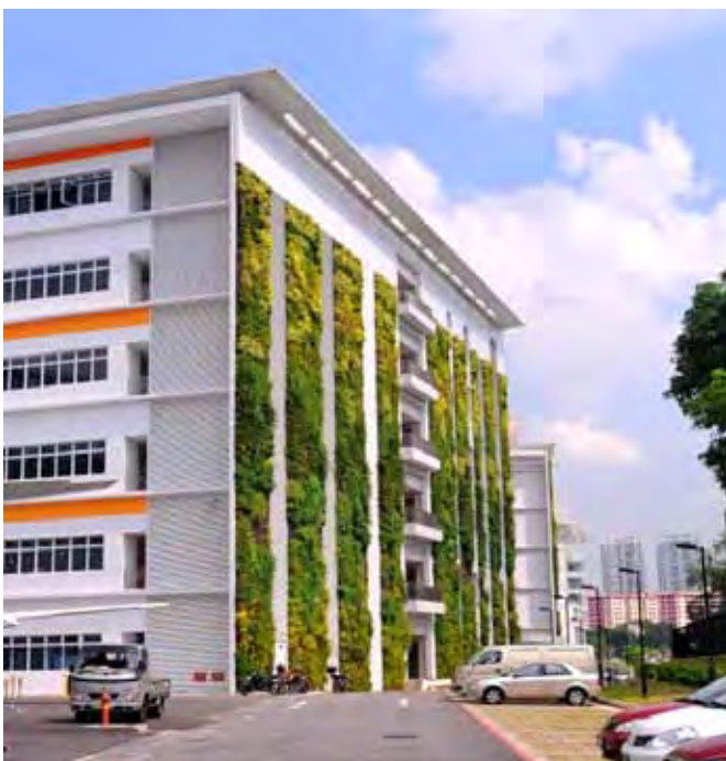
View of green walls along exterior building blocks of H, J, and K.
