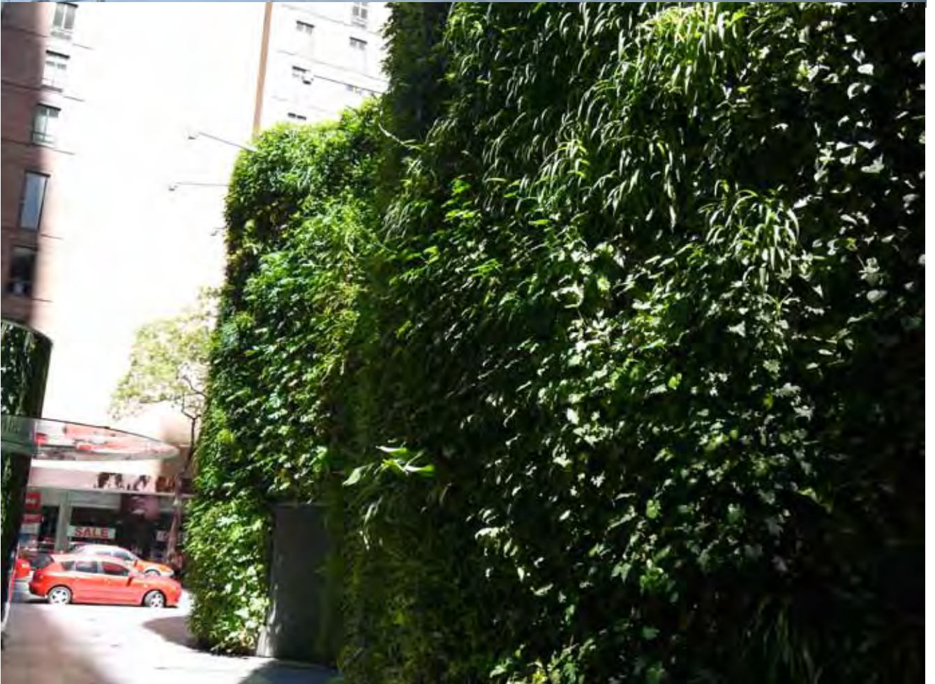
Fytogreen supplied vertical gardens for 1 Bligh Street in Sydney, Australia. Photos: © Fytogreen
