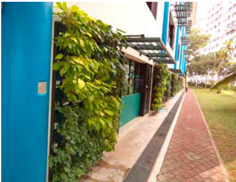
Staff from Prince's Landscape installing the green wall. Photo: © Prince's Landscape & Construction Pte Ltd
