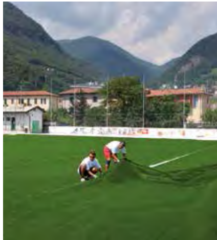
Positioning synthetic grass rolls.
