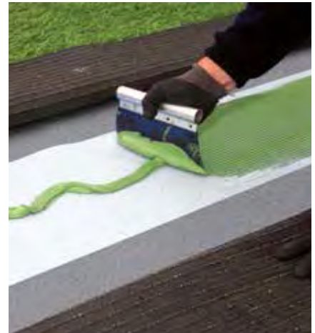
Spreading adhesive on ULTRABOND TURF TAPE 100 using a notched trowel.
