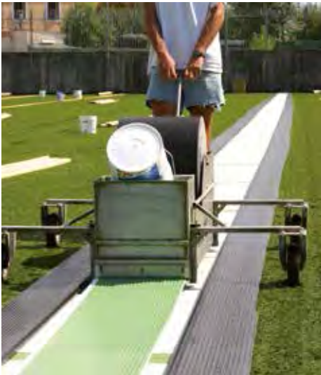
Spreading the adhesive with a manual applicator.
