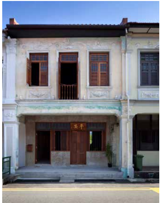
North Canal Road conserved shophouses faithfully reinstated. Photo: © Urban Redevelopment Authority
