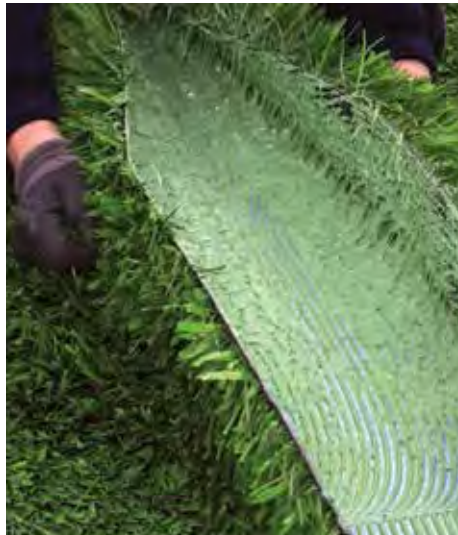
Checking the buttering on the back of the grass surface.
