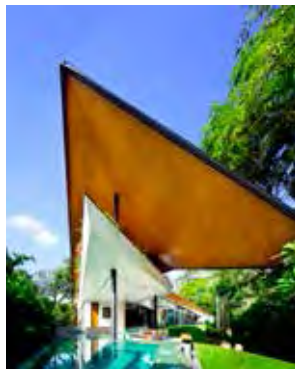
The Winged House. Photo: © SIA and K2LD Architects Pte Ltd
