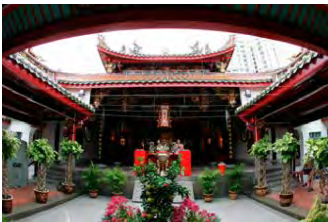
Main hall of 30 Mohamed Sultan Road (Hong San See Temple) restored. Photo: © Urban Redevelopment Authority
