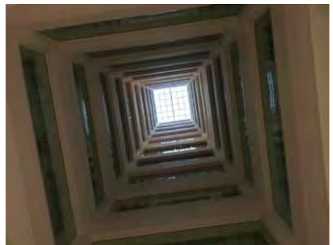
An interior atrium provides natural daylight for all the office spaces.
