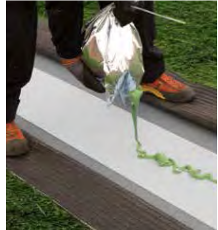
Application of ULTRABOND TURF PU 1K on the jointing tape, via extrusion from its aluminium package.
