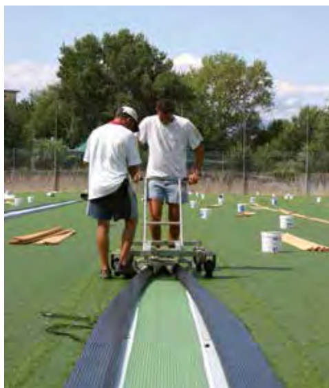
Bonding the edges of the synthetic grass with a manual applicator.
