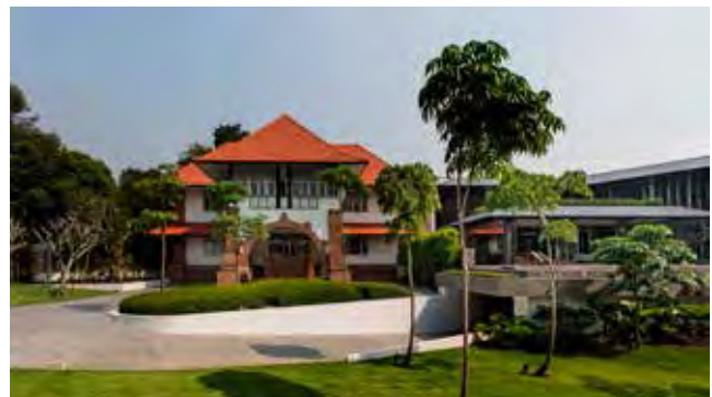
5 Chatsworth Park iconic Frank Brewer bungalow restored. Photo: © Urban Redevelopment Authority
