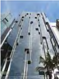
137 Market Street. Photo: © SIA and Teh Joo Heng Architects
