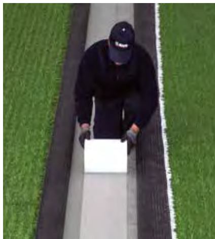
Laying the ULTRABOND TURF TAPE 100 jointing tape.
