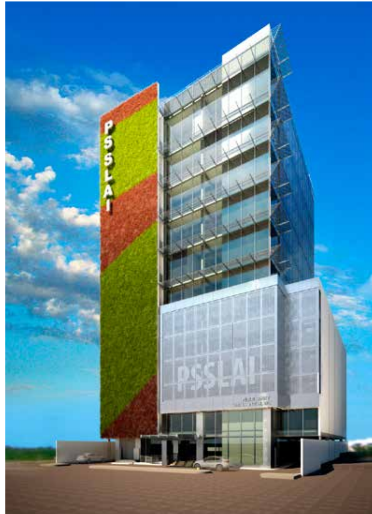
The Public Safety Savings and Loan Association Inc. headquarters along EDSA incorporates a 12 storey high green wall, among the tallest in the region. Meant to help reduce the carbon dioxide emissions generated by vehicles along a busy thoroughfare, it uses recycled rainwater for irrigation.
