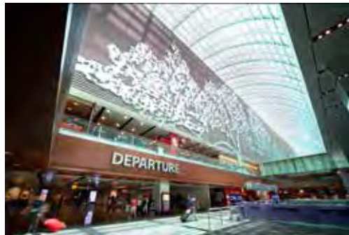
Changi Airport Terminal 1 Upgrading. Photo: © SIA and Architects 61 Pte Ltd
