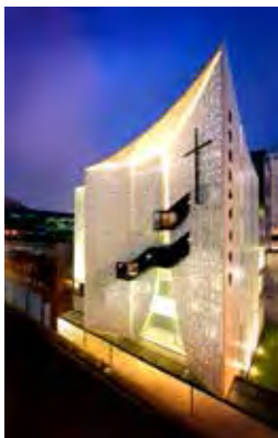
Singapore Life Church. Photo: © SIA and LAUD Architects Pte Ltd
