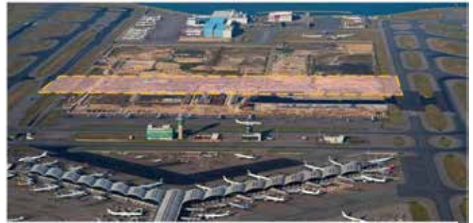
Project extension within Airport Midfield Area.
