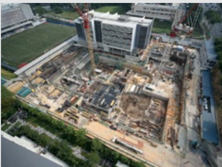
Overview of the Stamford American school.
