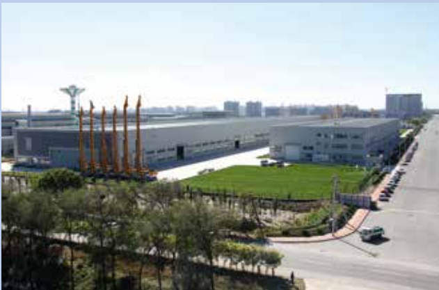
Bauer has moved to its new, larger facility in the Xiqing district in Tianjin. ■
