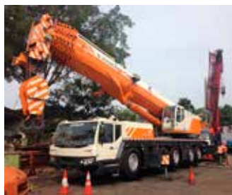
ALL TERRAIN CRANE
