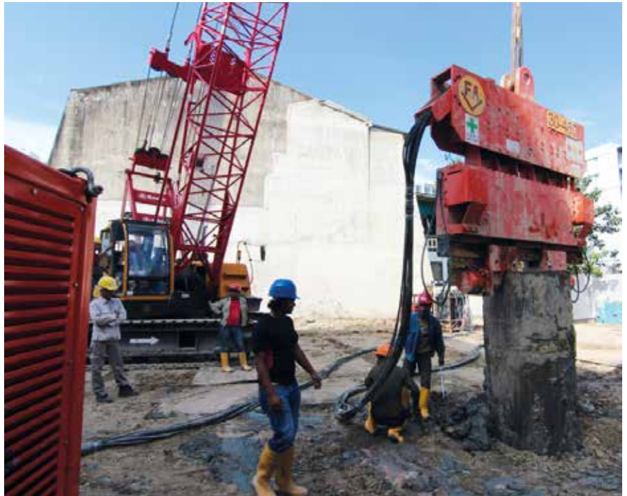
Above and below: The FAV 30-400 hydraulic vibro hammer from Foundation Associates Engineering has an improved eccentric moment of 30 kgm with a greater centrifugal force of 1,069 kN.
