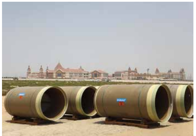
Top and above: The HOBAS CC-GRP jacking pipes have played an important role in the The Nad Al Sheba 4 Sewage & Drainage project.
