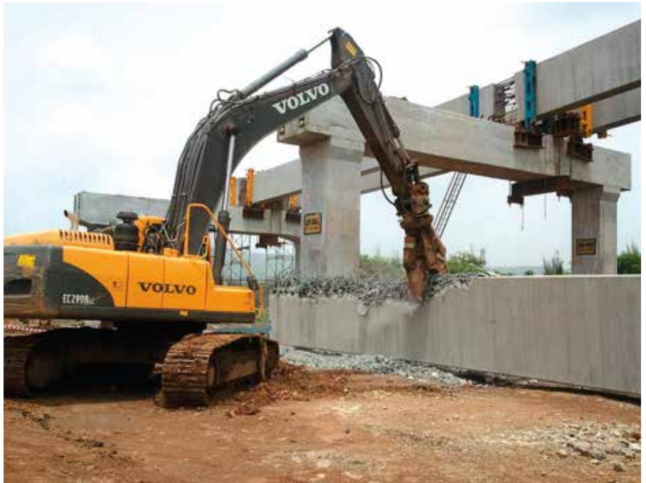
Above and bottom: The Volvo EC290B excavator demolishes the concrete.
