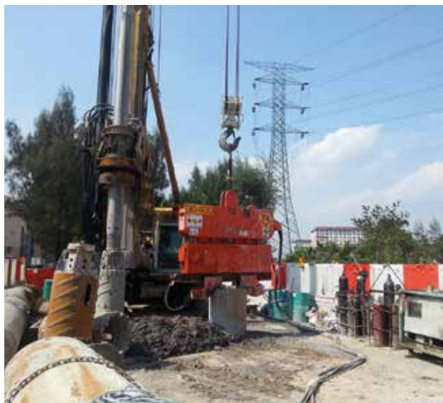
Above and below: The FAV 30-400 hydraulic vibro hammer from Foundation Associates Engineering has an improved eccentric moment of 30 kgm with a greater centrifugal force of 1,069 kN.
