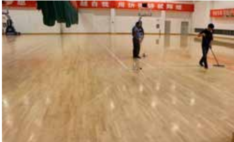
Application of Bona Traffic using a Bona T-Bar.
