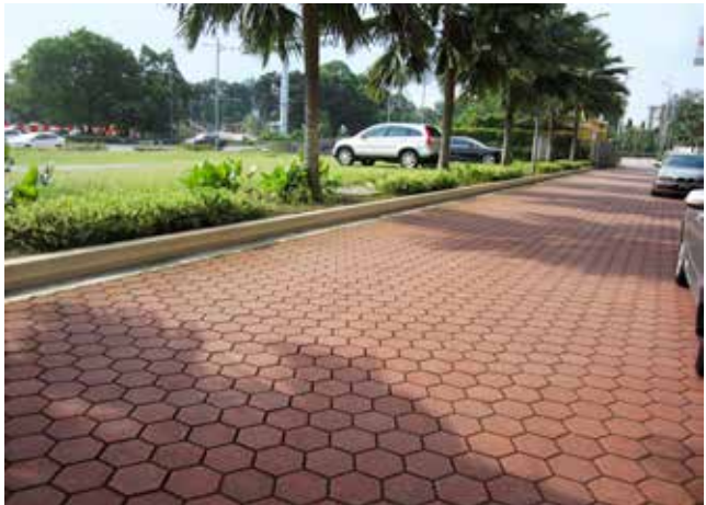
Product: ICP Product profile: Trafika Thickness: 80mm Size: 225mm X 197mm Location: Dataran Glomac, Petaling Jaya, Malaysia
