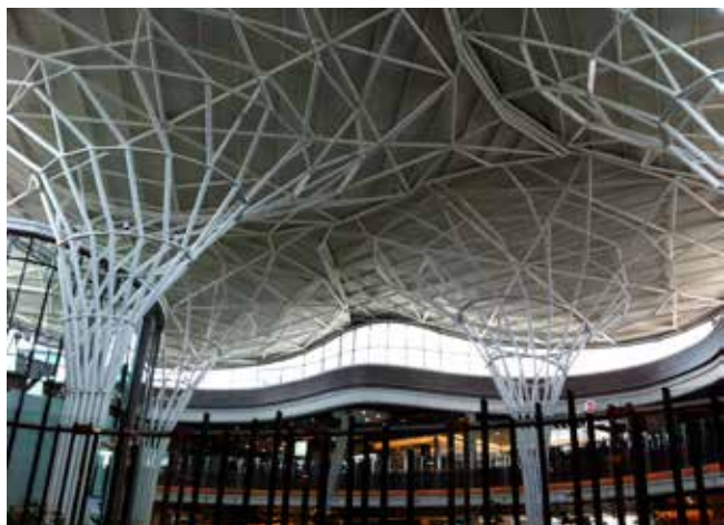
Not only are the white umbrella structures visually appealing, but they also serve the structural purpose in supporting the roof.
