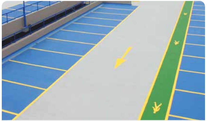
COLOURFUL CAR PARK COATING FOR EXTERNAL APPLICATION
