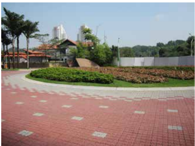
Product: ICP Product profile: Anchorlok Thickness: 80mm Size: 223mm X 111mm Location: South Quay, Bandar Sunway, Selangor, Malaysia
