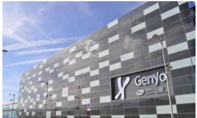
Onyx Solar Photovoltaic Ventilated Facade GENyO Project. Photo: © Onyx Solar Energy S.L.
