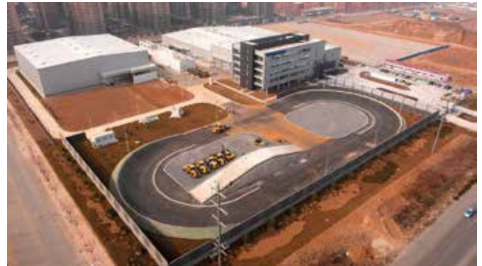
The new Volvo Construction Equipment Jinan Technology Centre will specifically focus on developing products and components for customers in emerging markets.
