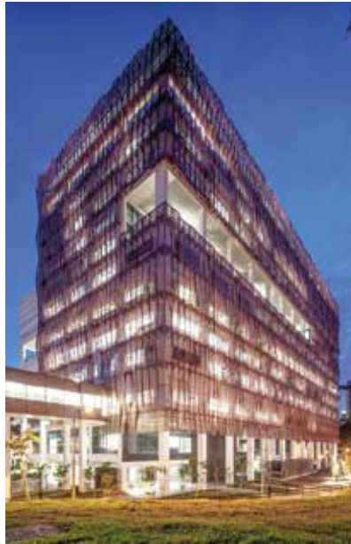
Singapore's National Heart Centre has been completed. Broadway Malyan acted as lead design consultant on the 48,000 sq m, 12-storey development.
