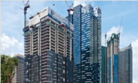
Asia Square Tower, located along Marina View at Marina Bay in Singapore, is a twin-tower mixed-use development. Tower 1 was completed in late 2011, Tower 2 is currently under construction.
