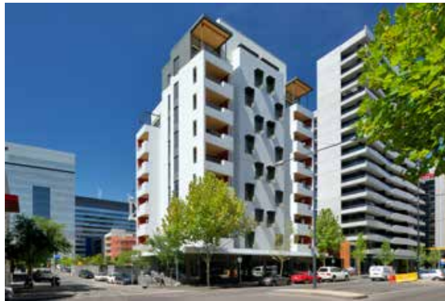
Forté was built using CLT. Designed and built by Lend Lease in Melbourne, Australia, Forté is 10 storeys high and is the tallest residential timber building in the world. Photos: © Lend Lease
