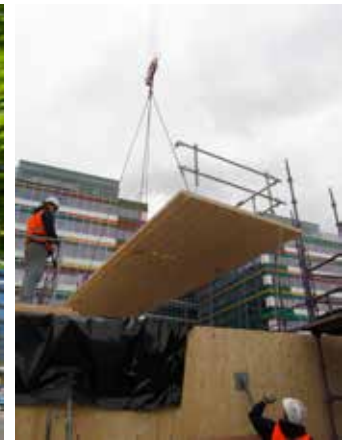
Forté was built using CLT. Designed and built by Lend Lease in Melbourne, Australia, Forté is 10 storeys high and is the tallest residential timber building in the world. Photos: © Lend Lease
