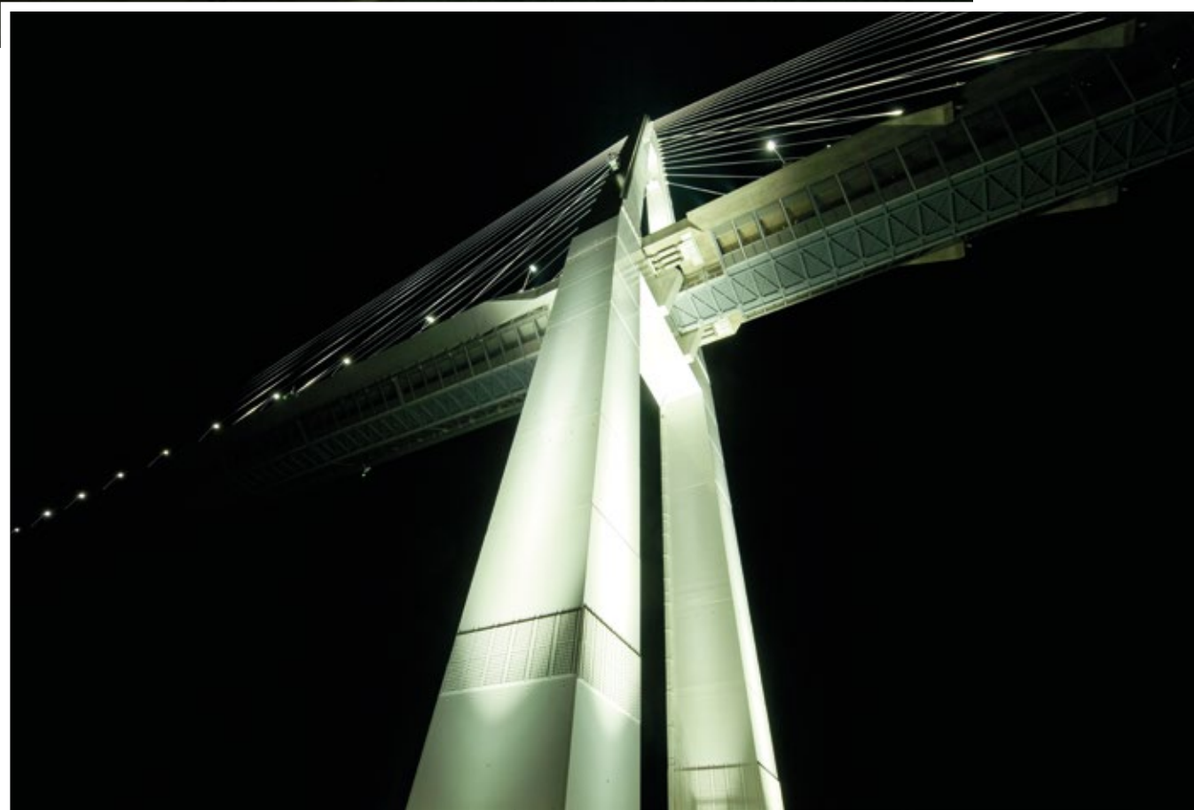
The bridge piers on the approach to Shinminato Bridge are illuminated by LEDioc FLOOD BLITZ 200W LED floodlights.
