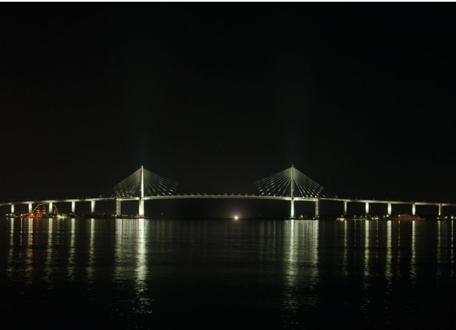
The view from within the city. The elegant form of this now-open, largest cable-stayed bridge on the Sea of Japan coast is illuminated by power conserving and environmentally-friendly LED lighting, producing a very pleasant scene.
