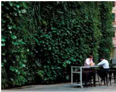
Green wall at 1 Bligh Street.
