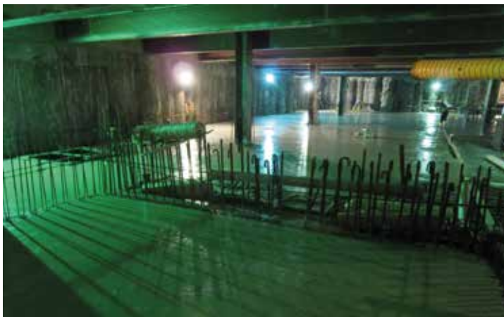
13,401 cubic metres of concrete was used. Photo: © GuocoLand
