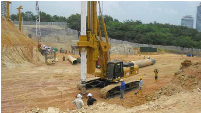
Above: A FAR 250 at a jobsite in Kuala Lumpur constructing bore pile foundation for a commercial building.
