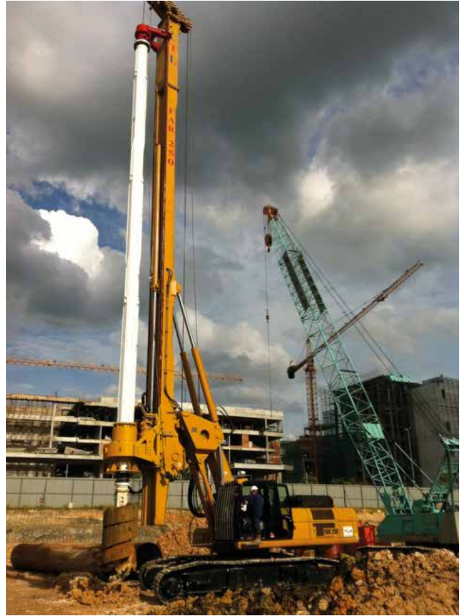
Above: A FAR 250 at a jobsite in Kuala Lumpur constructing bore pile foundation for a commercial building.
