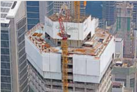
Clean and safe construction at high level with PERI safety screen.
