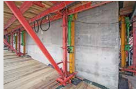
RCS self-climbing technology to eliminate crane usage.
