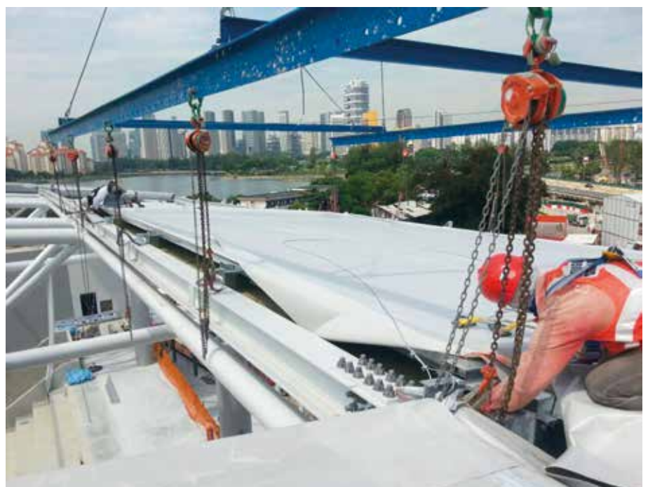
Photos showing application of the Sika® Sarnafil® G476-10. Photos: © SIKA
