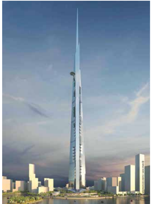
Kingdom Tower. Copyright Adrian Smith + Gordon Gill Architecture
