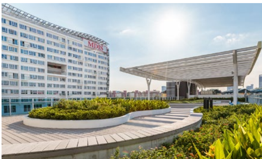
MDIS won the Building and Construction Authority (BCA) Green Mark Gold Plus Award for its 15-storey students’ hostel in 2010 and the revamped six-storey administrative Block A in 2013.
