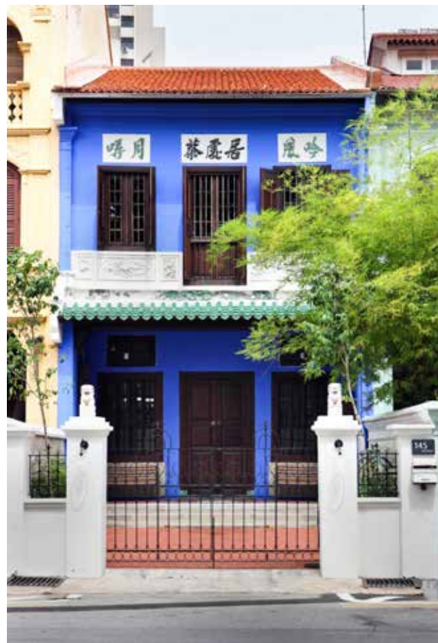
145 Neil Road. Transitional-Style Shophouse restored and repaired in vintage-inspired blue. Photo: © Urban Redevelopment Authority
