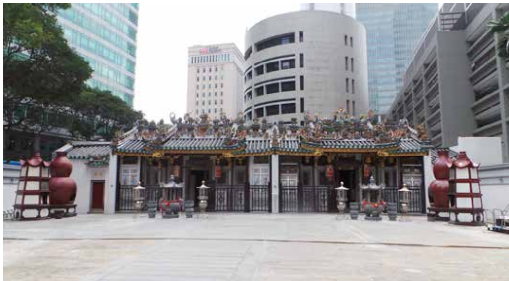
30B Phillip Street (Yueh Hai Ching Temple). Front view of twin temple recovered and revitalised, complete with railings of original design and material. Photo: © Urban Redevelopment Authority
