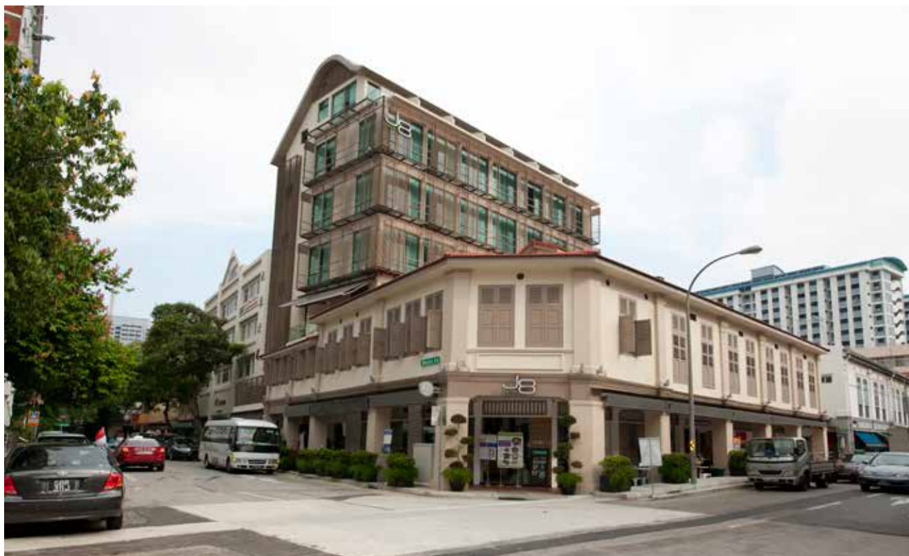
2,4,6,8 and 10 Townshend Road (J8 Hotel). Integration of five Transitional-Style shophouses with new six-storey tower to form a strong streetblock. Photo: © Urban Redevelopment Authority
