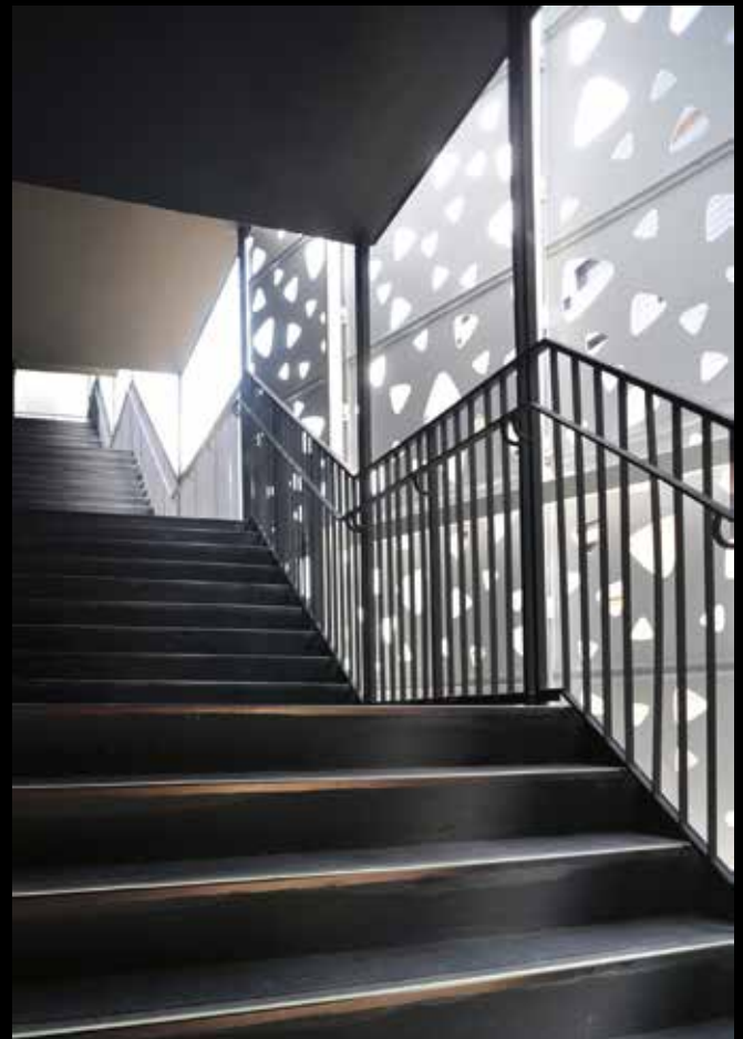
Alum perforated facade from interior.
