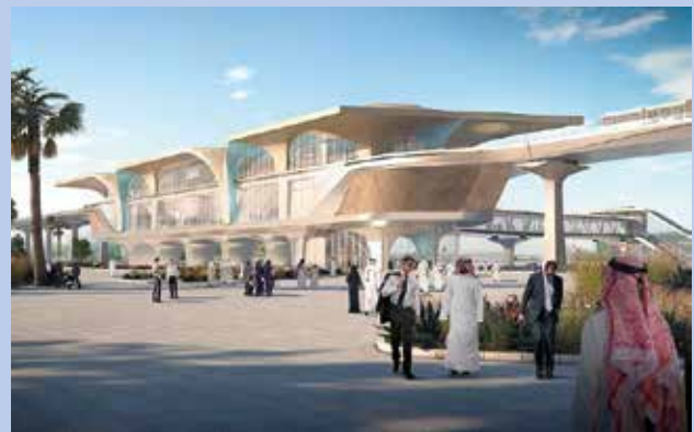
UNStudio designs over 30 stations in Phase One of the Doha Metro Network.
