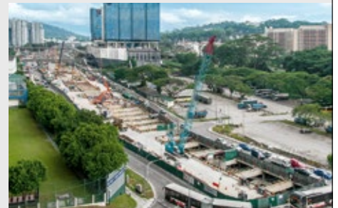
Aerial view of the Bukit Panjang MRT Station.
