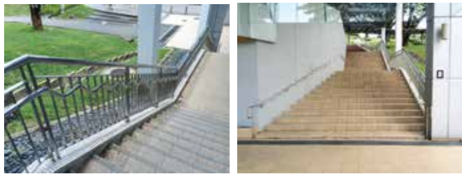
Photos of the J-Wayves installation at the YIH Building in NUS, Singapore.
