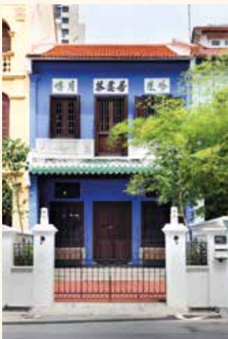
Transitional-Style Shophouse restored and repaired in vintage-inspired blue. Photo: © Urban Redevelopment Authority
