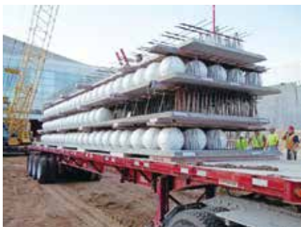
Every part of the BubbleDeck slab can be delivered on site in a precast state, eliminating the need for onsite formwork.
