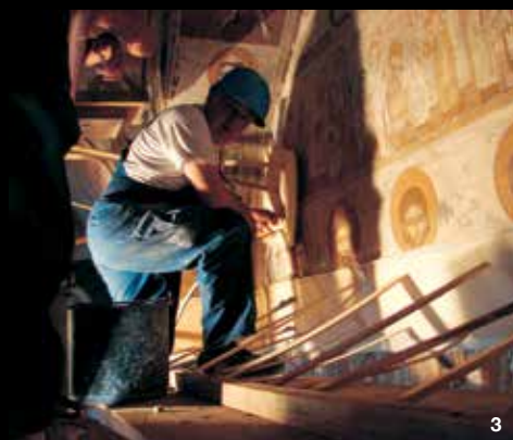
Photos 1, 2 & 3: MAPE-ANTIQUE F21 was used for repair works into the parekklession of Saint Stefan and for the Chapel of Saint John of Rila in some areas surrounding the frescos.
