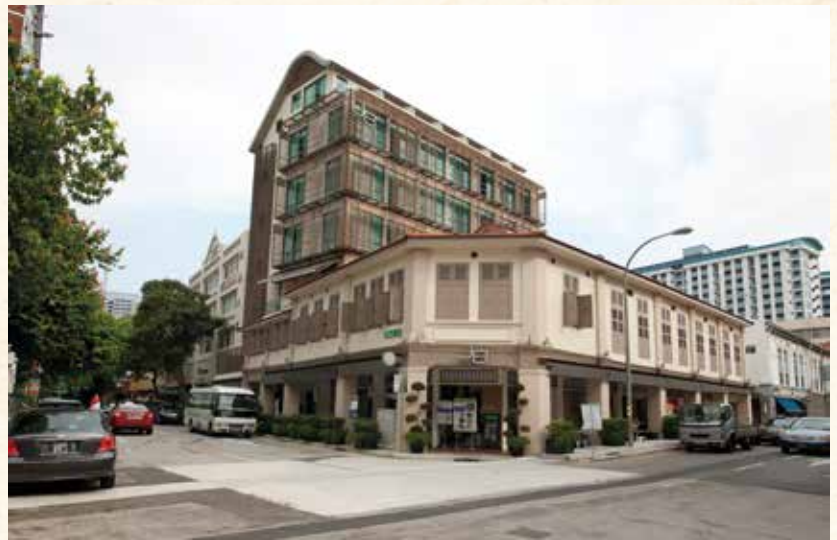
Integration of five Transitional-Style shophouses with new six-storey tower to form a strong streetblock. Photo: © Urban Redevelopment Authority
