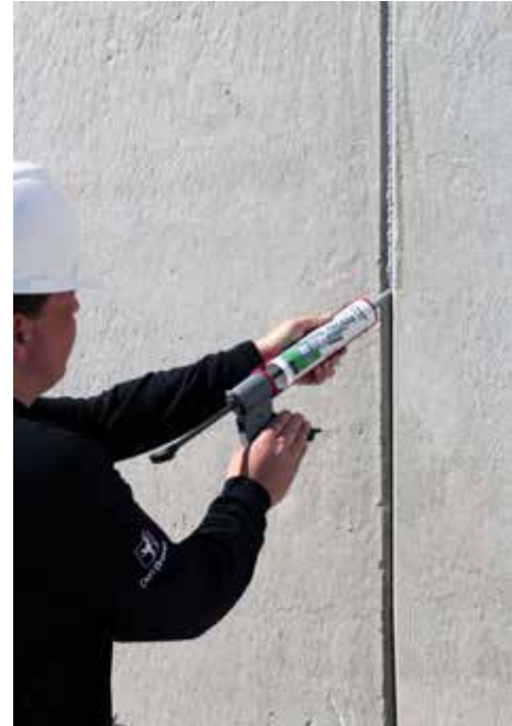
Application of the Zwaluw Hybriseal® Façade.
