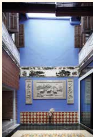
Original courtyard with ornate fish-mould centrepiece, carved relief wall panels and antiquated pigmented cement wall tiles. Photo: © Urban Redevelopment Authority
