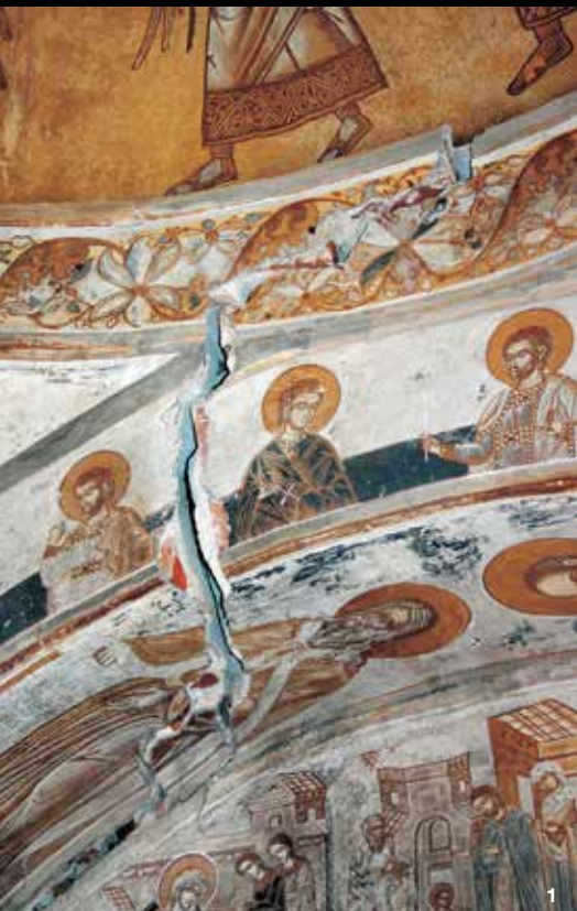
Photos 1, 2 & 3: MAPE-ANTIQUE F21 was used for repair works into the parekklession of Saint Stefan and for the Chapel of Saint John of Rila in some areas surrounding the frescos.
