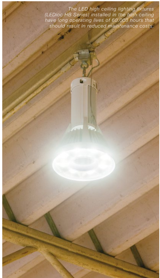
The installed LED high ceiling lighting fixtures (LEDioc HB200)
