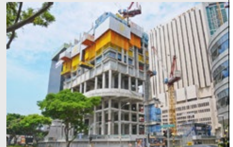
RCS Rail Climbing System and ACS Self-Climbing system minimise the dependency on tower cranes.
