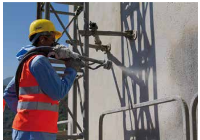
Application of Mapelastix Guard by spray.
