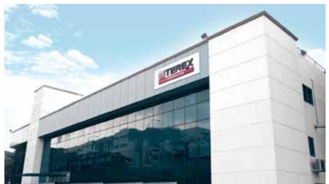
Terex AWP’s new facility includes an expanded workshop and warehouse.
