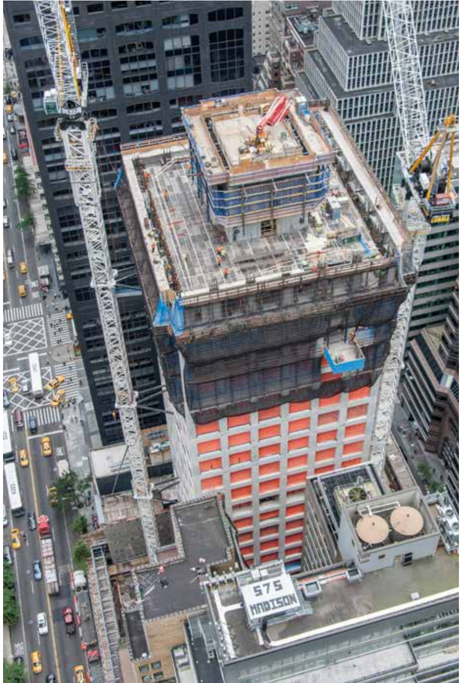
The Xclimb 60 automatic climbing formwork moves an individual steel formwork according to the customer.
