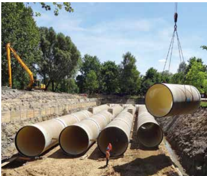
All images: To suit the local requirements at the junction of Ulica Przemysłowa street and Ulica Majakowskiego street, HOBAS designed the underground storage tank with a capacity of 2,410 cu m. The reservoir is made of four 62 m rows of HOBAS GRP pipes DN 3600, shafts, as well as bends with in- and outlet pipes and channels.
