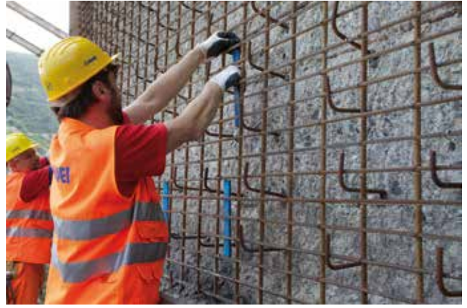
Placing Mapeshield I 30/20 anodes in position.
