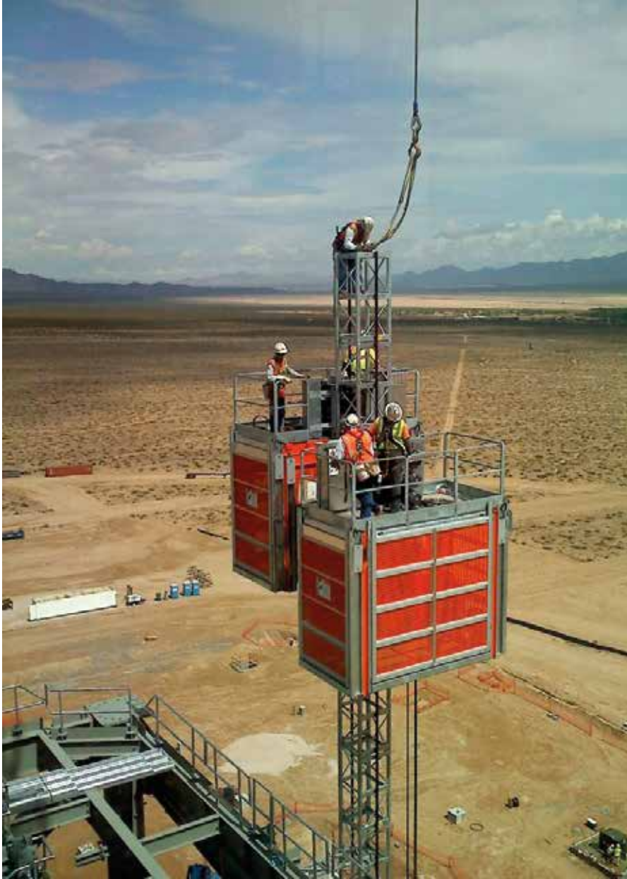
Left and above: Three Alimak Scando 650 passenger and material hoists with dual hoist cars were used during the construction of three 140 m solar receivers/boiler towers at the Ivanpah Solar Power Facility. With a payload of 3,200 kg and a lifting height of 140 m, the hoists provided efficient vertical access for both people and materials on the site.
