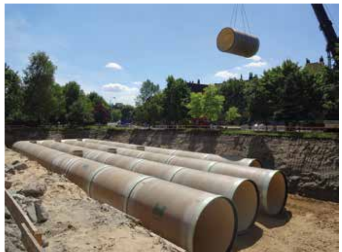
All images: To suit the local requirements at the junction of Ulica Przemysłowa street and Ulica Majakowskiego street, HOBAS designed the underground storage tank with a capacity of 2,410 cu m. The reservoir is made of four 62 m rows of HOBAS GRP pipes DN 3600, shafts, as well as bends with in- and outlet pipes and channels.
