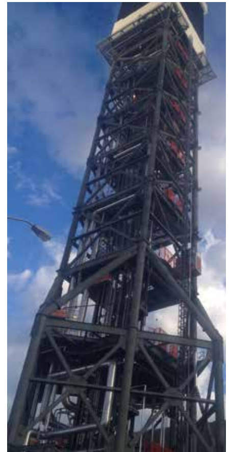
Left and above: Three Alimak Scando 650 passenger and material hoists with dual hoist cars were used during the construction of three 140 m solar receivers/boiler towers at the Ivanpah Solar Power Facility. With a payload of 3,200 kg and a lifting height of 140 m, the hoists provided efficient vertical access for both people and materials on the site.
