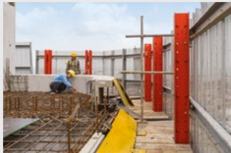
RCS P Climbing Protection Panel and Guardrails serve as a gap-free enclosure and safety barrier against falling.
