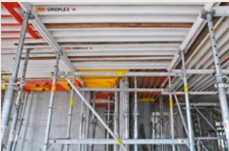
GRIDFLEX Grid Element Slab Formwork and PERI UP Rosett Flex for slab and beam solution.
