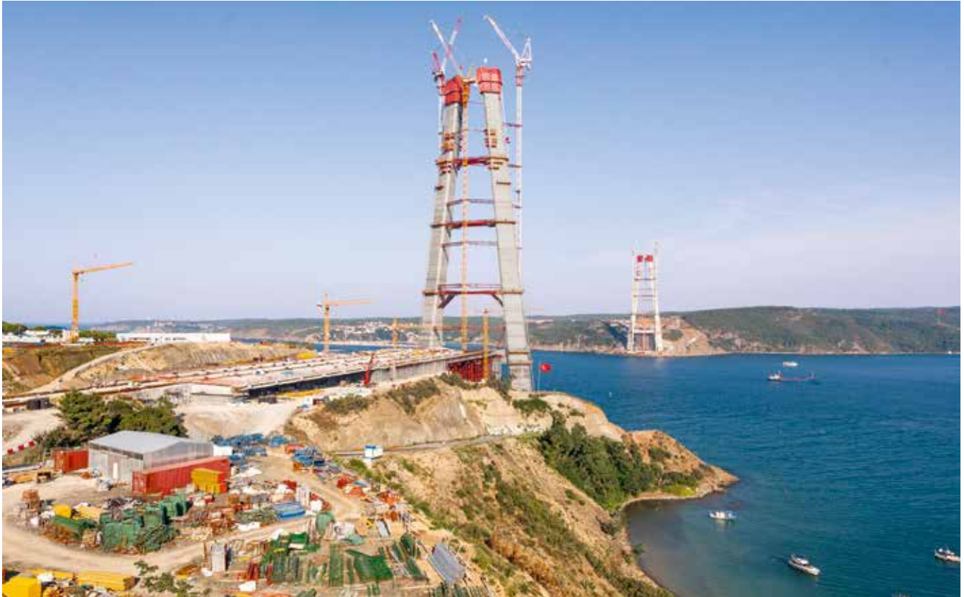
The third Bosphorus Bridge is believed to have the highest concrete bridge piers in the world. It is also said to be the world's largest concrete suspension bridge with railway tracks.
