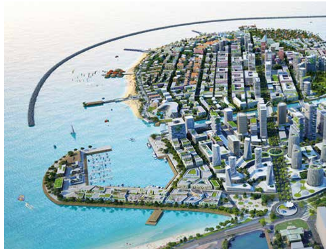
Atkins has been commissioned to assess the opportunity of incorporating a marina into the proposed 2.5 sq km mixed use Colombo Port City development in Sri Lanka.
