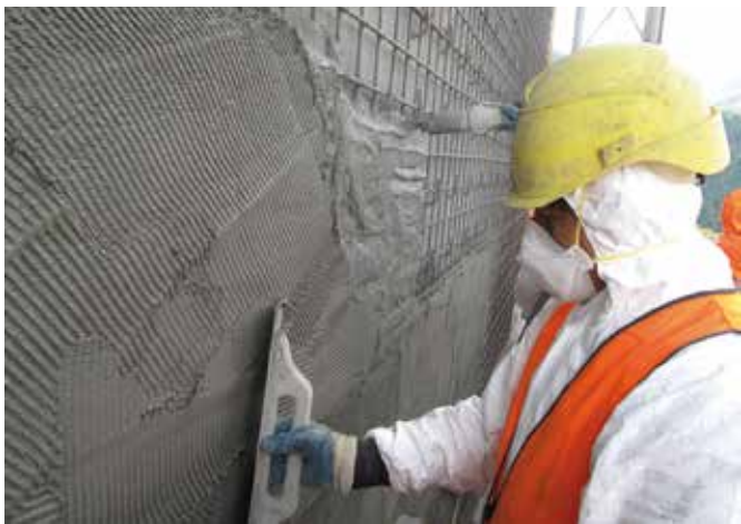
Application and roughening of the first layer of Mapegrout Easy Flow.
