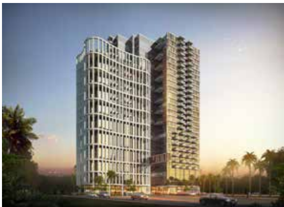
Ampang 201, Kuala Lumpur, Malaysia, designed by ThomsonAdsett.
