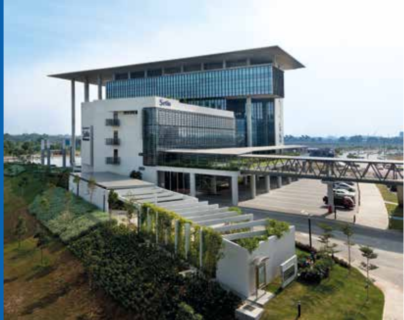
Formal entrance to the Setia Corporate Headquarters.
