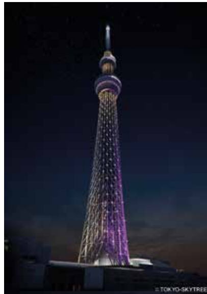
Tokyo Skytree illuminated with 1,995 LED lighting fixtures from Panasonic. Photo: © Tokyo Skytree
