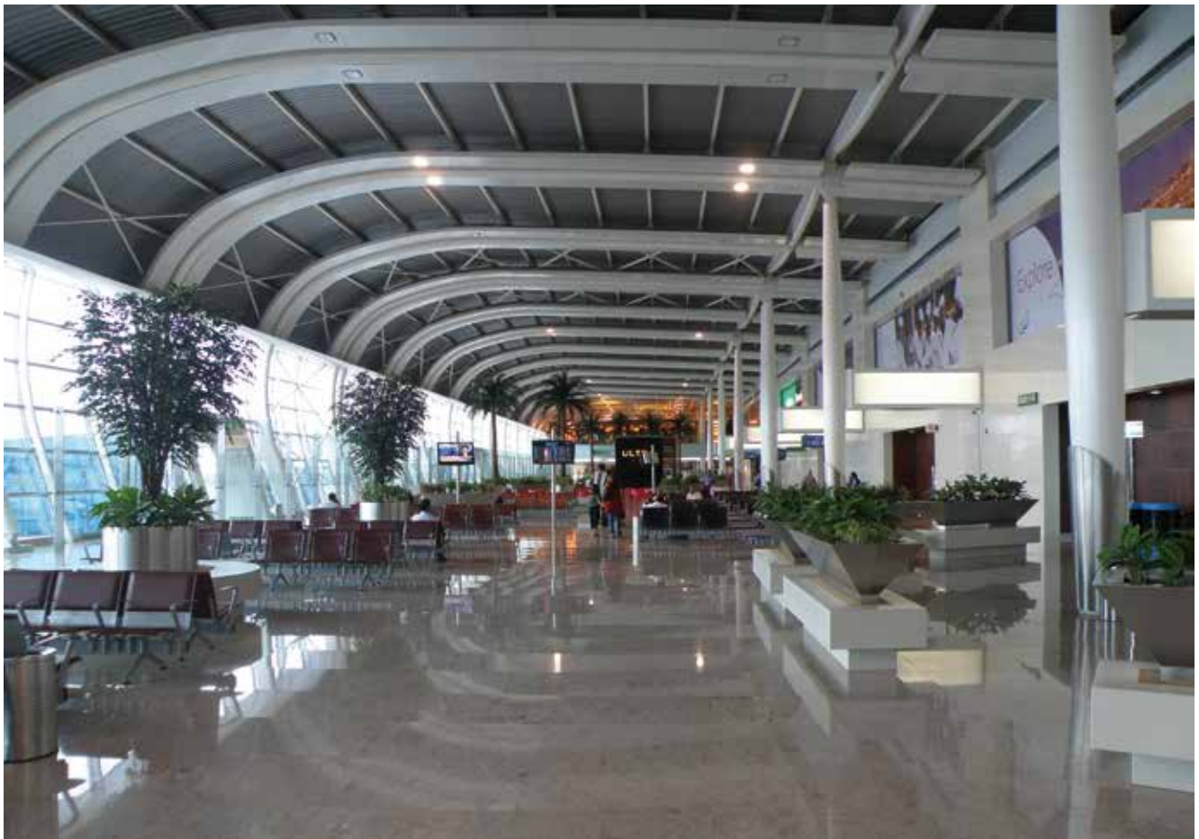
Mumbai airport upon completion of work.
