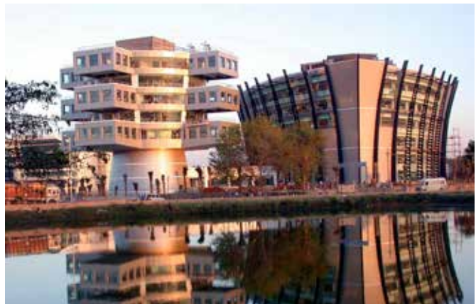
IFLEX Software building in Bangalore, India.
