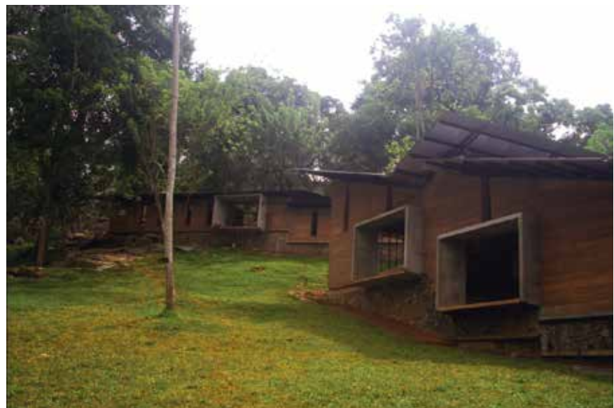
The library is under construction now.
