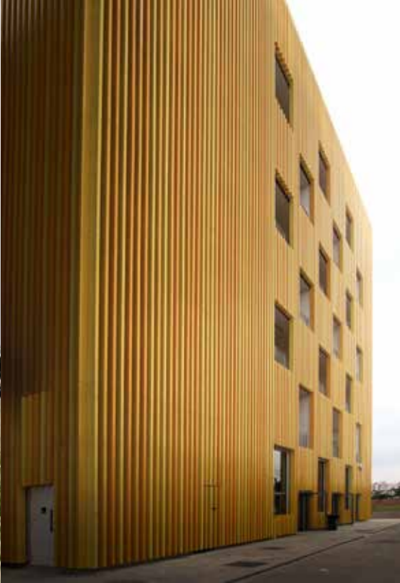
Facade treatment for worker dorms is designed to allow for privacy as well as allow ample natural ventilation into the spaces.
