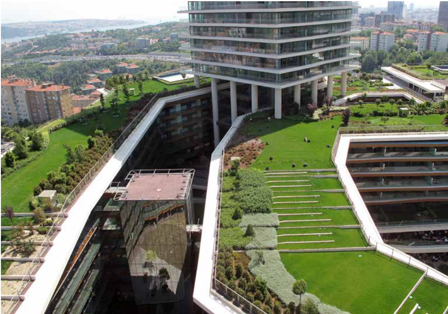
Green Roof shells of Zorlu Center. Photo Copyright: Onduline Avrasya A.S.
