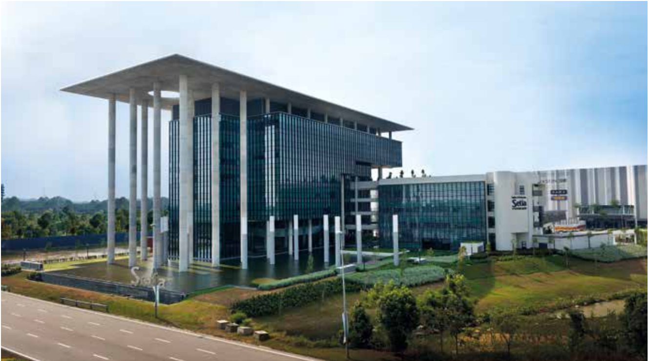
Nine columns rising 40 metres lift the building like a parasol into the sky.
