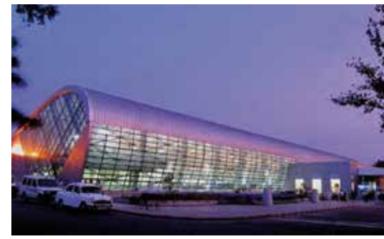
Mumbai airport after completion.
