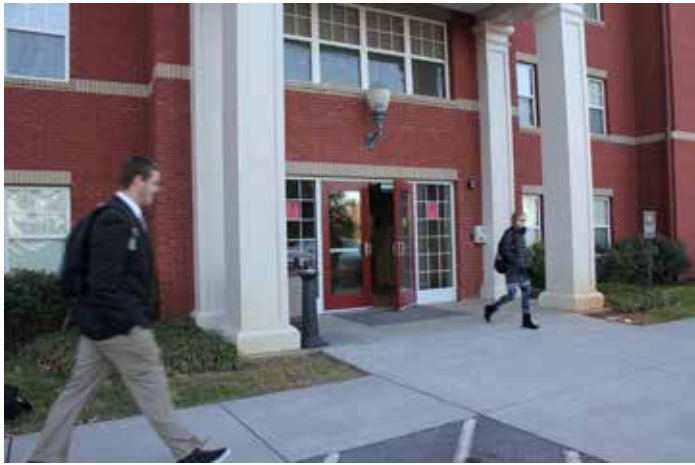
Gibson Hall, Maryville College's newest dormitory, is more secure with System Galaxy.
