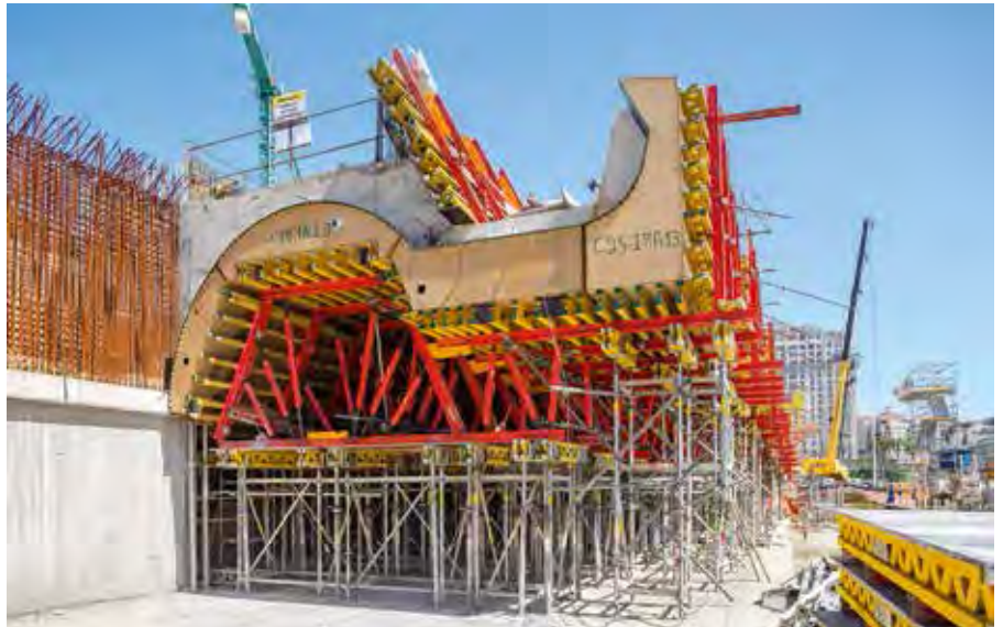
Above: Supported by Peri Up shoring and working scaffolds, as well as a Variokit raised formwork units, the customised elements were assembled on site to form a complete 3D formwork construction.
