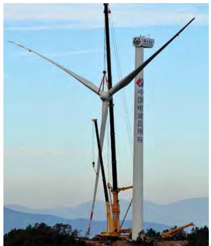
Left and above: The XCA5000 erects a 2 MW wind turbine.
