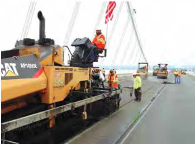
The epoxy offered significant benefits, including durability and traction, but was very difficult to work with.
