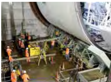
Tunnel Boring Machine Launching
