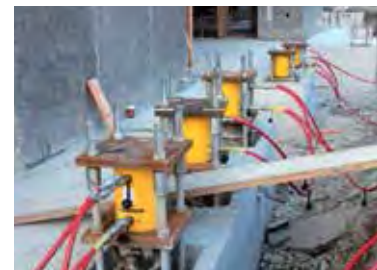
Lifting unstable structure for foundation repair
