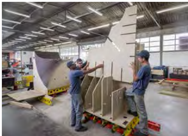
Above: Supported by Peri Up shoring and working scaffolds, as well as a Variokit raised formwork units, the customised elements were assembled on site to form a complete 3D formwork construction.
