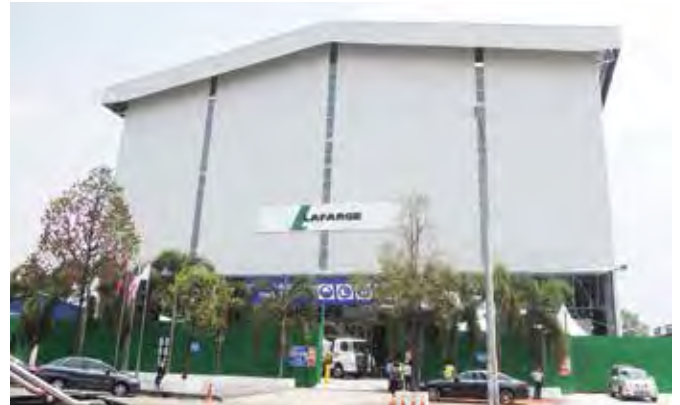
Left and above: Lafarge Malaysia has taken delivery of a ready-mixed concrete batching plant from IPS-Eurotec. The plant is fully enclosed, featuring reduced noise and low air pollution level.
