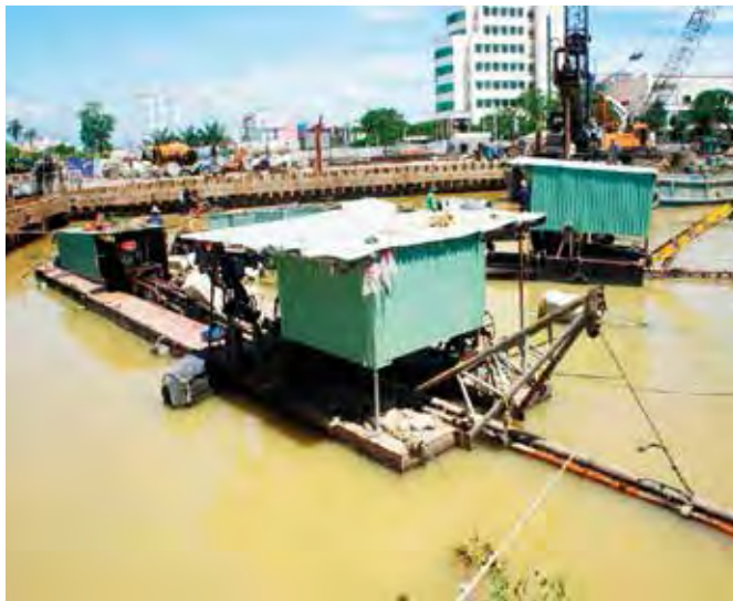
P3 concrete pile application.
