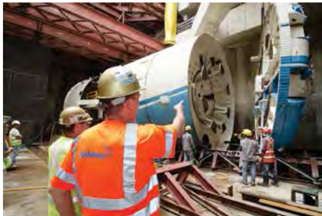
Above: Assembly of GS Engineering’s C925 EPB took place in a cradle that had to be jacked into place for the tunnel alignment.
