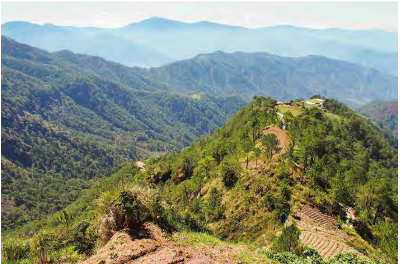
Top and above: When fully operational, the Sabangan hydropower plant will supply the Mountain Province with 14 MW of clean and renewable energy.
