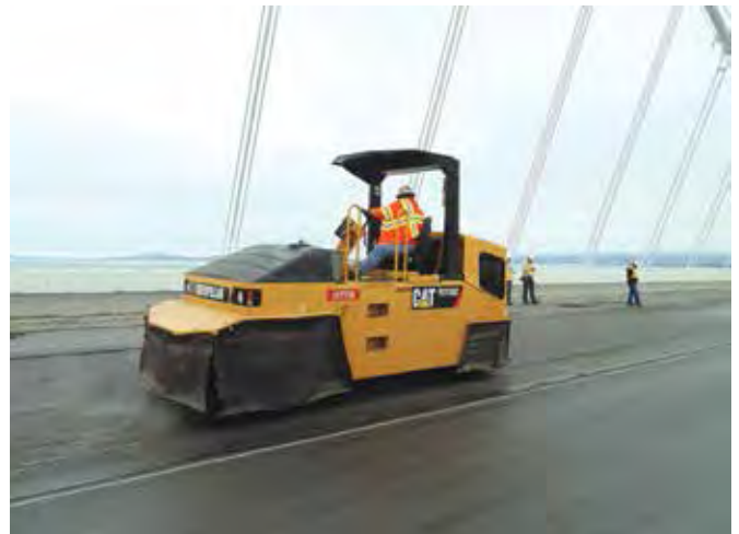
Compaction and rolling patterns were closely monitored given the challenging material.
