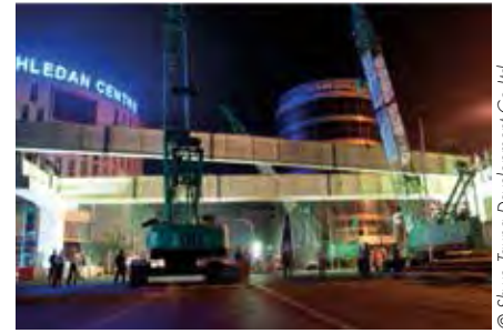
Top and above: Erection of steel girders.
