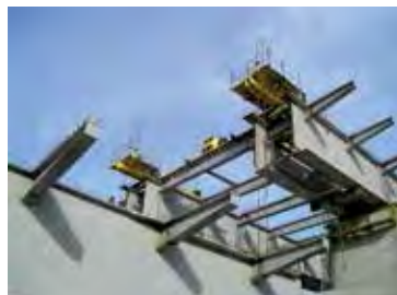
Lifting a bridge deck
