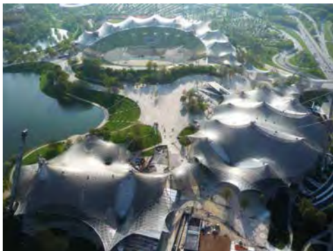
Roofing for main sports facilities in the Munich Olympic Park for the 1972 Summer Olympics, 1968–1972, Munich, Germany. Photo: © Christine Kanstinger
