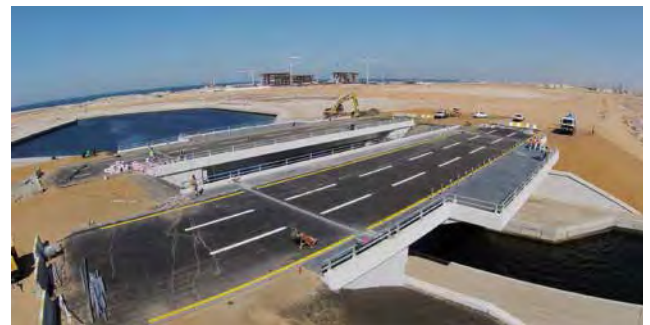
Al Zohra infrastructure development in progress.
