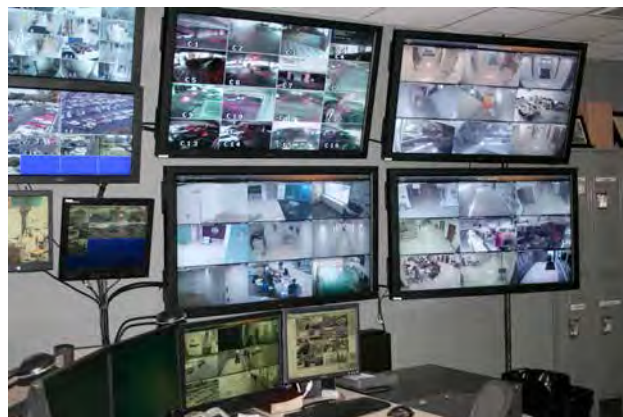
Missouri State's Public Safety Dispatch Center houses a video wall, controlled by OnSSI's Ocularis Video Management Software. The video wall displays feeds from the more than 500 constant and motion-activated cameras located throughout the 225-acre campus.
