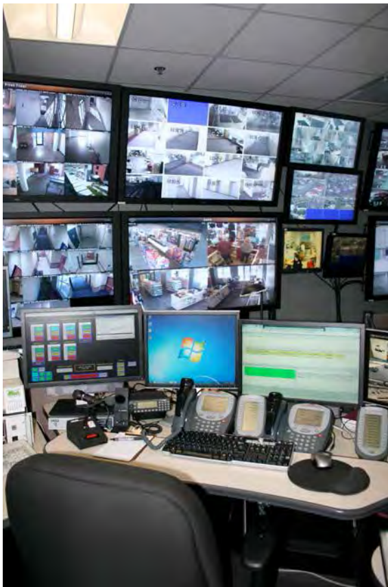
Missouri State's Public Safety Dispatch Center houses a video wall, controlled by OnSSI's Ocularis Video Management Software. The video wall displays feeds from the more than 500 constant and motion-activated cameras located throughout the 225-acre campus.
