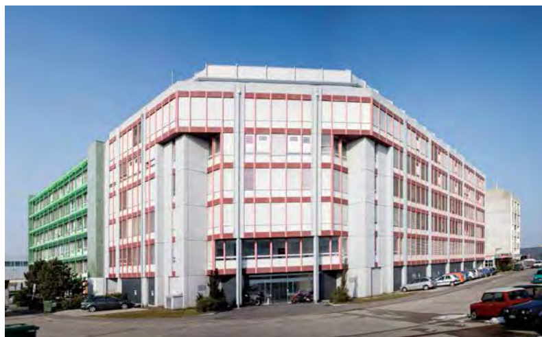
Safe Host, a Swiss data center, uses a Sinorix gas extinguishing system.
