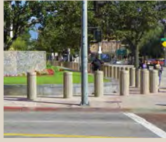
U.S. FEDERAL COURTHOUSE- LOS ANGELES Delta Fixed Bollards
