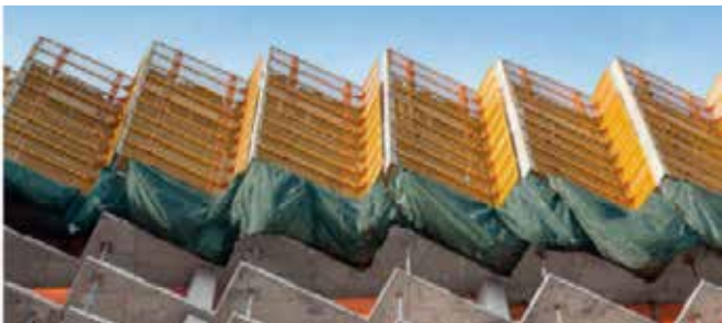
The LPS screen is available in two versions, either as a perimeter protection system or with a working platform that provides access to the bulkhead formwork.
