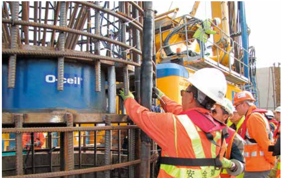
Above: Final check on O-cell assembly before lowering into bored hole.
