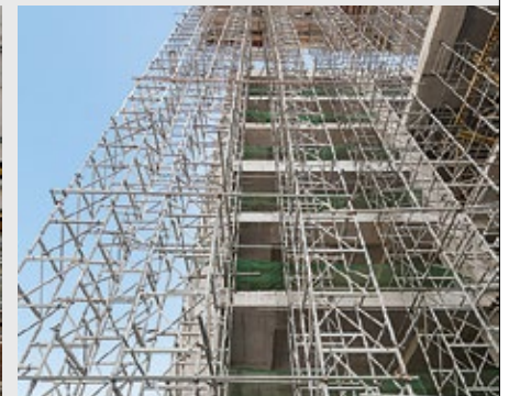
ST 100 Stacking Towers as high shoring system to support beam and slab.
