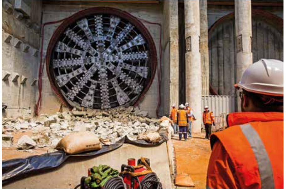
Above: At the end of September 2014, the cutting wheel of TBM Alice broke through the target shaft wall for the first time.
