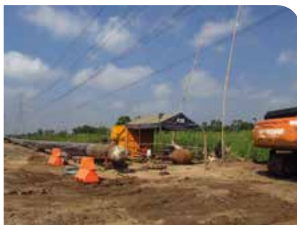
Left and right: The 28-in pipe was being prepared for installation at the exit pit.
