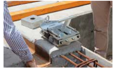
Left: Pulling power for the skidding operation was provided by pairs of RR series double-acting Enerpac RR 3014 cylinders with 368 mm strokes.
