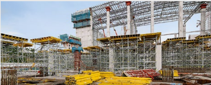
PERI UP Rosett Shoring System for slab and beam support.
