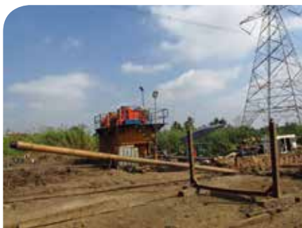
Left and right: The 28-in pipe was being prepared for installation at the exit pit.
