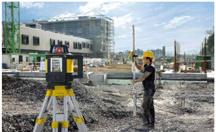
Above: The Rugby 870 laser is suitable for applications such as levelling, concrete pours and drainage in single axis.
