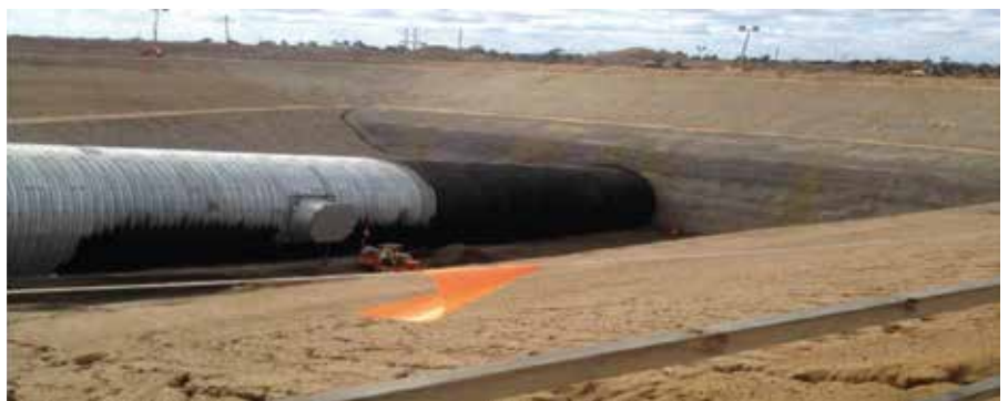
All images: TBM technology is being deployed to build two drifts at the Grosvernor coal mine. Here, Mapei admixtures have also been used for backfill grout.
