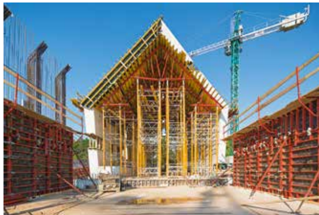
Below: The tilting walls are formed using Peri's Trio large sized elements – supported by diagonal bracing.
