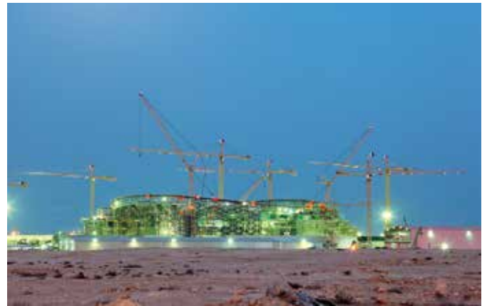
Construction of a new stadium near Lusail, Qatar.
