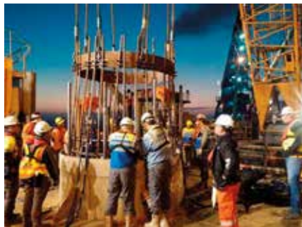
Above: Final check on O-cell assembly before lowering into bored hole.
