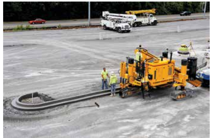
The GT-3600 curb and gutter machine.
