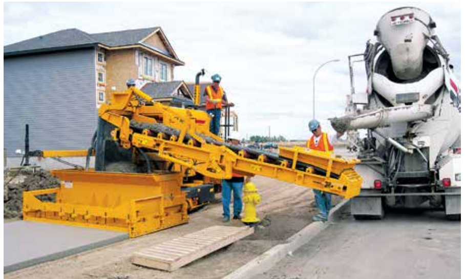
The conveyor on the GT-3200 sidewalk paver can be hydraulically raised without being folded to avoid smaller obstacles such as fire hydrants and utility boxes.
