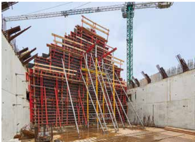
Below: The tilting walls are formed using Peri's Trio large sized elements – supported by diagonal bracing.
