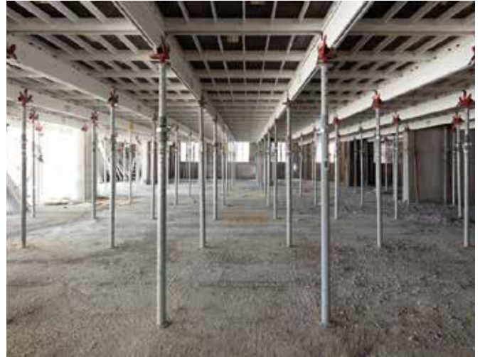
Pilosio's Slabform system is designed for concrete slabs with thicknesses of up to 100 cm.
