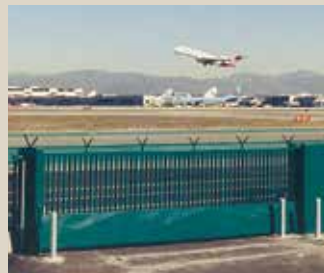
LOS ANGELES INTL. AIRPORT Delta SC3000 Sliding Gate
