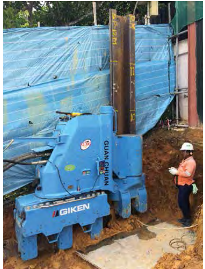
The Zero Clearance Method employs a specially designed press-in machine (zero piler) and zero sheet piles (NS-SP-J) to press-in piles with zero 'dead space' between the piles and the adjacent structure.
