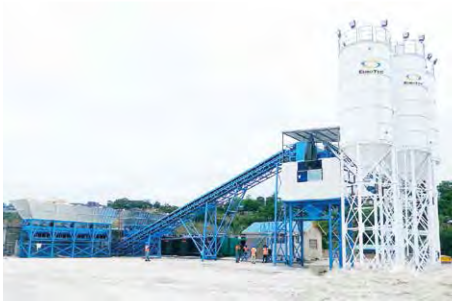
Eurotec's concrete batching plant at the Mombasa Port Development Project site.
