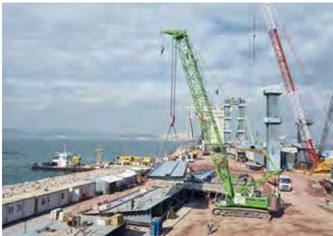
Above and below: A Sennebogen 5500 crawler crane performs lifting tasks at the Izmit Bay Bridge.
