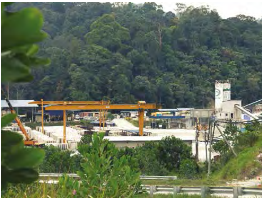
Top: The first of three Robbins TBMs excavated 11.2 km, and broke through in March 2013.
