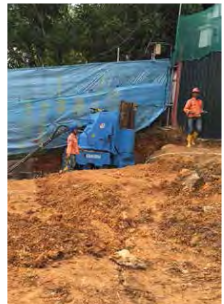
The press-in machine grips securely onto the completed piles, so there is no risk of overturning.
