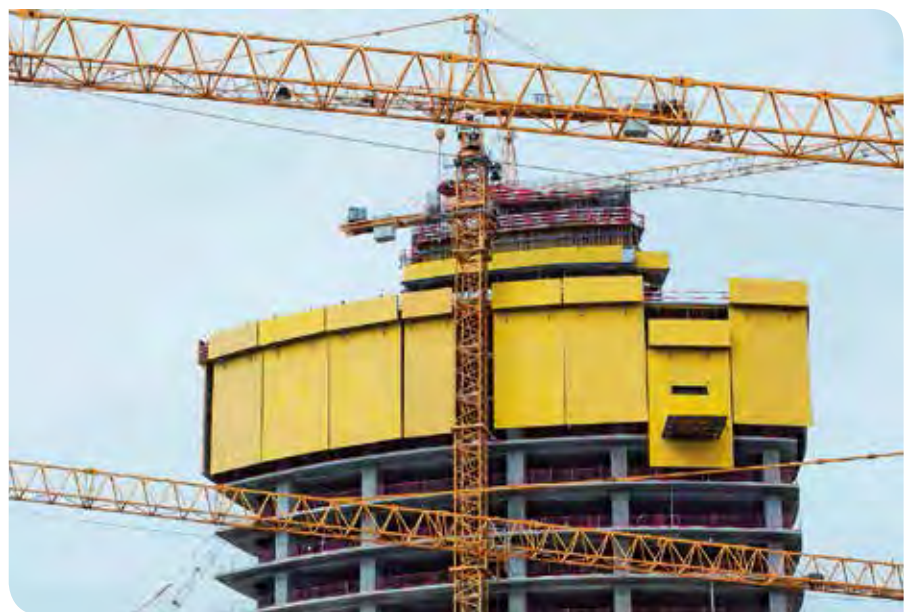
The TLS table lifting system is a safe method for repositioning floor formwork without a crane and an ideal add-on to the Xclimb 60 protection screen.
