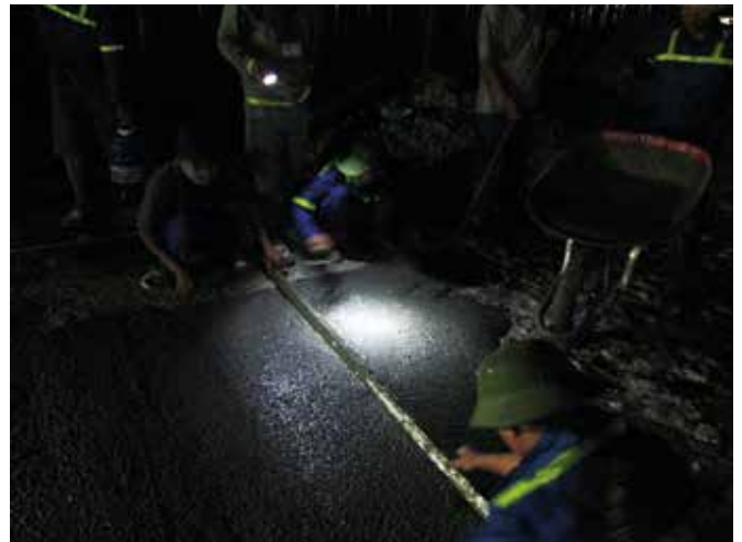
Above and below: In the first phase of concrete repair work, the surface of the damaged existing concrete slabs was removed up to 5 cm in depth, before applying a mixture of gravels and Mapefill SP high-flow shrinkage-compensated cementitious grout.
