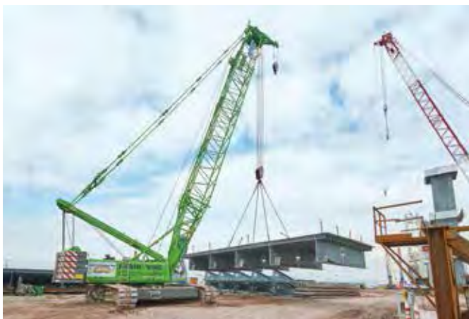
Above and below: A Sennebogen 5500 crawler crane performs lifting tasks at the Izmit Bay Bridge.
