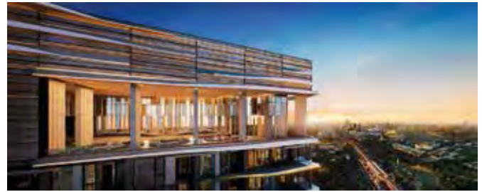
The LINE Jatujak-Mochit condominium project is scheduled for completion in November 2017.
