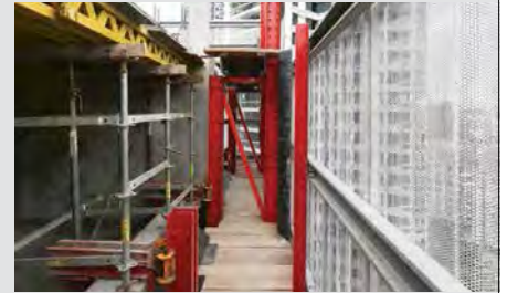
The RCS rail climbing safety screen provides safe and efficient working conditions for high-rise structures
