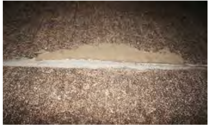
Above and below: In the second phase of concrete repair work, Mapegrout SV quick-setting and hardening, compensated-shrinkage hi-flow mortar was used for cracks and damages along the flexible joints (above) and on the existing concrete slabs.
