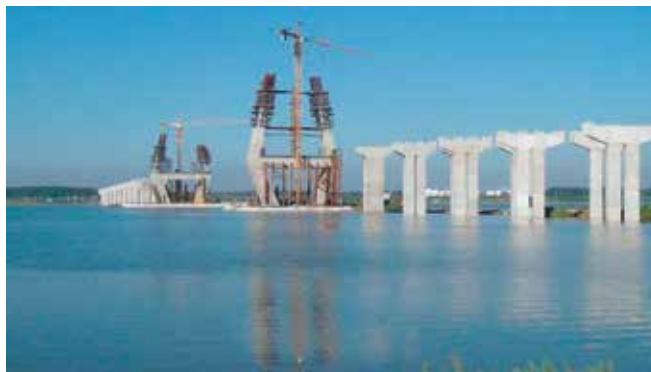
Above and left: A new cable-stayed prestressed concrete bridge in Shandong province, China, was recently opened to traffic. Construction of this massive bridge spanning the Yi River was said to be a huge challenge.
