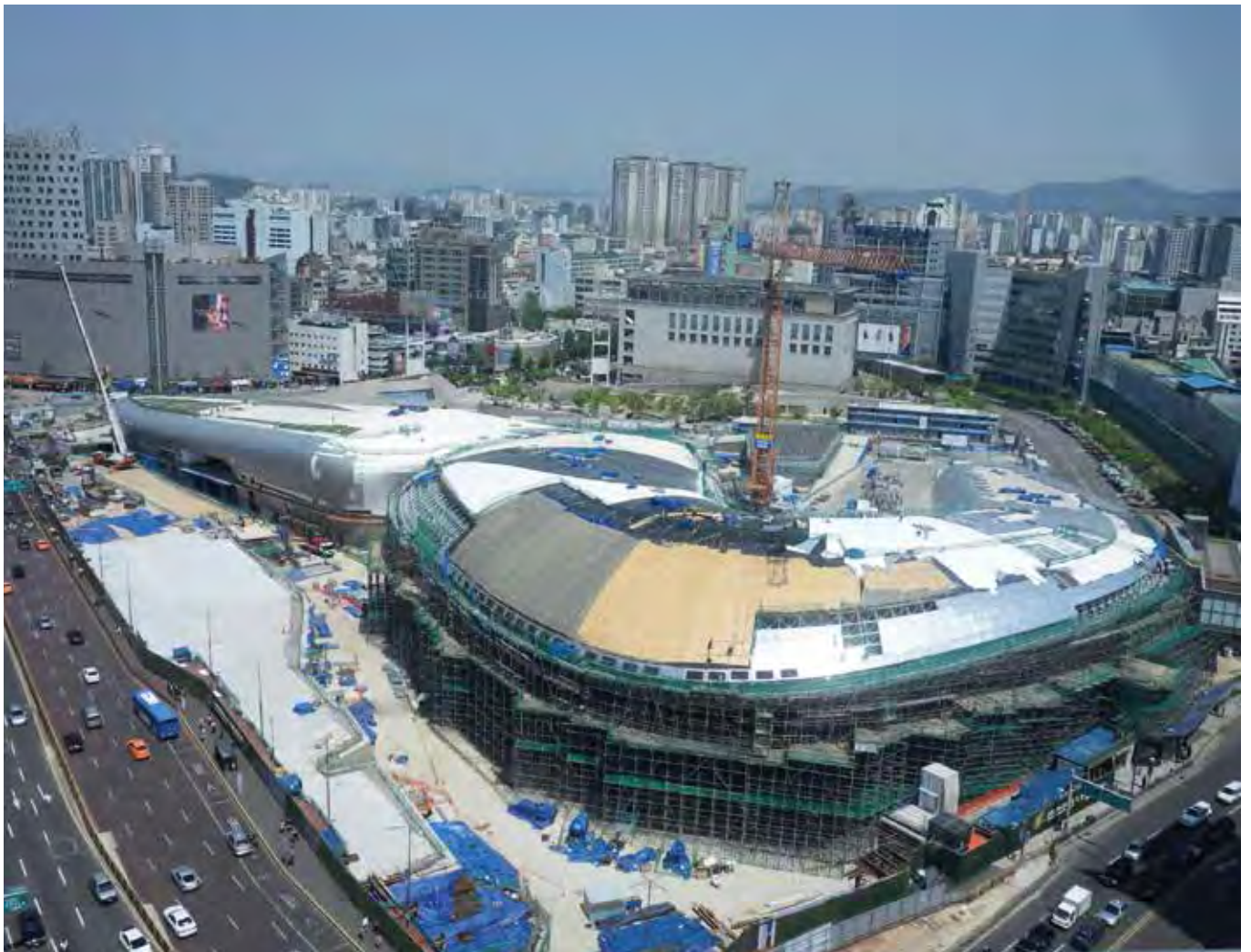
Above and below: The building's exterior is made up of more than 45,000 panels, with no two panels having the same shape.
