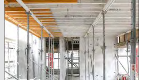
GRIDFLEX Grid Element Slab Formwork and PERI UP Rosett Flex for the casting of beams and slabs
