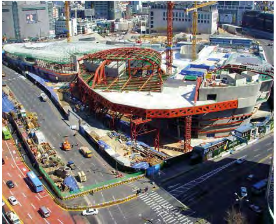
Above and below: The building's exterior is made up of more than 45,000 panels, with no two panels having the same shape.
