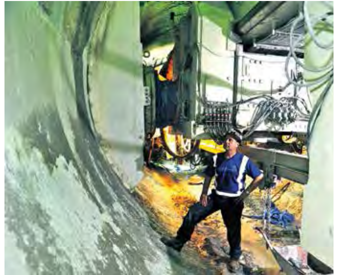
Andy Birch, Robbins Adit 4 site manager, surveys the excavated tunnel.
