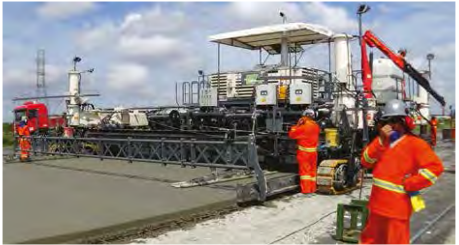
The super smoother moves back and forth and from side to side.
