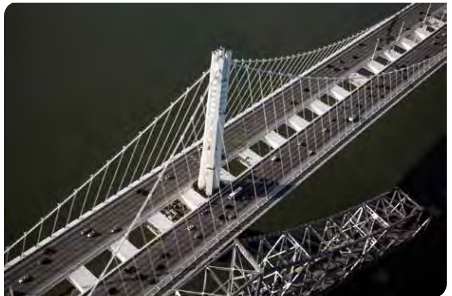
The SAS is believed to be the world's first suspension bridge with no connection between the deck and tower. Instead, the box girders 'float' at the tower, with the suspenders providing the only connection between the box girders and tower.
