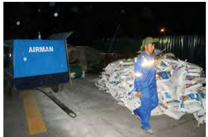
Mapefill SP at the worksite.
