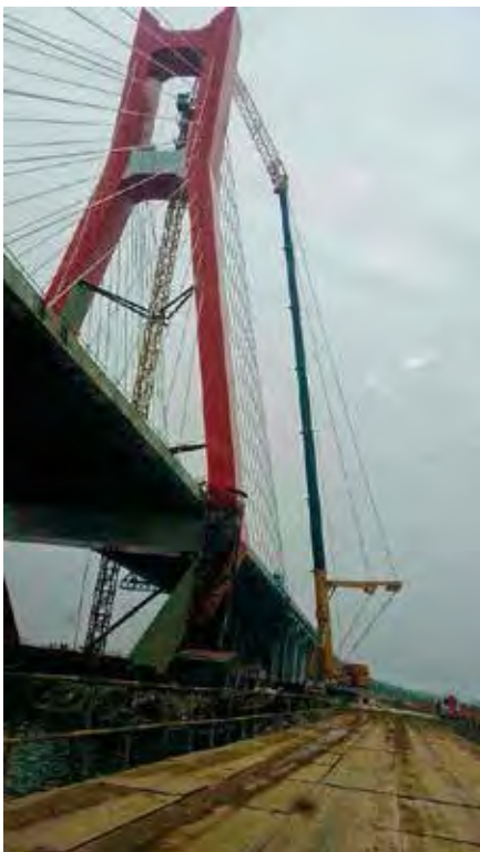
Above, left and right: To cope with the challenge, the construction team employed an XCMG QAY500 all-terrain crane with a maximum lifting capacity of 500 t.
