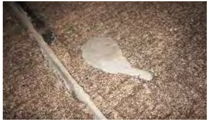
Above and below: In the second phase of concrete repair work, Mapegrout SV quick-setting and hardening, compensated-shrinkage hi-flow mortar was used for cracks and damages along the flexible joints (above) and on the existing concrete slabs.
