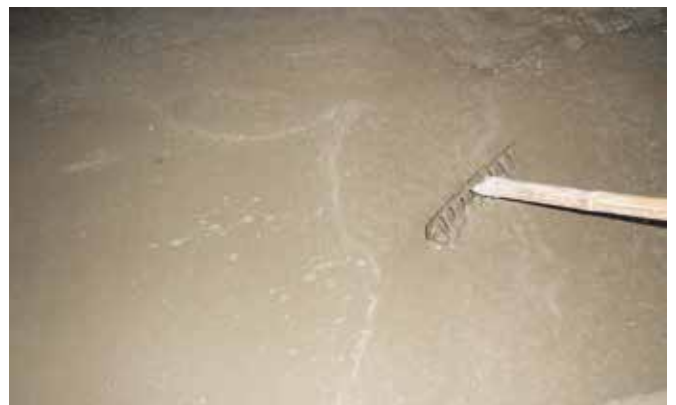
Above and below: In the first phase of concrete repair work, the surface of the damaged existing concrete slabs was removed up to 5 cm in depth, before applying a mixture of gravels and Mapefill SP high-flow shrinkage-compensated cementitious grout.
