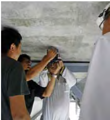
Pull-off test to check substrate strength.
