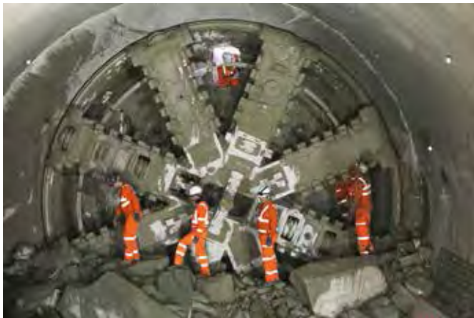
The TBM Elizabeth achieved a breakthrough on 10 May 2015.
