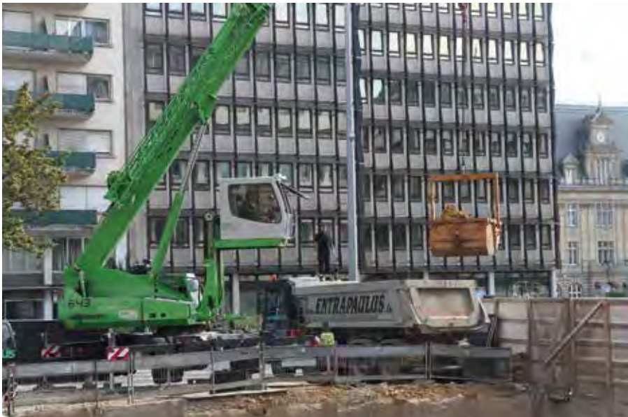
A Sennebogen 643 telescopic crane lifts some excavated soil to the surface and loads it onto the truck. The crane is currently helping to construct the foundation of an eight-storey office building in Luxembourg.
