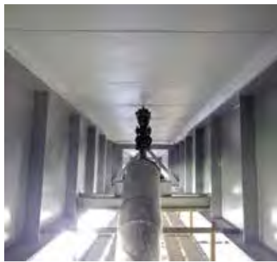
Completion of Colorite 880 W application.
