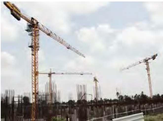
Potain cranes being used on the DSK Dream City development in Pune, India.
