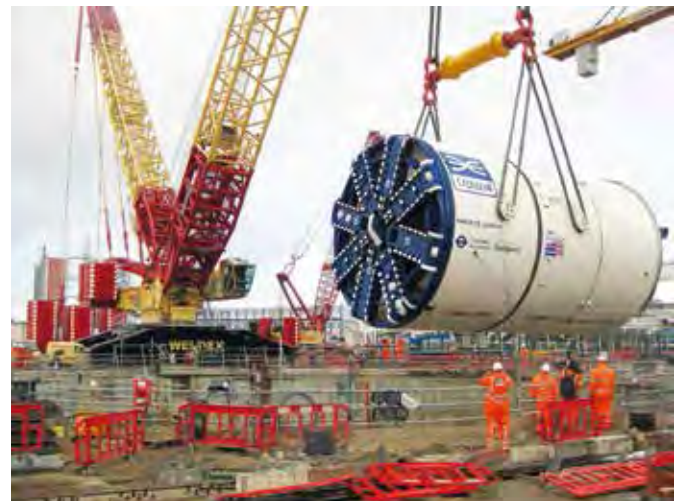
The TBM Victoria being lifted into the Limmo Peninsula launch shaft. It then bored its way from east to west through central London. Over a distance of 8.2 km the TBM drove beneath Soho, Hyde Park and several housing estates.
