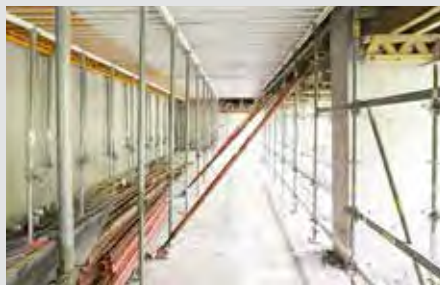
Panels of Grid Element Slab Formwork system GRIDFLEX are supported by PEP Props & PERI UP Rosett.
