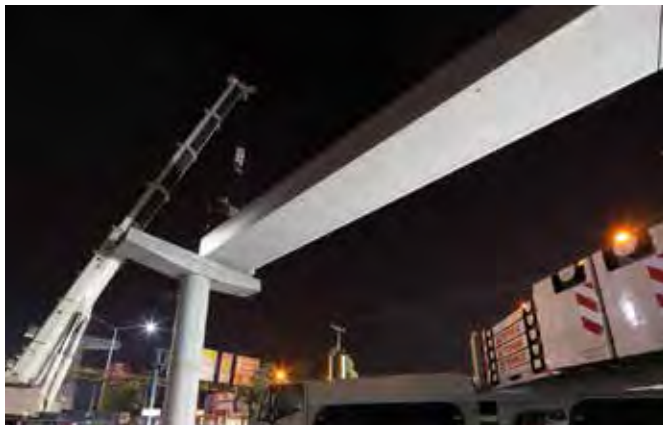
Top and above: Terex AC 350/6 and AC 500-2 all terrain cranes being used on the Metrorrey Line 3 project.
