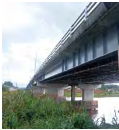
Top and above: Batu Kawa Bridge has recently been upgraded.
