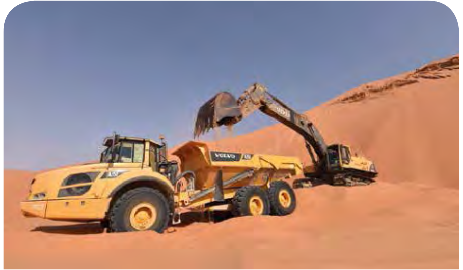
Volvo machines used on the project included a range of articulated haulers, excavators and motor graders.
