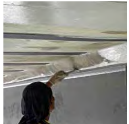
Application of Colorite 880 W to provide protective and decorative coating.
