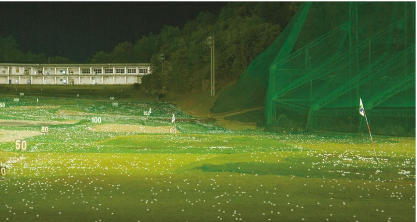
Looking at the north tee-off area from the 100-yard mark. The high-output LED floodlights (LEDioc FLOOD DUELL 1000W) installed on the roof have a good balance of both wide and narrow light distribution and light the fairway in symmetrical light.
