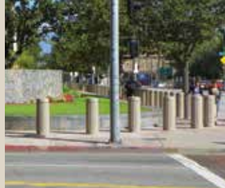
U.S. FEDERAL COURTHOUSE- LOS ANGELES Delta Fixed Bollards
