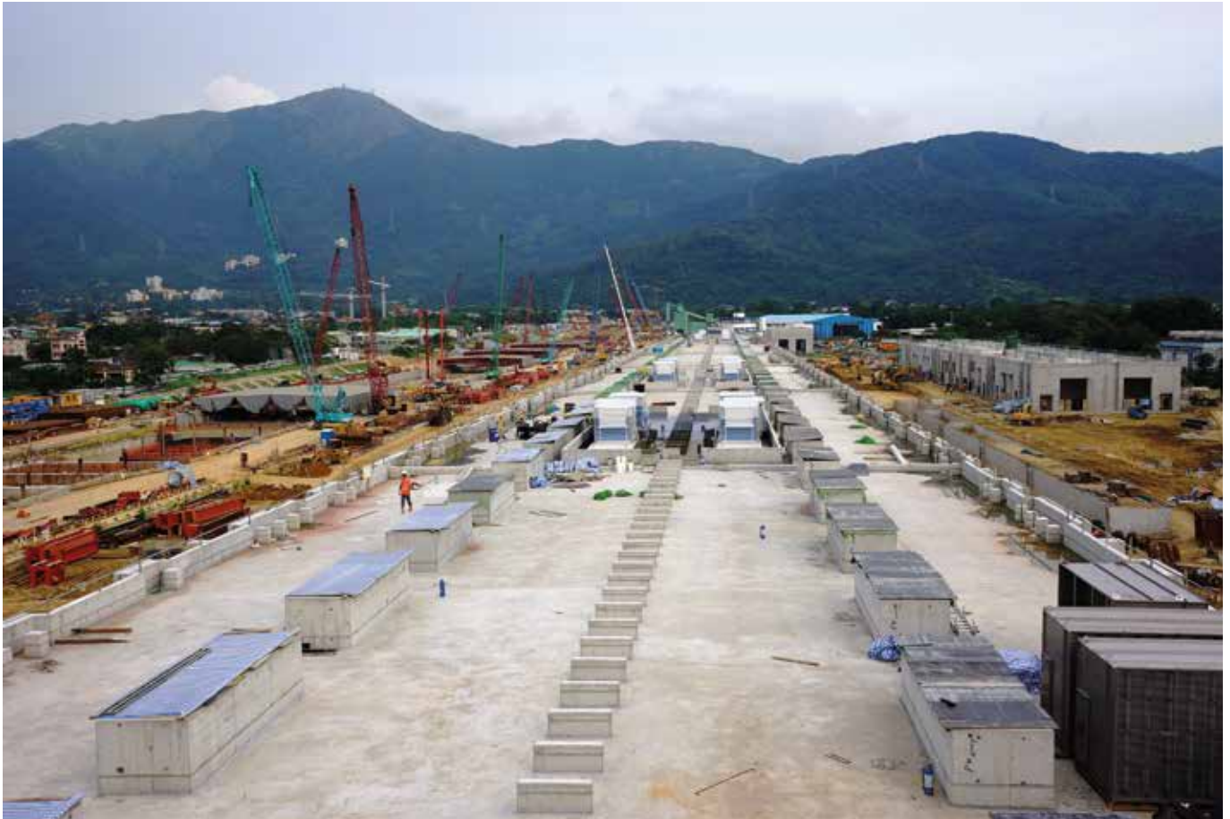
The rooftop of a maintenance and plant building.
