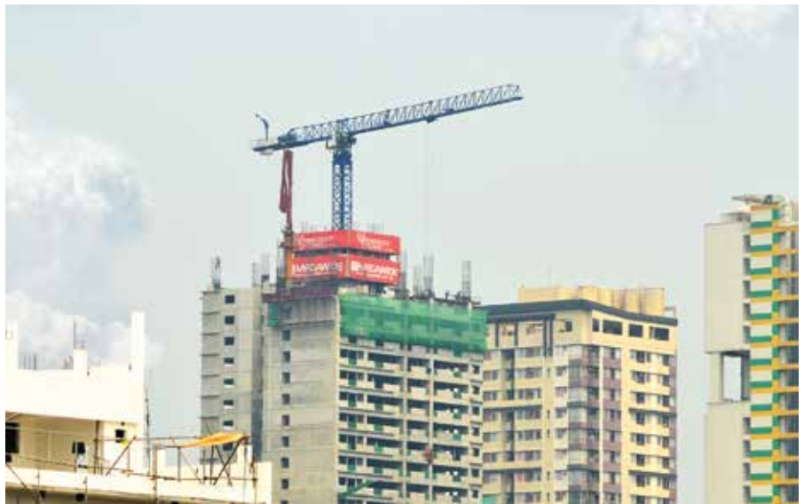
Comansa CM's 21CJ290 flat top tower crane on the University Tower P. Noval project.
