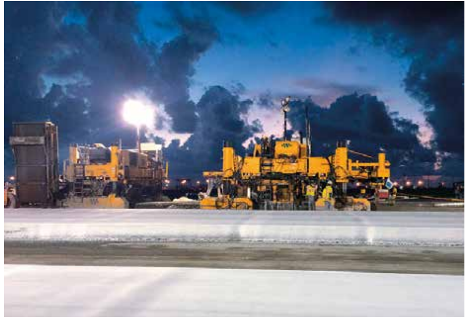
Above: Archer Western Construction slipformed the new 2,438 m southern runway with its Gomaco PS-2600 placer/spreader, GHP-2800 paver and T/C-600 texture/cure machine.
