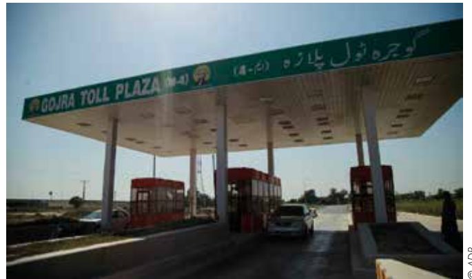
The Faisalabad to Gojra section of the M-4 has been completed.
