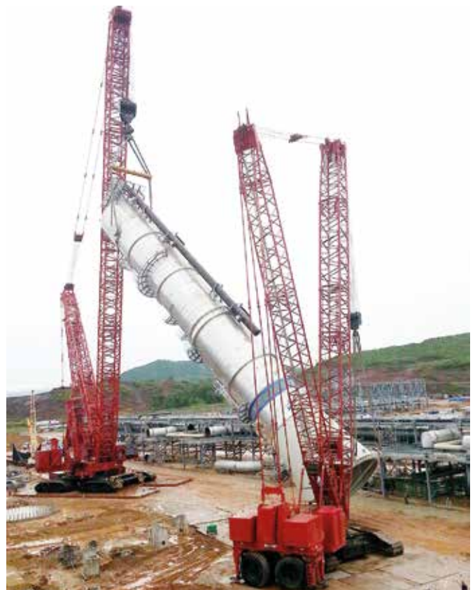
Manitowoc 31000 works on a petrochemical refinery project in Thanh Hoa province, Vietnam.
