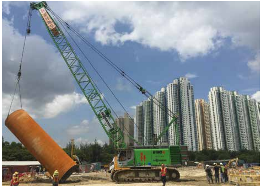
The 6130 HD crane performs foundation work for a new Hong Kong skyscraper.
