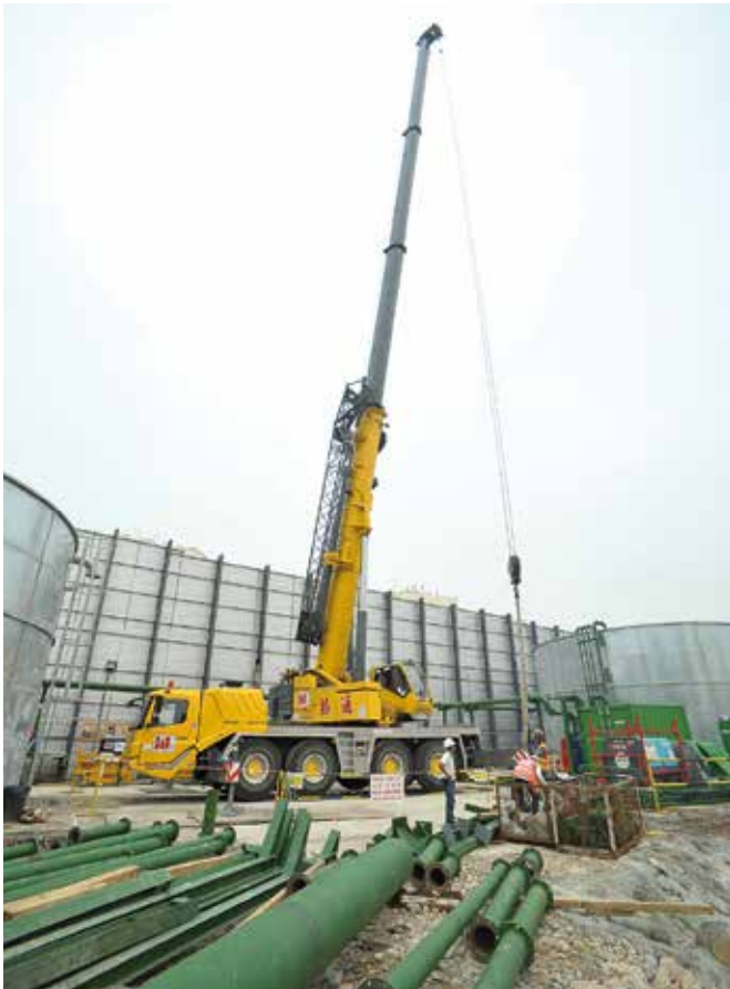
Grove GMK4100 being used at the Lentor MRT Station jobsite in Singapore.
