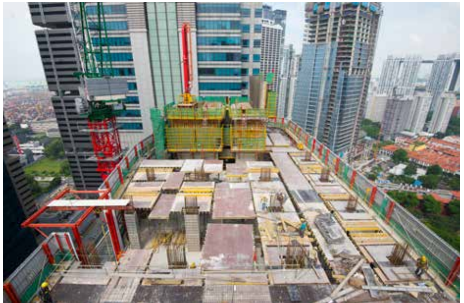
Above: Peri systems being used at the SBF Centre, a new commercial development in Singapore.
