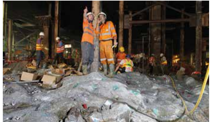
The Contract 810A is awarded to the Leighton-Gammon Joint Venture. The JV is excavating 1.7 mil cu m of earth, and placing 600,000 cu m of concrete and 150,000 t of steel reinforcement.
