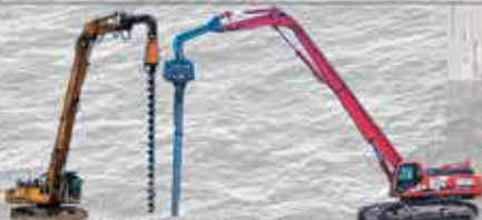
Excavator Auger / Vibro
