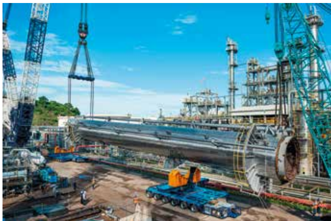
Loading the propylene fractionator on to the Goldhofer self propelled trailers.
