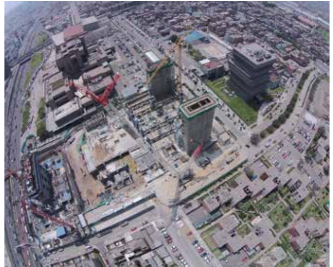
Having a tight deadline, Grúas y Maniobras used the Terex Superlift 3800 lattice boom crawler crane to help build the new convention centre.
