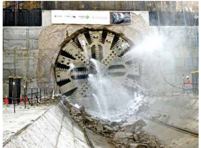
The 'San'ah' Metro TBM arrives at the Salah Al-Din station, having completed 1.2 km out of its designated 5 km within Line 5.
