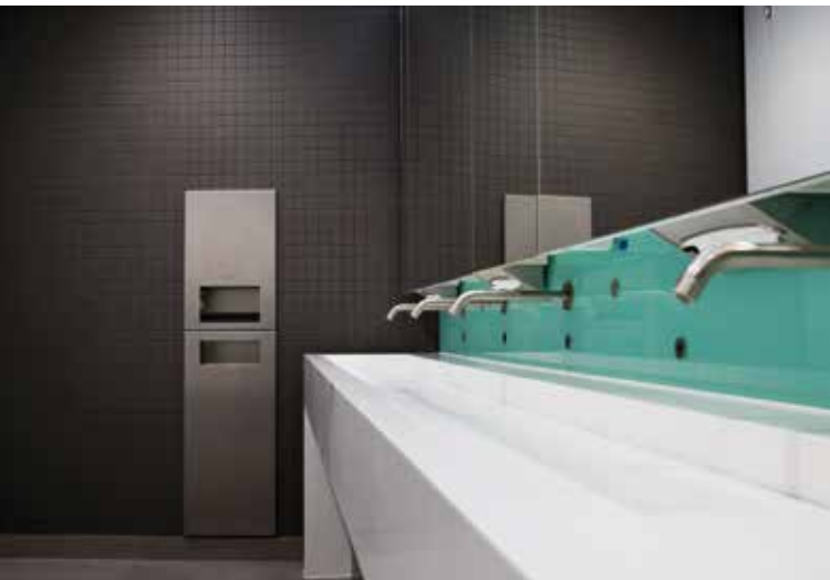
KERAFLEX cementitious adhesive was used to bond ceramic tiles on the toilettes' walls.
