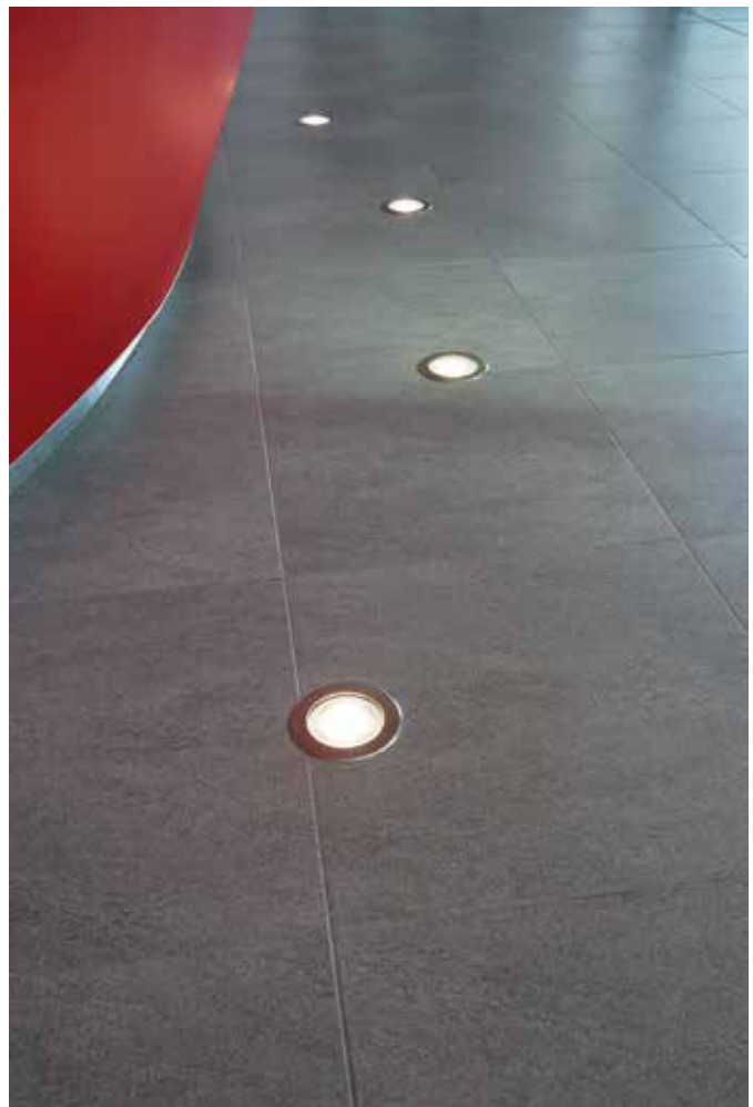
In all the involved areas the tile joints were grouted with ULTRACOLOR PLUS .
