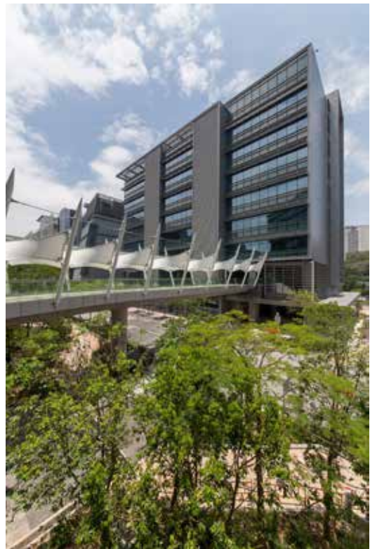
Building 15W in Hong Kong Science Park Phase 3 has garnered Final Platinum rating under Building Environmental Assessment Method (“BEAM Plus”) New Buildings V1.1 Final Assessment, the highest rating accredited by Hong Kong Green Building Council Limited (HKGBC) for its perfect integration of green technology and energy-efficient building design. This reinforced HKSTP’s effort in embracing sustainability and driving Hong Kong for its transformation into a smart city. Photo: © The Hong Kong Science and Technology Parks Corporation
