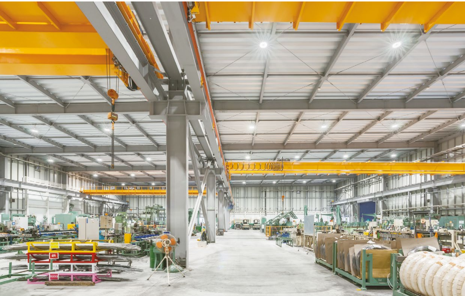
Sufficient brightness levels are achieved in the aisles, ensuring safety for handling incoming and outgoing products.
