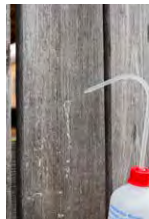
Passing the weathering test: even after 17 years of outdoor weathering, wood treated with the silicone resin is still water repellent. This affords a way of reliably protecting wood against moisture and wet for many years. Photo: Wacker Chemie AG
