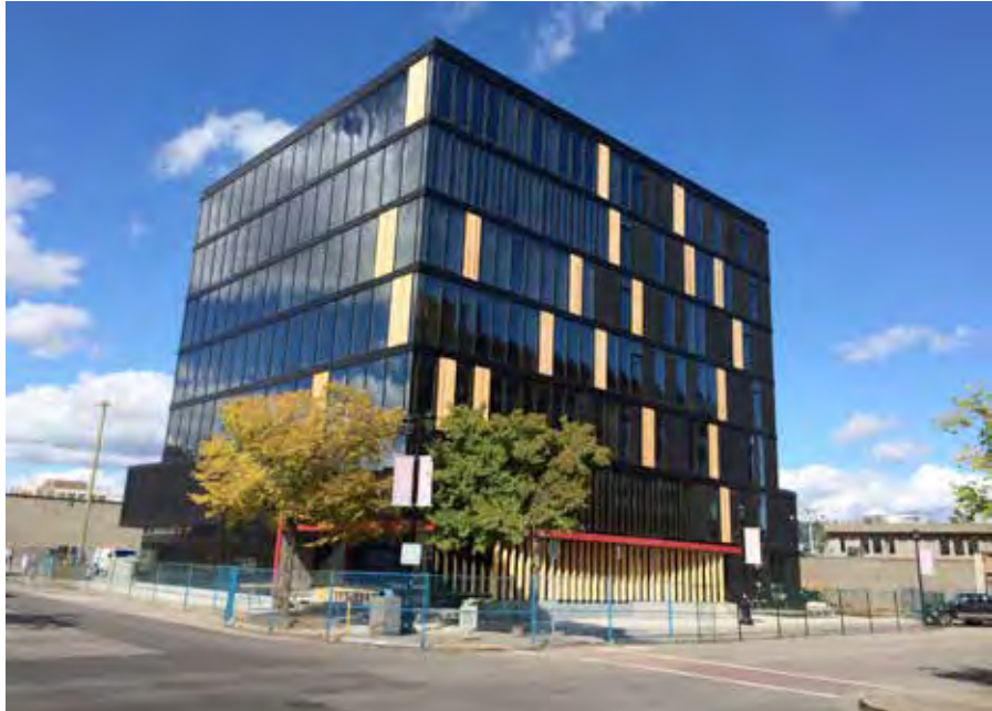
Wood Innovation and Design Centre in Prince George BC – the tallest wood building in North America.
