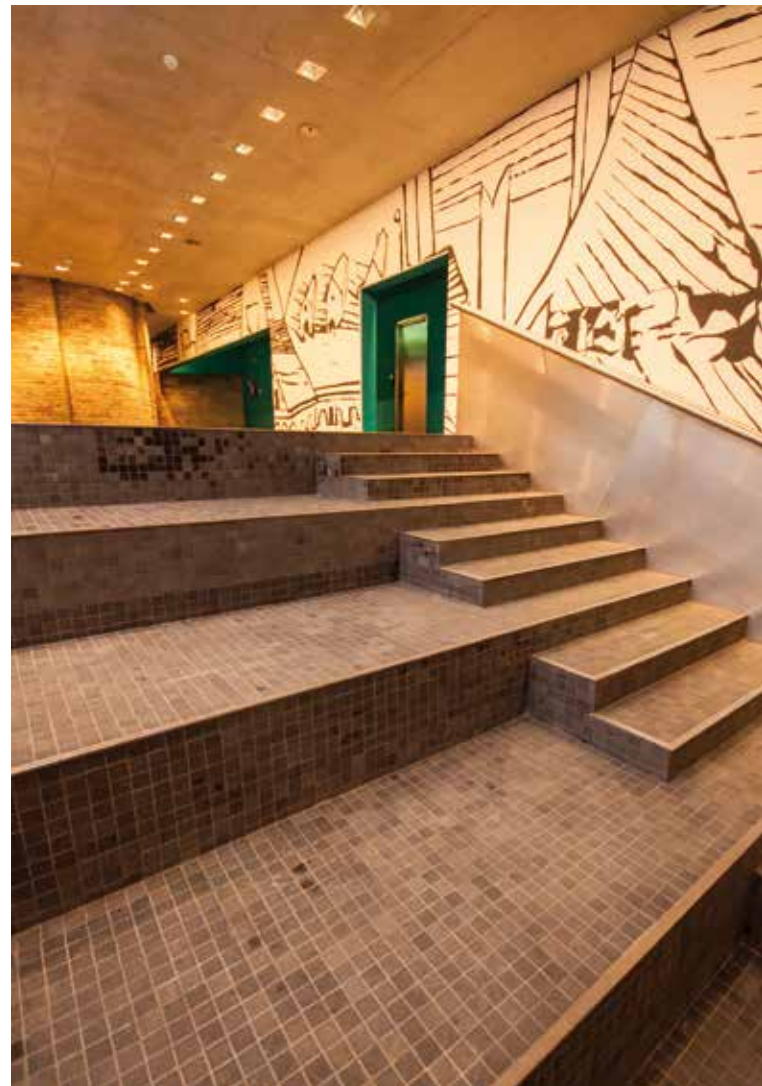
The floor substrates of the stairs, corridors, dressing rooms and bathrooms were first smoothed with PLANITOP FAST 330, then covered with porcelain tiles using KERAFLEX adhesive. Joints were grouted with KERACOLOR FF FLEX which is distributed on the Hungarian market by Mapei Kft.
