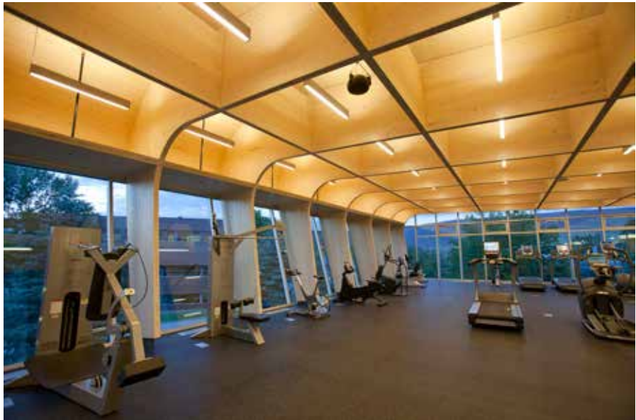
The University of British Columbia Okanagan Fitness Centre with one of a kind roof system.
