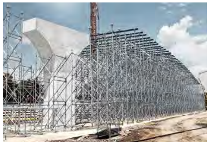
Doka d3 load-bearing tower.
