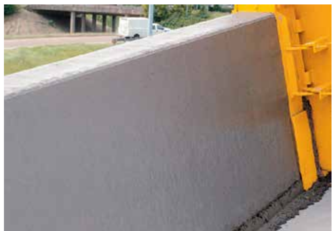
Left: WMC Contracting slipforms new bridge parapet on a flyover for the Memphis I-40/240 project. The company is working 33 m above ground level with its Gomaco 4400 barrier paver. Parapet production averages 244 m during a six-hour day.
