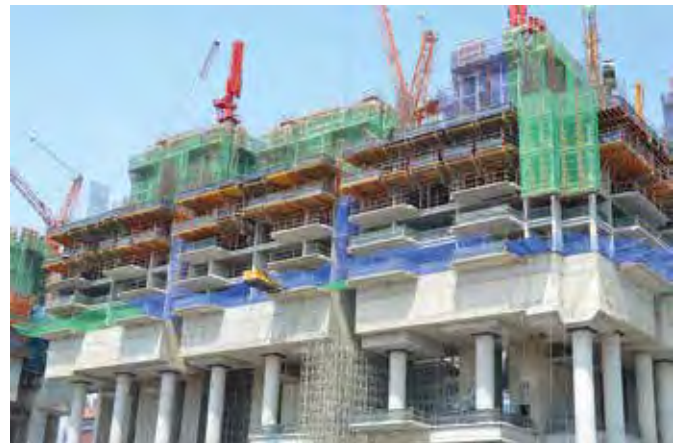
Below: The Skytable and RCS-P climbing protection panel on one of Marina One's residential towers.
