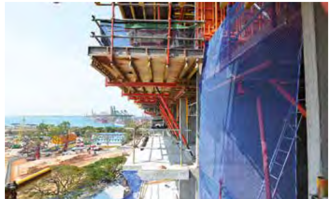
Above: Peri's Skytable system being used to support the staggered balconies on the Marina One development.
