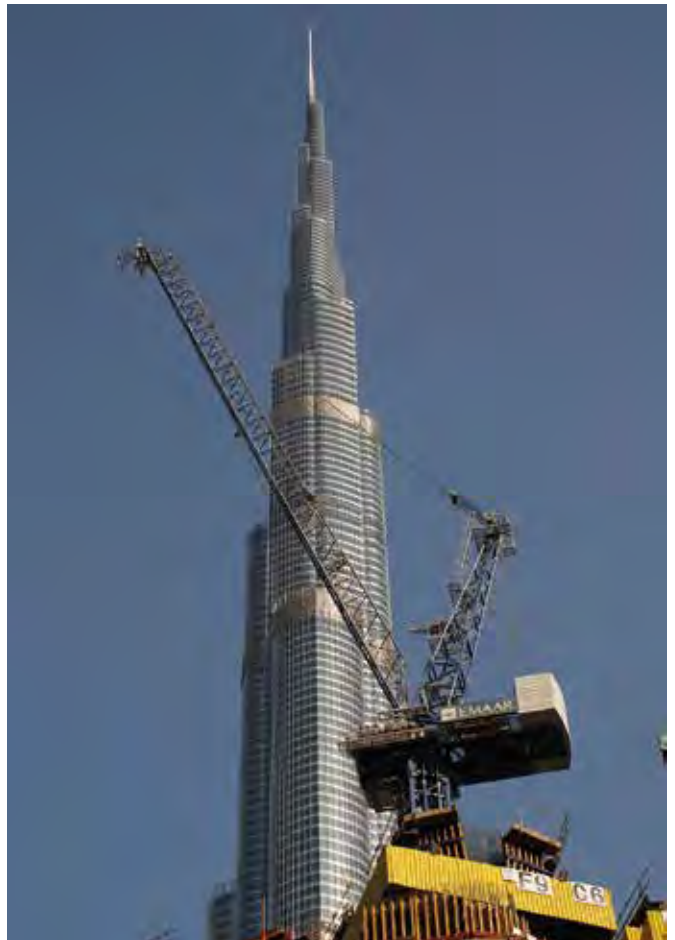
Linden Comansa LCL280 luffing-jib crane.
