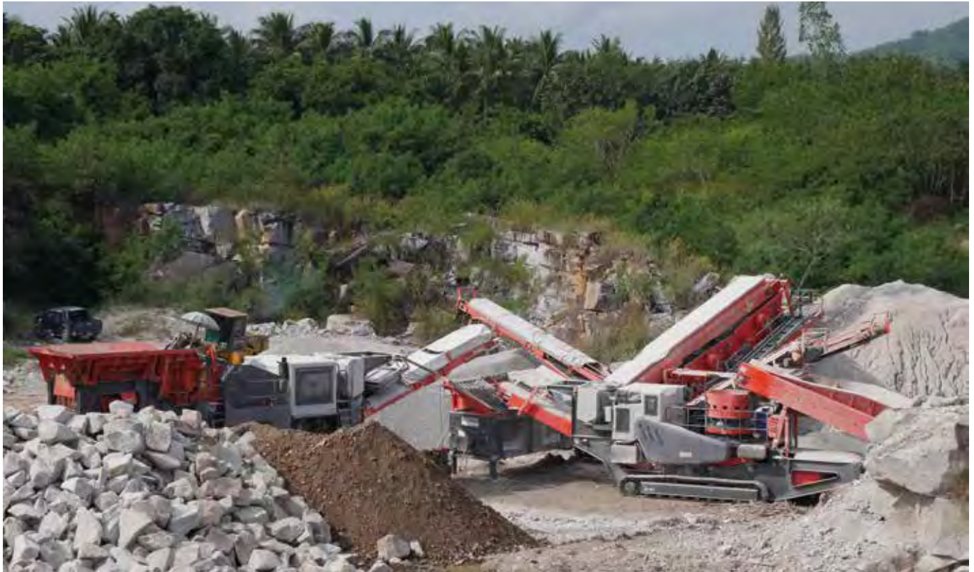
The Sandvik mobile screening and crushing plant currently works in closed circuit, in a 'star formation' designed to maximise the efficient production of the aggregates.
