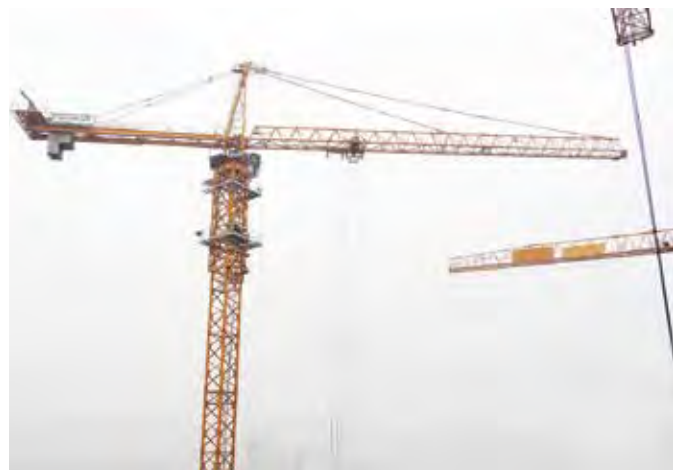
Second Harbor Engineering recently used Potain MC 480 tower cranes to help complete the largest project in its history – the 11 km long Hutong Yangtze Bridge.
