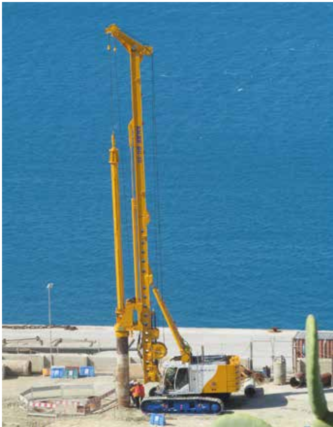
Bauer BG 30 ValueLine drilling rig.
