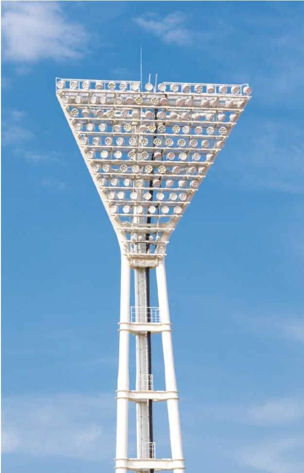
Left: The installed LEDioc FLOOD DUELL LED floodlights have been painted white to match the color of the lighting towers. Furthermore, 80W LEDioc FLOOD BLITZ have been installed on the lowest level of the lighting towers for event lighting.
