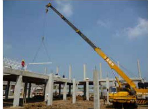
VCON Hollow Core Slabs and Precast Concrete installation. Photo: © VCON Group
