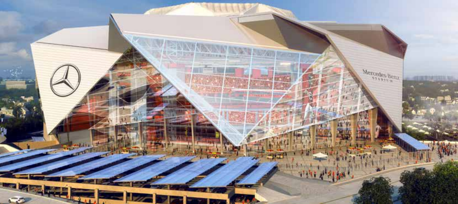
Mercedes-Benz Stadium's entry plaza. Photo: © HOK
