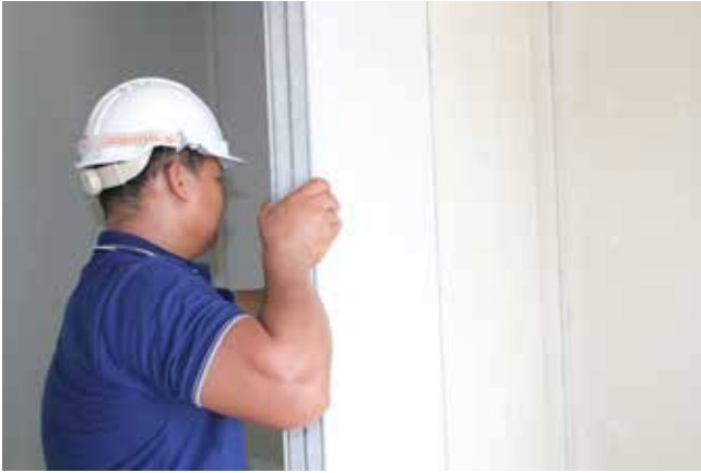
Worker installing a BB Wall Panel for fast and cost-efficient building construction.
