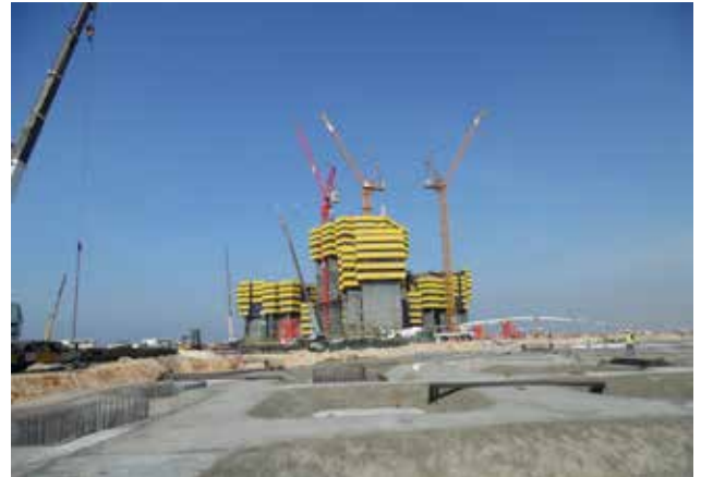
Kingdom Tower under construction. Photo: © Pinnacle
