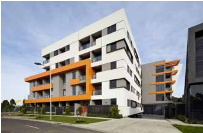
Exterior of The Green in Parkville, Melbourne, Australia. Photo supplied by Frasers Property Australia
