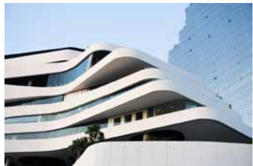
VCON white glass fiber reinforced concrete on the façade of Emquartier. Photo: © VCON Group
