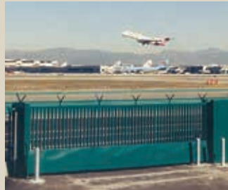
LOS ANGELES INTL. AIRPORT Delta SC3000 Sliding Gate
