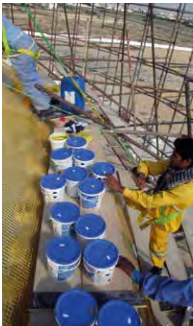
Above and below: Mapei system was applied on a 1,400 sq m area of the roof.
