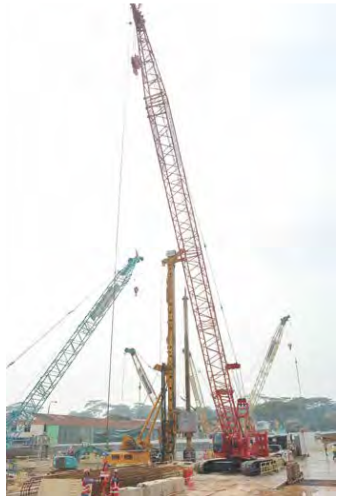
Left and right: Manitowoc's crawler cranes being used by Fuchi Pte Ltd to support strutting and waler positioning efforts at Springleaf MRT Station in Singapore.
