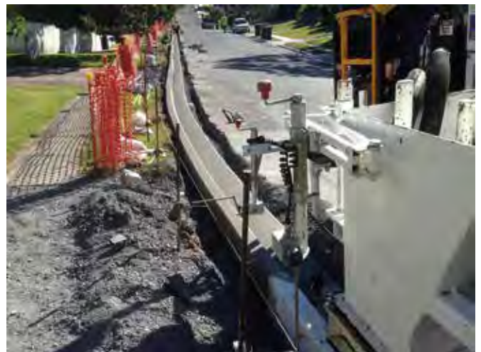
Left and below (left and right): Two Arrow 750XL customised slipform kerb machines have been chosen by the Brisbane City Council for its kerb replacement programme.
