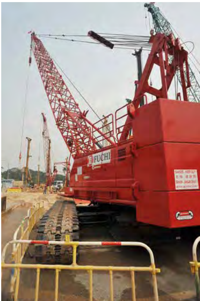
Left and right: Manitowoc's crawler cranes being used by Fuchi Pte Ltd to support strutting and waler positioning efforts at Springleaf MRT Station in Singapore.
