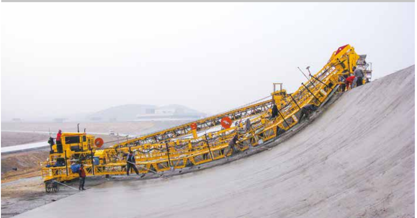
Above and below: The track's shape was constantly changing as it went from flat to curved sections. It created a design challenge for Gomaco.
