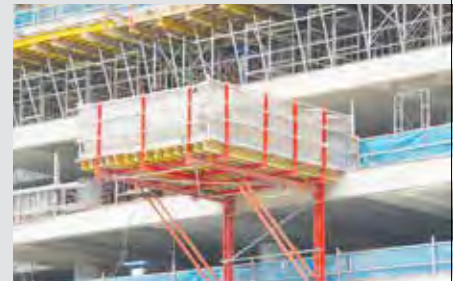
RCS Landing Platform for easy lifting of PD-8 Tables and loose formwork
