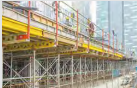
PD 8 Table with handrails for safe work at construction level
