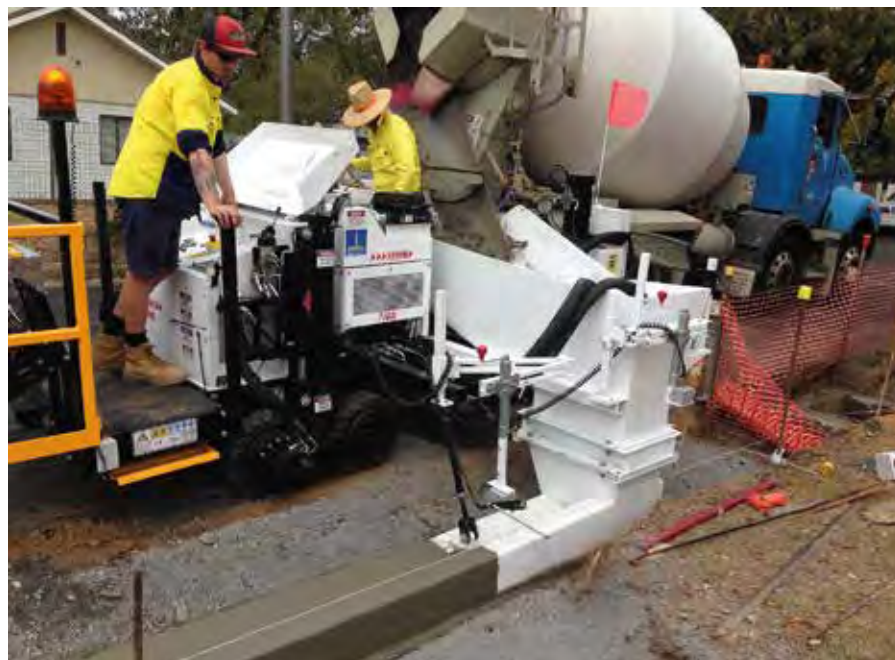
Left and below (left and right): Two Arrow 750XL customised slipform kerb machines have been chosen by the Brisbane City Council for its kerb replacement programme.
