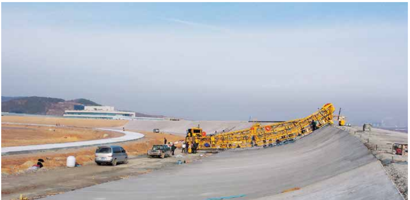
Above and below: The track's shape was constantly changing as it went from flat to curved sections. It created a design challenge for Gomaco.
