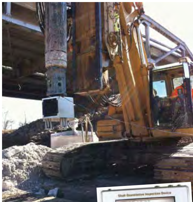
Above and inset: Pile Dynamics' Shaft Quantitative Inspection Device is an alternative to the camera-based visual inspection of the excavated shaft base.
