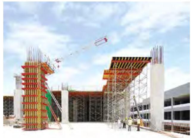
Peri has supplied its formwork systems to build a new warehouse facility in Singapore. Here is a view of Peri PD 8 slab table and Vario GT 24 column formwork from outside the building.
