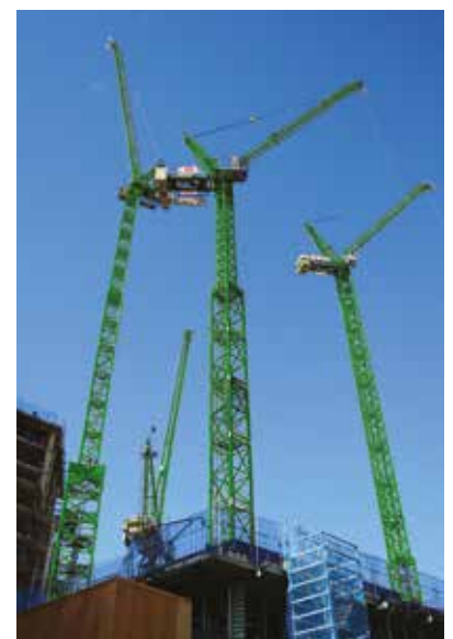
Jaso tower cranes.
