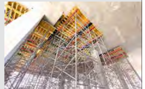
PD 8 slab table for clear heights up to 9.50m
