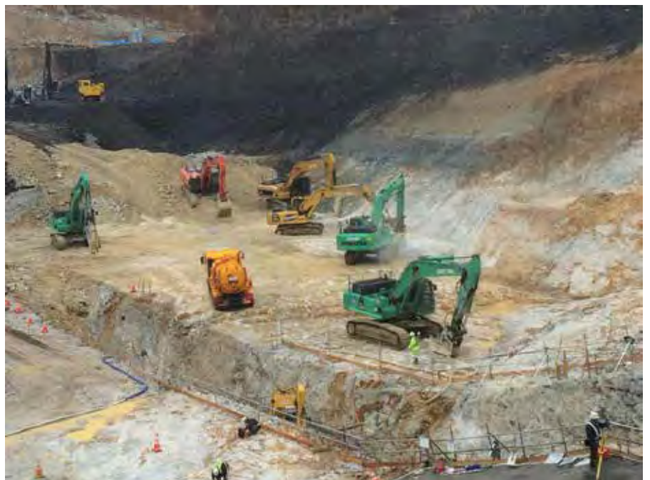
Above, left and below: Tomijima equipped five excavators and five dozers with the Trimble GCS900 Grade Control System. The company has also utilised four Site Positioning Systems Essentials Kits and deployed Trimble SPS620 total stations to conduct high accuracy structural works and checks. Plus, it adopted VisionLink site productivity technology from Trimble for a holistic view of the project site and to track site productivity and materials movement.
