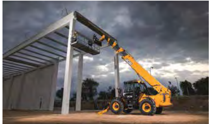
A JCB Loadall telehandler on a jobsite.
