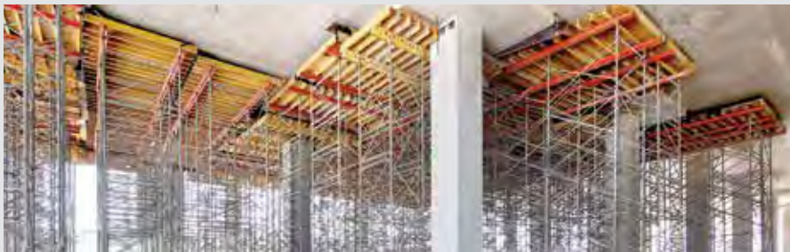
PD 8 slab table has been dismantled and moved to another casting
