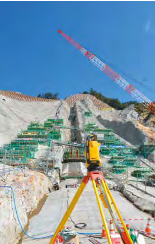
Above, left and below: Tomijima equipped five excavators and five dozers with the Trimble GCS900 Grade Control System. The company has also utilised four Site Positioning Systems Essentials Kits and deployed Trimble SPS620 total stations to conduct high accuracy structural works and checks. Plus, it adopted VisionLink site productivity technology from Trimble for a holistic view of the project site and to track site productivity and materials movement.
