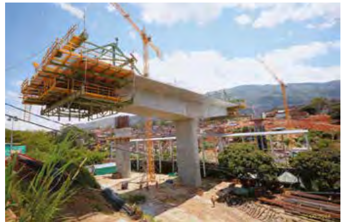
Alsina formwork system being used on a bridge project.
