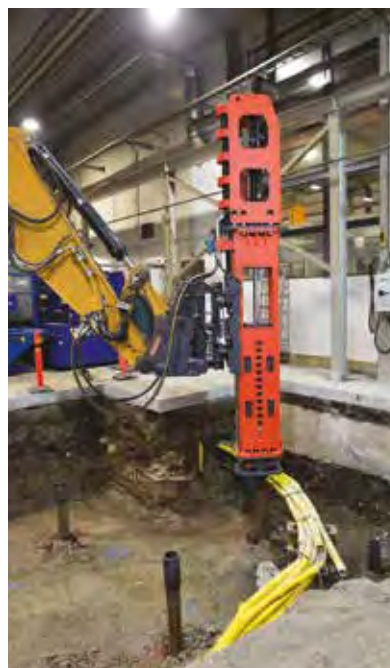
Movax DH-20 piling hammer.
