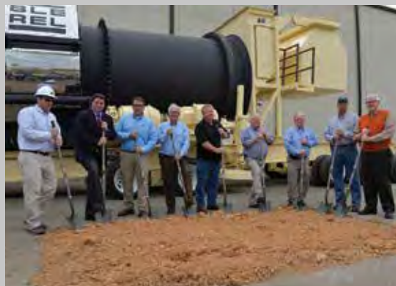
Work on Astec's new facility has begun.
