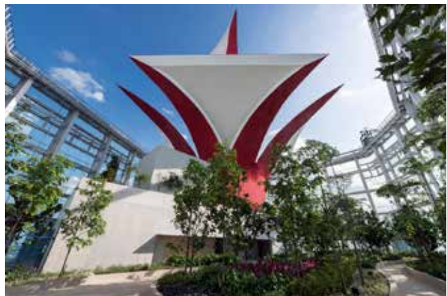
The crown of the CapitaGreen building is marked by a distinctive red and white sculptural petalled wind scoop. Photo: © CapitaLand
