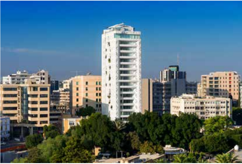
The White Walls. Photo: © Yiorgis Yerolymbos, Courtesy of Nice Day Developments
