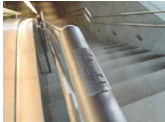
English Braille / tactile indicators at the start and end of the stairway, from CapitaGreen to the pedestrian underpass in the CapitaGreen. Photo: © CapitaLand
