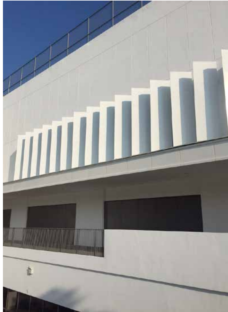
Aluminium sun-shading devices designed at the north and south façades of the indoor sports hall, The Box. Photo: © DP Architects
