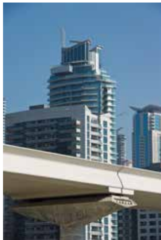
The Dubai Metro network is a fully automated and driverless system running on two lines. SILRES® BS 290 was applied as a primer and as an anti-carbonation top coat. (Photos: WACKER)
