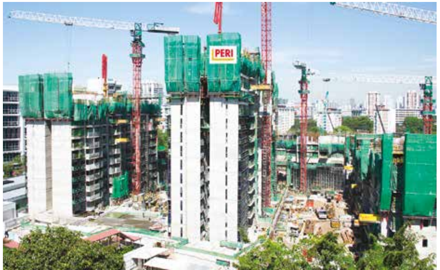
Above: Sims Urban Oasis under construction.
