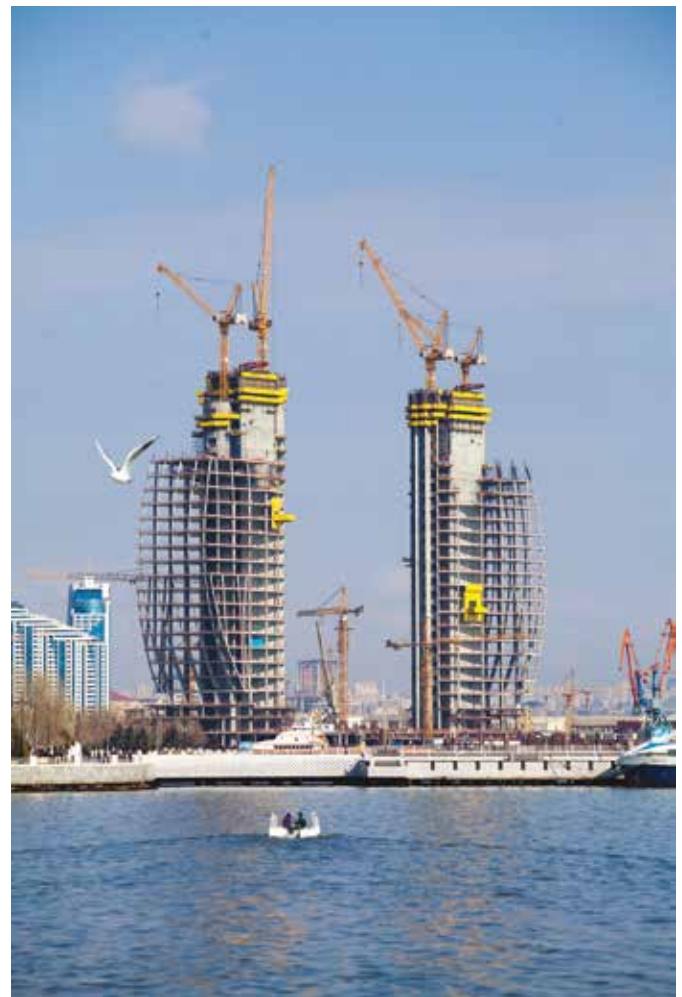
Right: Four Liebherr luffing jib tower cranes at the construction of The Crescent Hotel in Baku.
