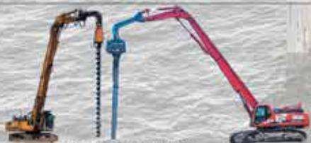
Excavator Auger / Vibro
