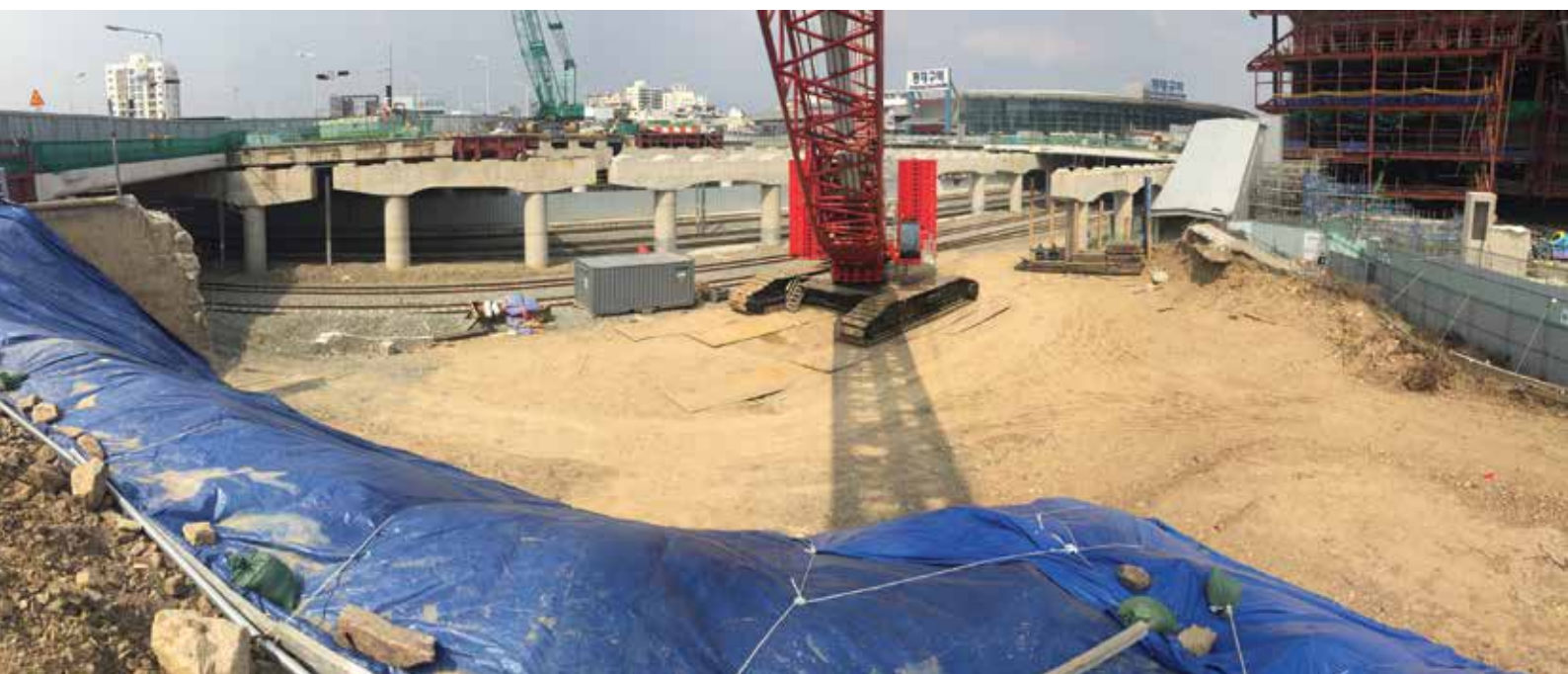
Doosan Heavy Industries & Construction performs heavy lifting operations at a congested railway station jobsite in Daegu City, South Korea, using a Manitowoc MLC650 crawler crane. The machine features a 68 m main boom with the VPC-MAX attachment.
