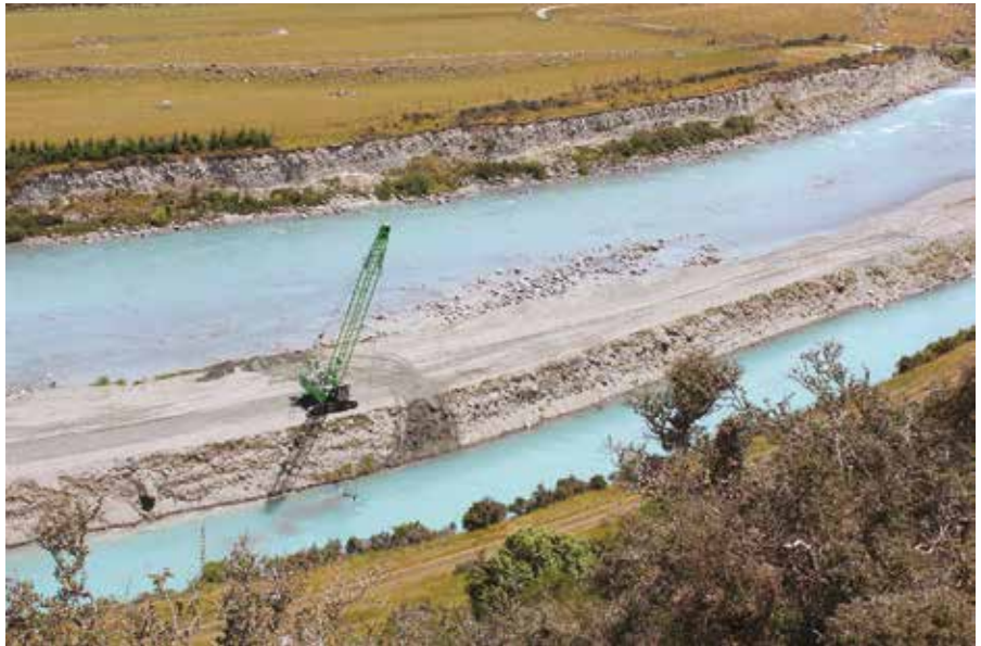
Sennebogen 655 duty cycle crane helps to clean sand and gravel from the riverbed of the Rangitata Canal in New Zealand.
