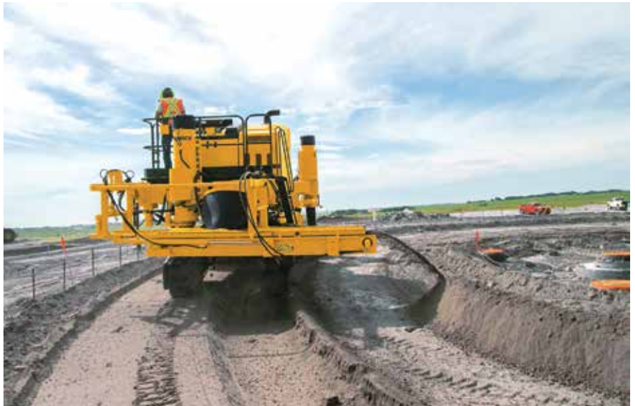
Marmot's Gomaco Commander III high-production trimmer cuts through the clay-based and rocky soil found in Calgary, Alberta, Canada.
