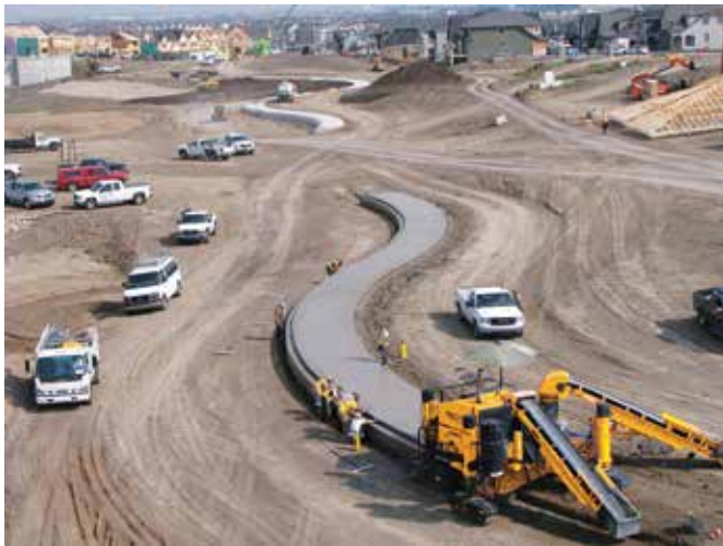
Above: The three-track Commander III machine, with an extra concrete conveyor, slipforms 800 m of the profile at the Mahogany Central Beach site in Calgary.
