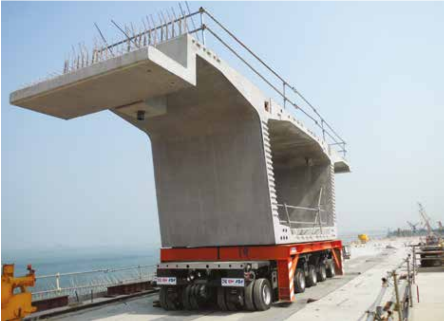
Nicolas vehicle transports precast bridge elements on the HZMB project.
