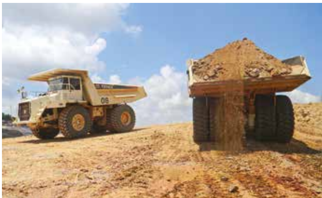
TR60 rigid trucks work on a project in Indonesia.
