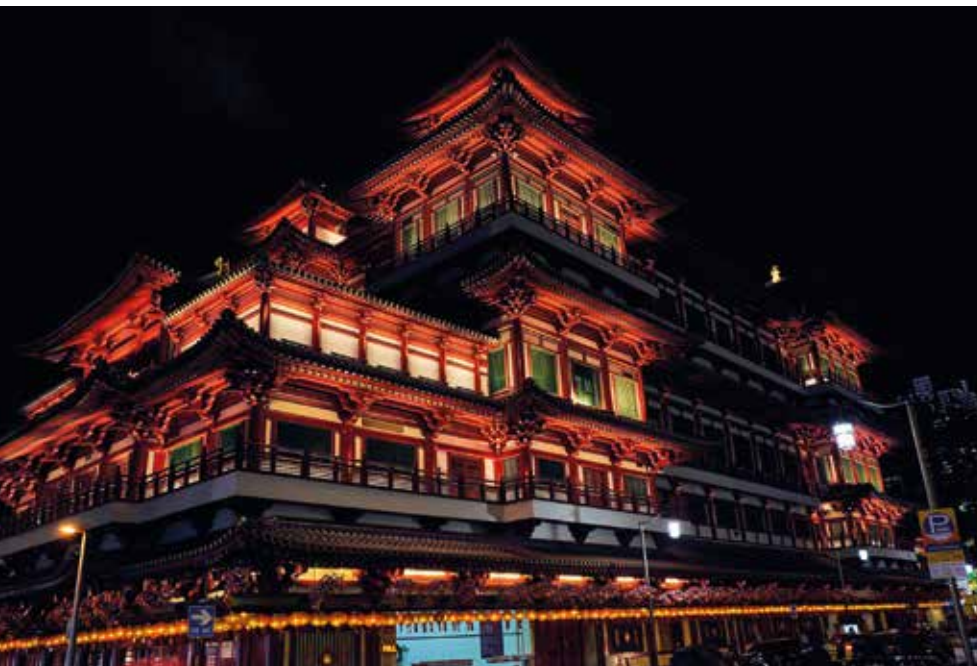
After upgrading. Photo: © Aurecon
