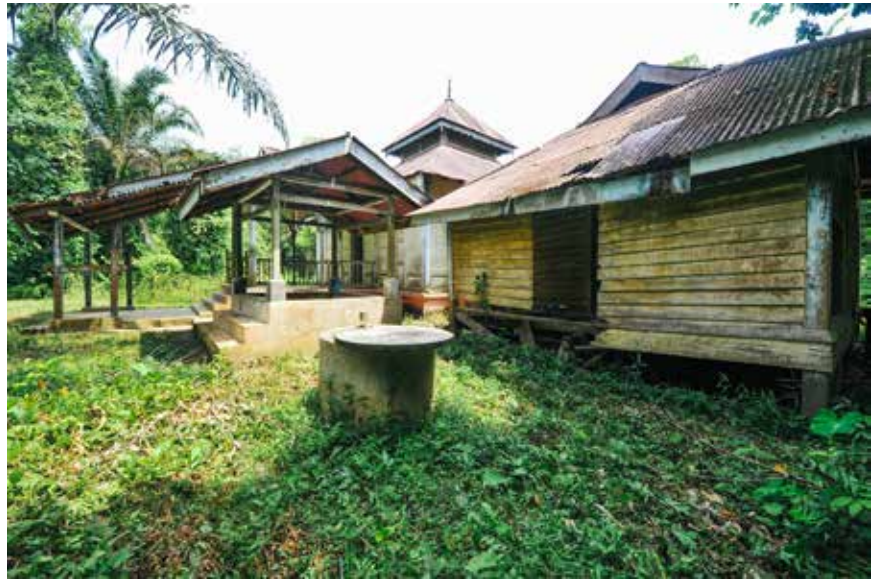
View towards the balai lintang and kolah structure. Photo: © ATSA Architects Sdn Bhd
