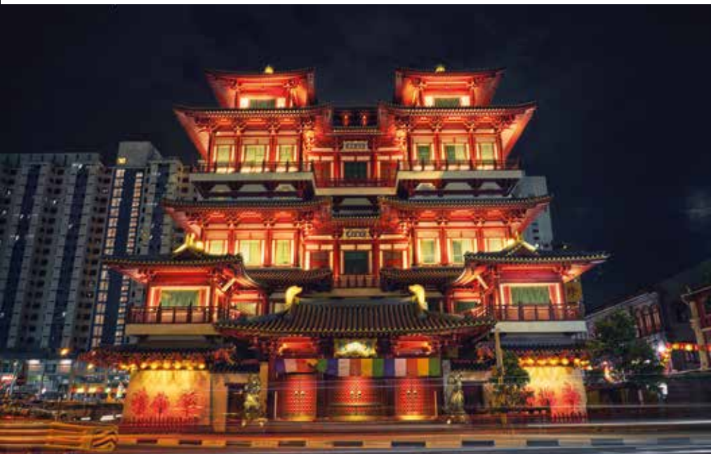
After upgrading. Photo: © Aurecon
