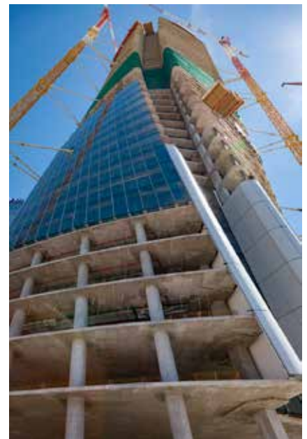
Generali Tower under construction. Image by Alberto Fanelli @ Citylife
