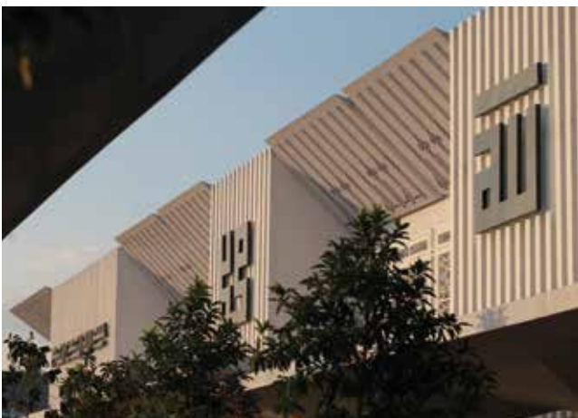
Detailed view of the GRAC wall panels.
