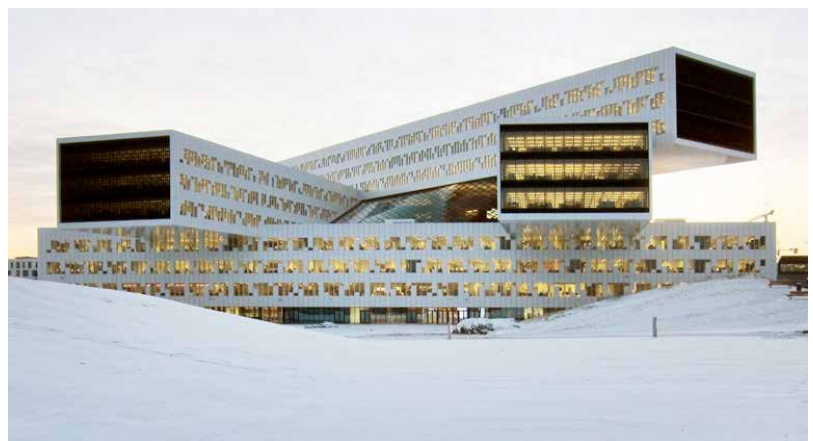
Statoil Building in Oslo Fjord. Photo: © Elval Colour S.A.
