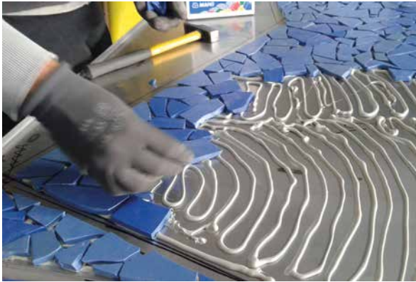
Fragments of ceramic tiles were bonded to steel panels with MAPEFLEX PU 45.
