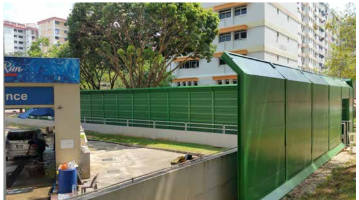
Permanent Noise Control Barrier - Town Council Project, used in Petrol Station. Photo: © Jinbiao
