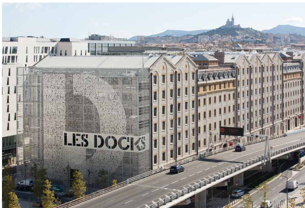
Les Docks Village is a large, iconic building in the Joliette area of Marseille.
