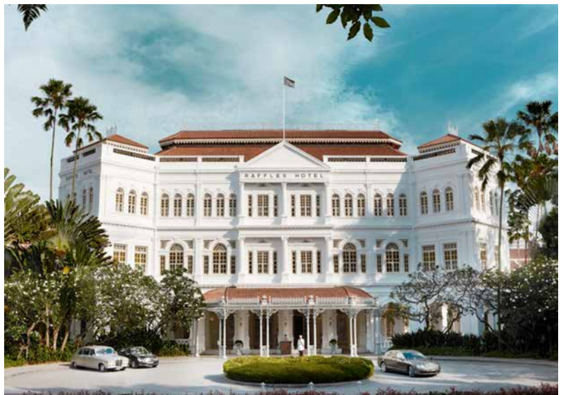
Raffles Hotel Singapore Façade. Photo: © Raffles Hotel Singapore
