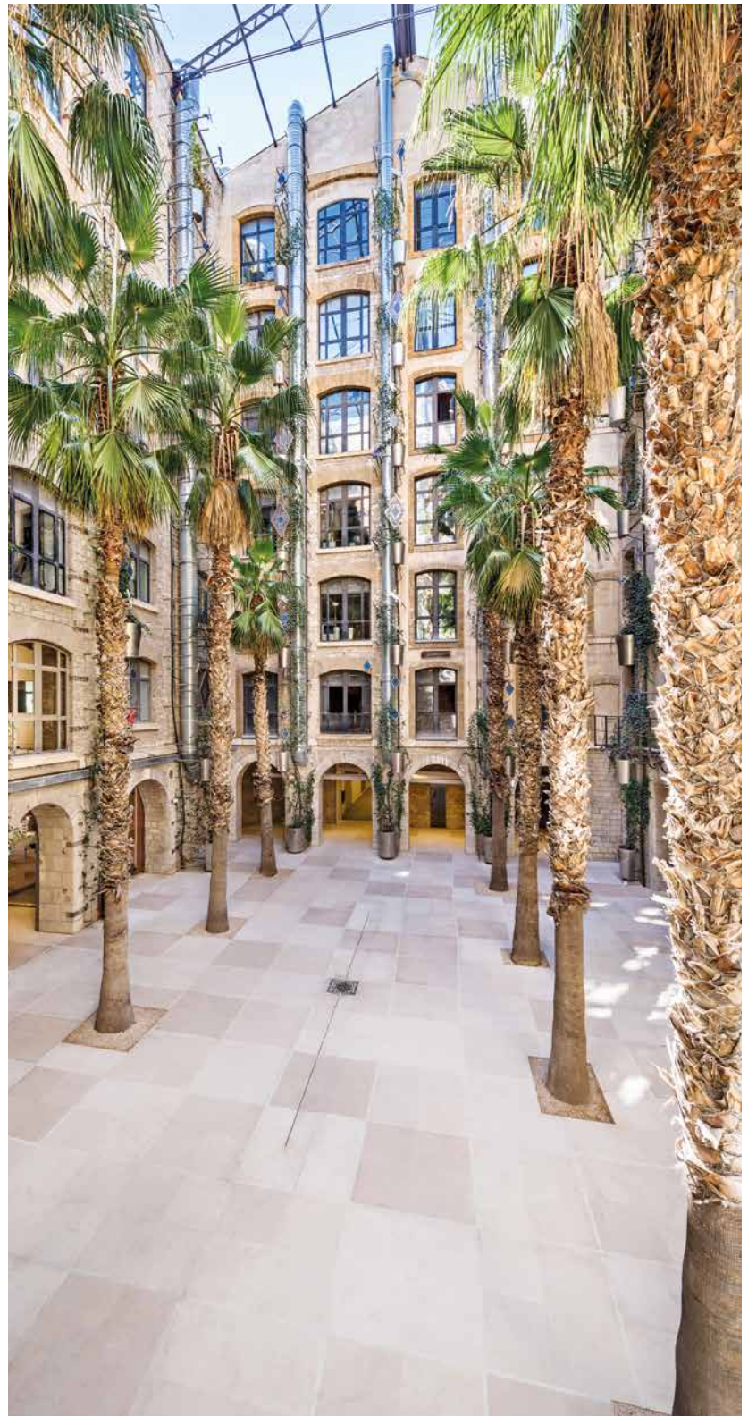
1,300 m 2 of Moleanos stone slabs were bonded to the floors in Place des Palmiers and Place du Marché squares with KERAFLEX S1. The joints were grouted with ULTRACOLOR PLUS.
