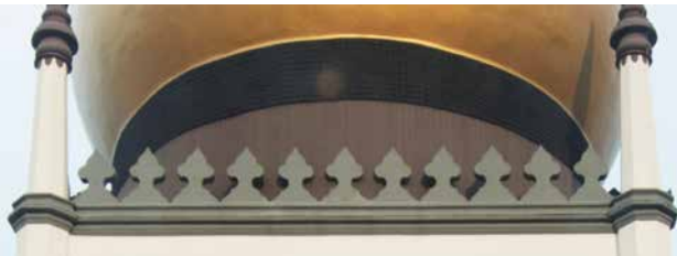
Plaster details cleaned, restored and repainted in new scheme with consideration of maintenance. Photo: © Urban Redevelopment Authority. All rights reserved.
