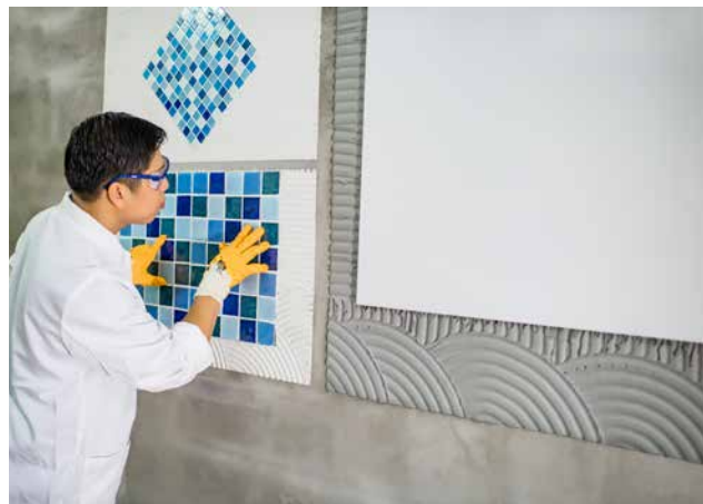
Experts at the new "Application House" will demonstrate the advantages of WACKER's construction chemicals in different applications. (Photo: Wacker Chemie AG)
