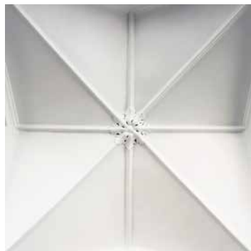
Restored ceiling ribs. Photo: © Urban Redevelopment Authority. All rights reserved.
