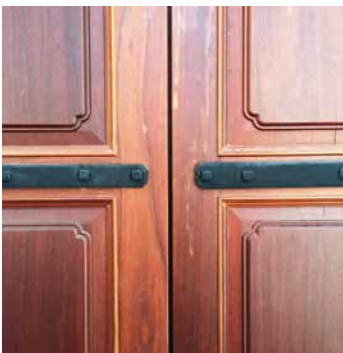
Old timber doors reconditioned. Photo: © Urban Redevelopment Authority. All rights reserved.
