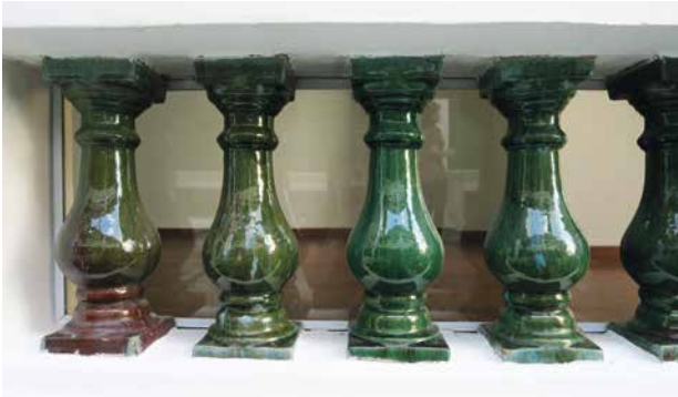
Glazed balustrades cleaned. Photo: © Urban Redevelopment Authority. All rights reserved.
