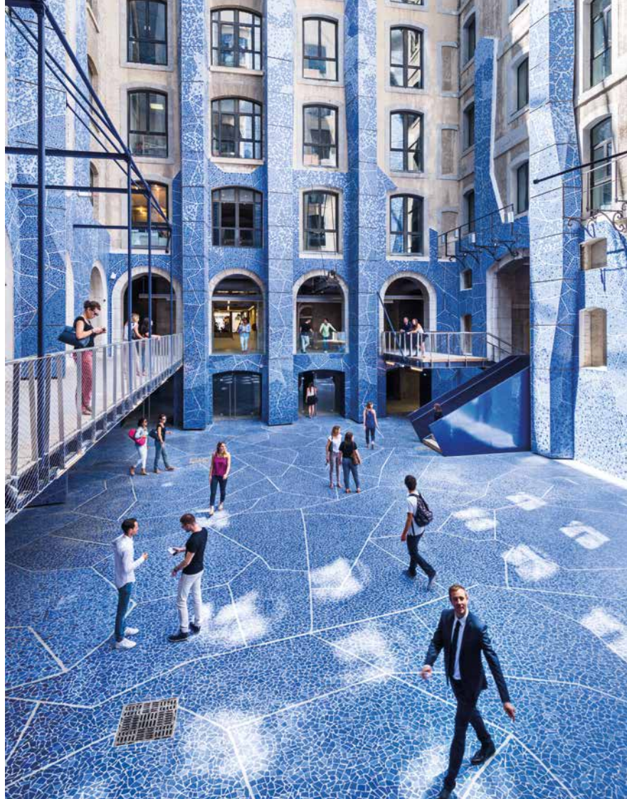
In Place du Port square the mosaics were installed on over 780 panels using Mapei products.
