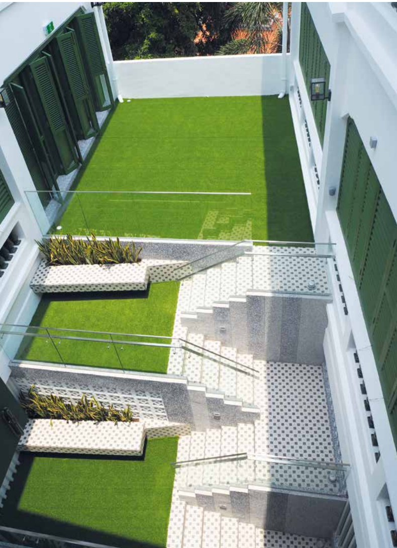
Open rear court recovered. Photo: © Urban Redevelopment Authority. All rights reserved.
