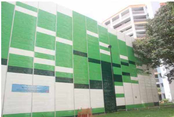
Temporary Noise Control Barrier - MOH Project, future Polyclinic. Barrier with a 'tree' design. Photo: © Jinbiao
