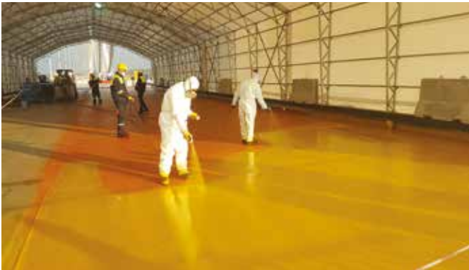
Above and left: Stirling Lloyd's Eliminator system being applied on the Yavuz Sultan Selim Bridge, covering a total of 37,435 sq m.
