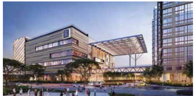
Top and above: Lendlease's S$3.2 bil Paya Lebar Quarter urban regeneration project will be a significant landmark of URA's 12-ha Paya Lebar Central development.
