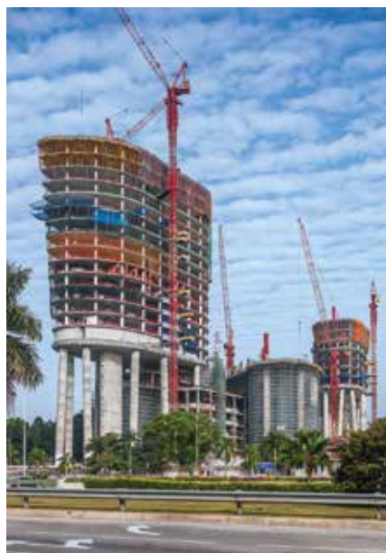
Above: On the basis of the RCS rail climbing system, the inclined circular columns could be efficiently constructed.
