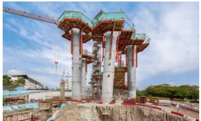
Above: On the basis of the RCS rail climbing system, the inclined circular columns could be efficiently constructed.
