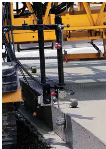
Top: The Gomaco T/C-600 texture/cure machine applies a white spray cure and longitudinal tine finish to the new Interstate 376.
