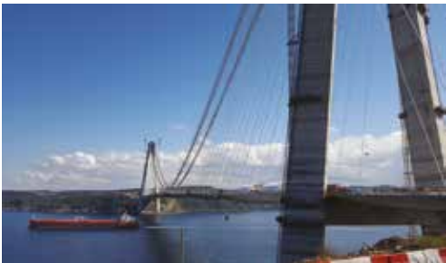
Above and left: Stirling Lloyd's Eliminator system being applied on the Yavuz Sultan Selim Bridge, covering a total of 37,435 sq m.
