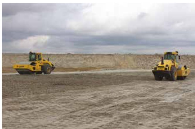
Above and right The BCM 05 compaction control system and the Bomag GPS system ensure that the daily compaction checks required are documented smoothly.
