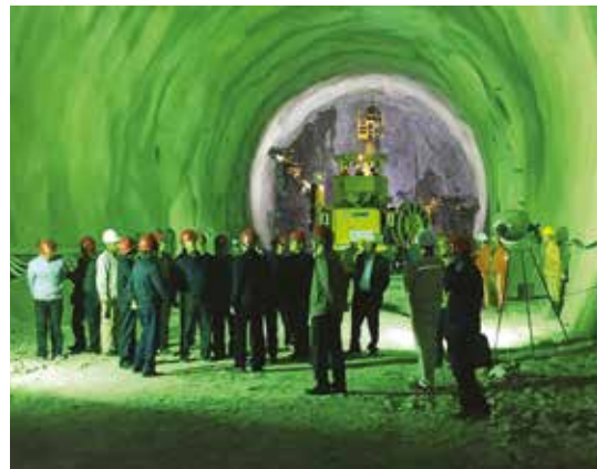
Far left and left: The XCMG TZ3A hydraulic rock drill jumbo plays role in the Mongolia-China railway project.
