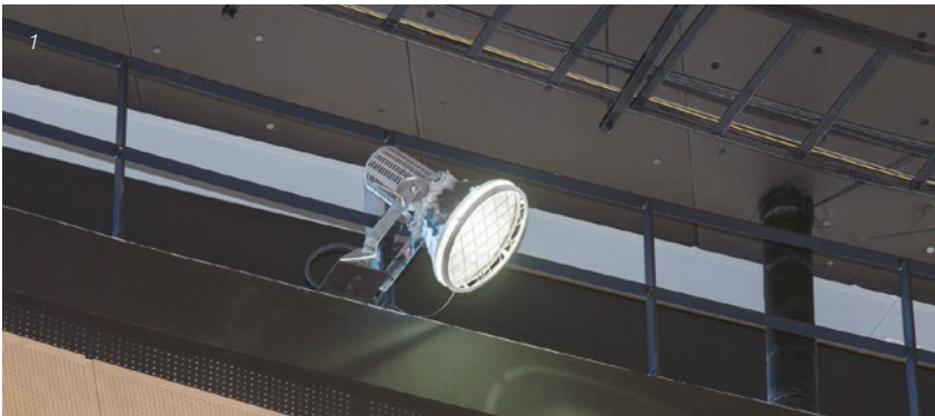
1 - The 210W LEDioc FLOOD SPOLART LED floodlights turned on
