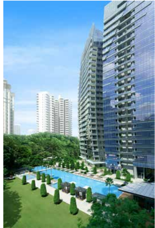
Gramercy Park stands out with its unique sculptural design featuring two curvilinear towers. Photo: © City Developments Limited
