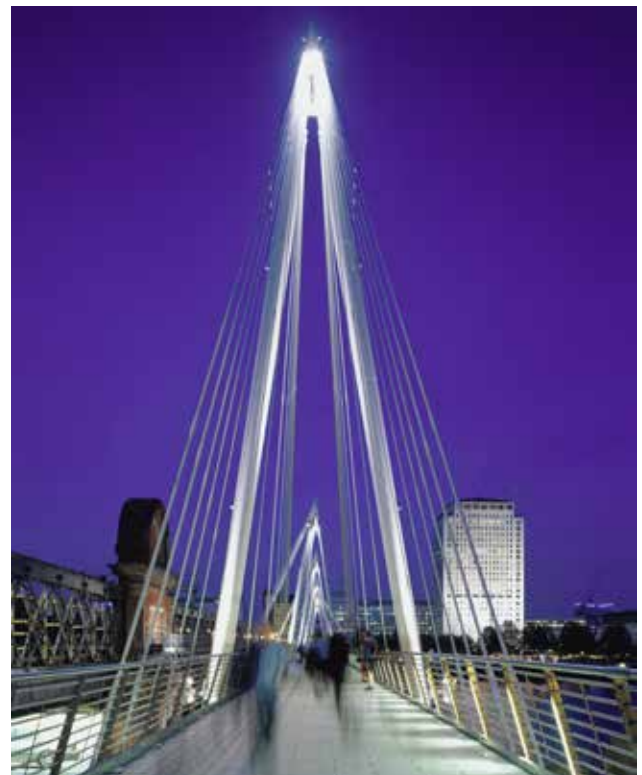
Hungerford Bridge London Architect: Lifschutz Davidson Sandilands Photo: © Tim James
