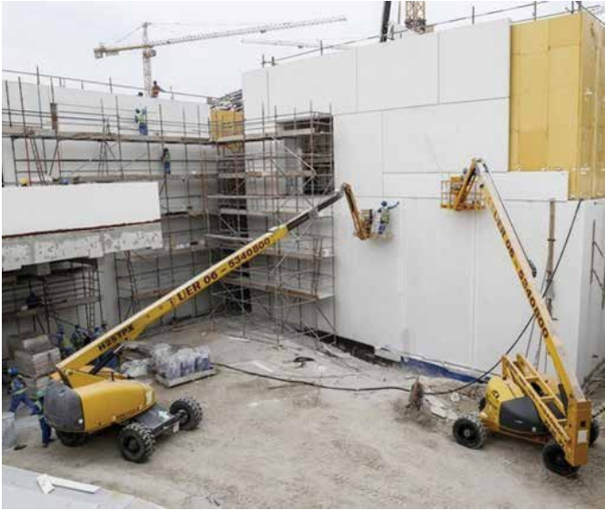
Above and left: Haulotte aerial platforms have been used in the construction of Louvre museum in Abu Dhabi. Supplied by United Gulf Equipment (UGER), most of them comprised diesel articulated and telescopic big booms.
