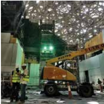
Above and left: Haulotte aerial platforms have been used in the construction of Louvre museum in Abu Dhabi. Supplied by United Gulf Equipment (UGER), most of them comprised diesel articulated and telescopic big booms.
