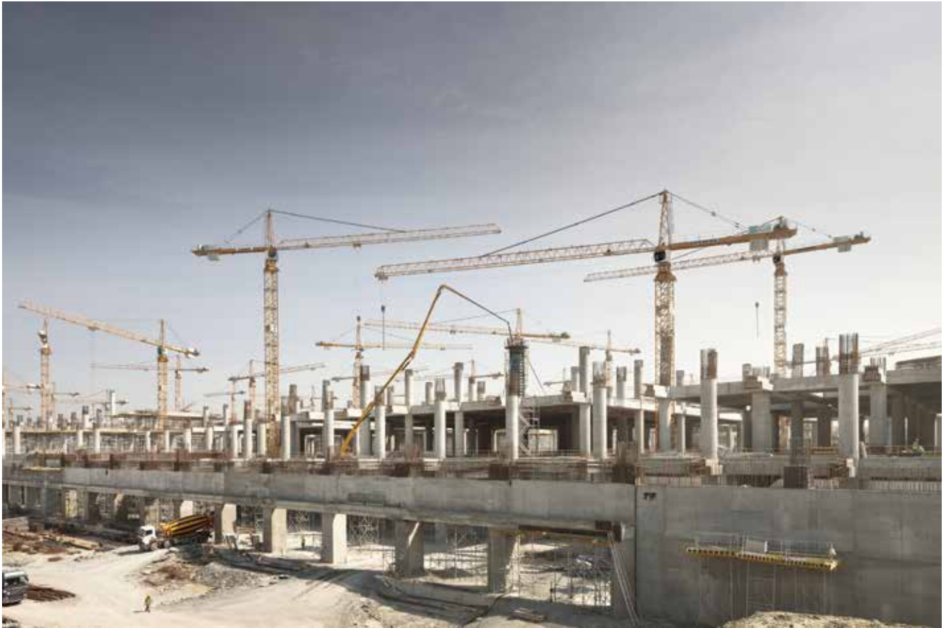
Above and left: Liebherr has delivered a total of 58 tower cranes for the project, which will be used for a variety of lifting tasks. The cranes include the 154 EC H, 280 EC H and 200 EC H models.
