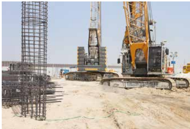
Above and left: Dutco Balfour Beatty uses four Liebherr machines to carry out piling operations at Expo Village in Dubai. Among them is a Liebherr HS 8100 HD duty cycle crawler crane, which has been modified to help increase productivity on the job.
