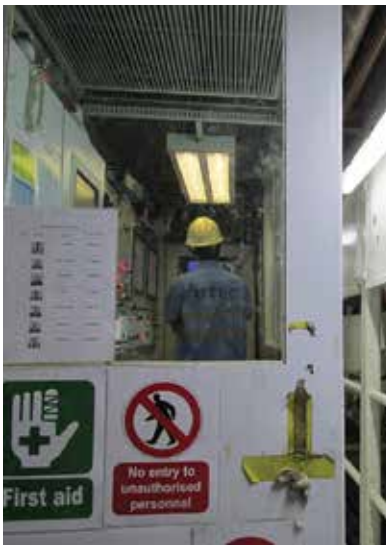
Top and above: One of the slurry TBMs in operation.
