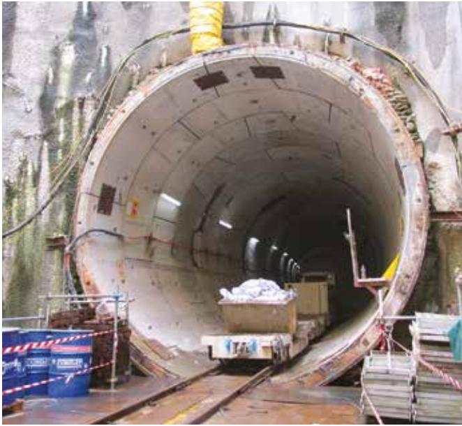
Above and left: The tunnel linings are made of steel fibre reinforced concrete (above), making them more durable and fire-resistant.
