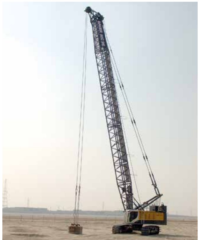
Above and below: A new district is currently under construction in Abu Dhabi to provide homes for 22,000 people. Here, a Bauer MC 96 duty-cycle crane (below) is used for ground compaction.
