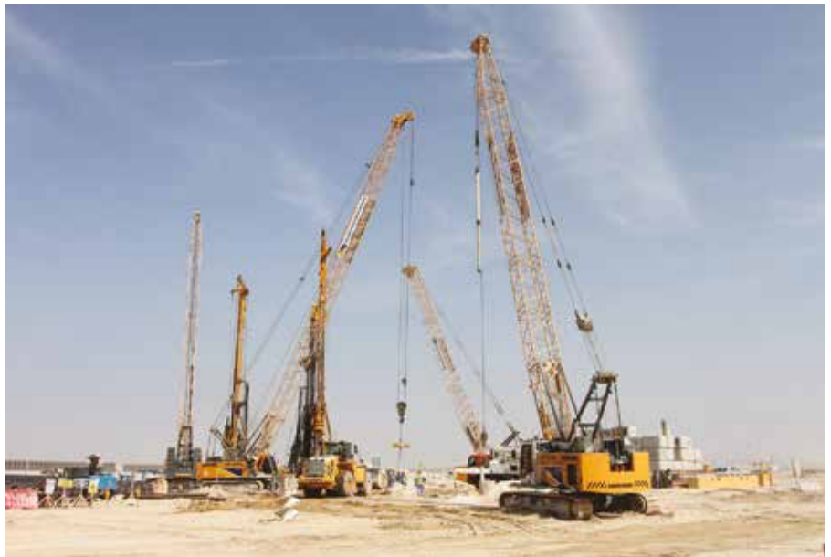
Above and left: Dutco Balfour Beatty uses four Liebherr machines to carry out piling operations at Expo Village in Dubai. Among them is a Liebherr HS 8100 HD duty cycle crawler crane, which has been modified to help increase productivity on the job.
