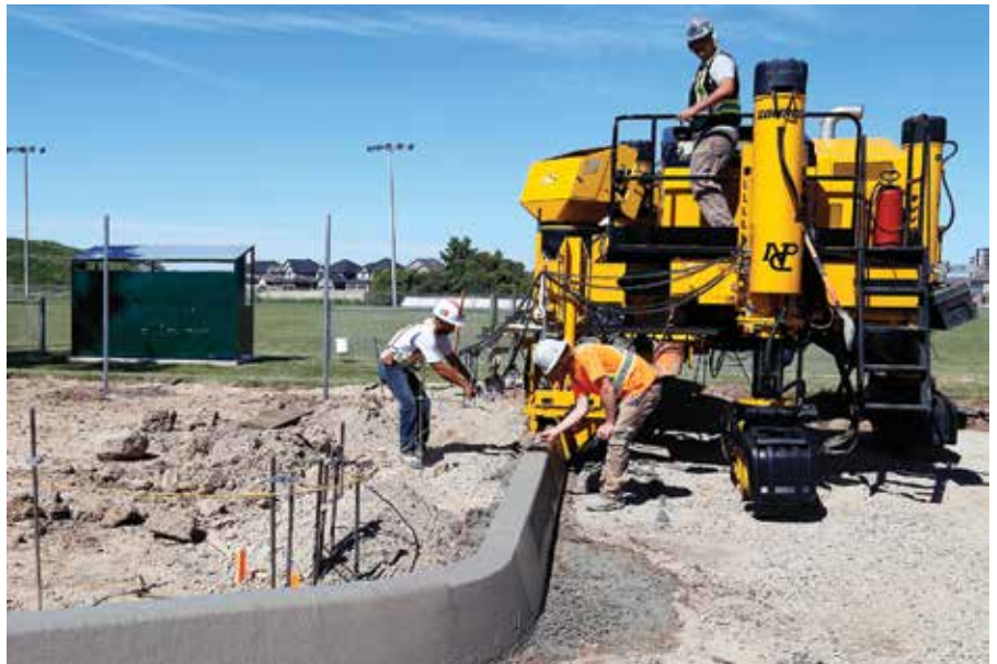
Gomaco's three-track Commander III Xtreme has the ability to slipform a 610 mm radius.
