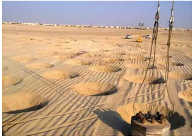
Above and below: A new district is currently under construction in Abu Dhabi to provide homes for 22,000 people. Here, a Bauer MC 96 duty-cycle crane (below) is used for ground compaction.
