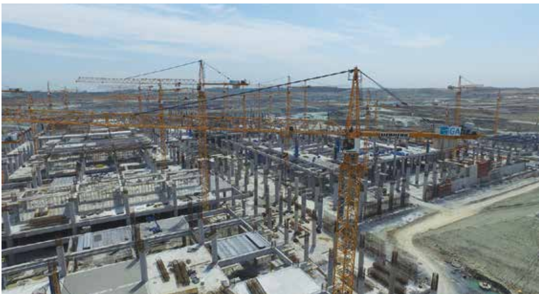
Above and left: Liebherr has delivered a total of 58 tower cranes for the project, which will be used for a variety of lifting tasks. The cranes include the 154 EC H, 280 EC H and 200 EC H models.
