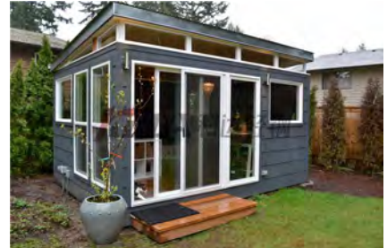
Keda Light Steel recently completed a new prefab house in Malaysia. Photo: © Keda Light Steel Housing System Co., Ltd
