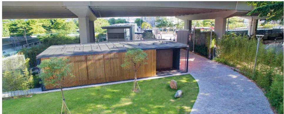
Aerial View from Hing Man Street. Photo: © Architectural Services Department
