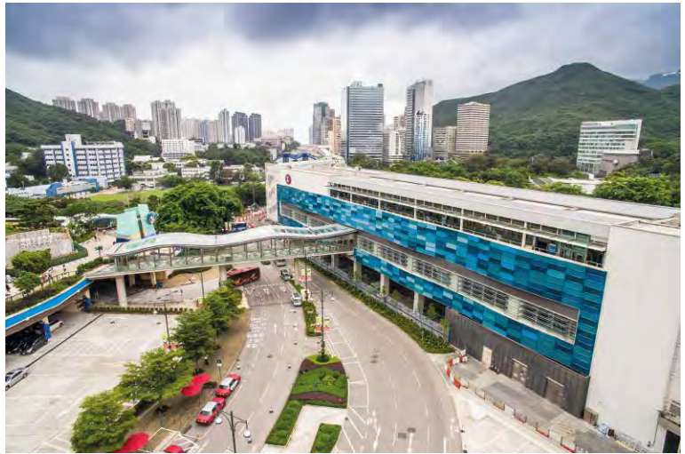
Ocean Park station on the South Island Line. Photo: © Atkins
