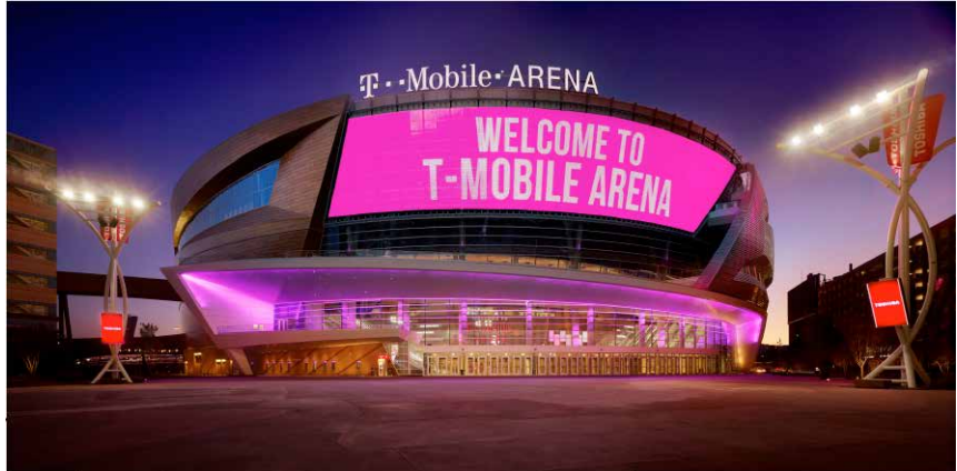
Toshiba Tec's digital signage solution is used at the building of "T-Mobile Arena" located in Las Vegas, USA. Photo: © Toshiba Tec
