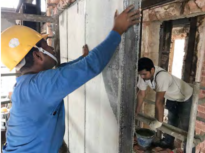
Worker installing vPanel for PSB fire rating test. Photo: © Vodapruf
