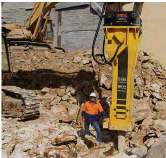
Above: EMC uses an Atlas Copco HB10000 hydraulic breaker for inner city bulk excavation work in Brisbane, Australia.
