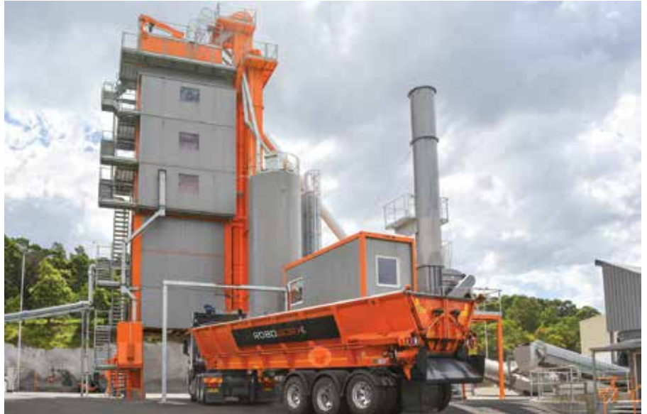
Above, below and bottom: Roadworx has commissioned an Ammann ABA UniBatch asphalt-mixing plant in Wollongong, Australia. The plant has comprehensive environmental features, such as an ability to use recycled asphalt (RAP) and options that dramatically reduce noise and odour.
