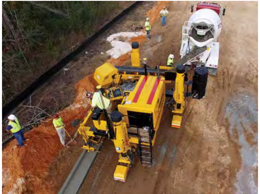
Above: Gomaco's Commander IIIx at work slipforming curb and gutter on a parking lot project.
