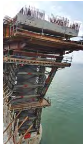
Top, above and right: For the latest phase of the HKZMB project, RMD Kwikform has supplied its formwork and shoring solutions to support the construction of the turnaround facilities in the water, over the marine viaducts.
