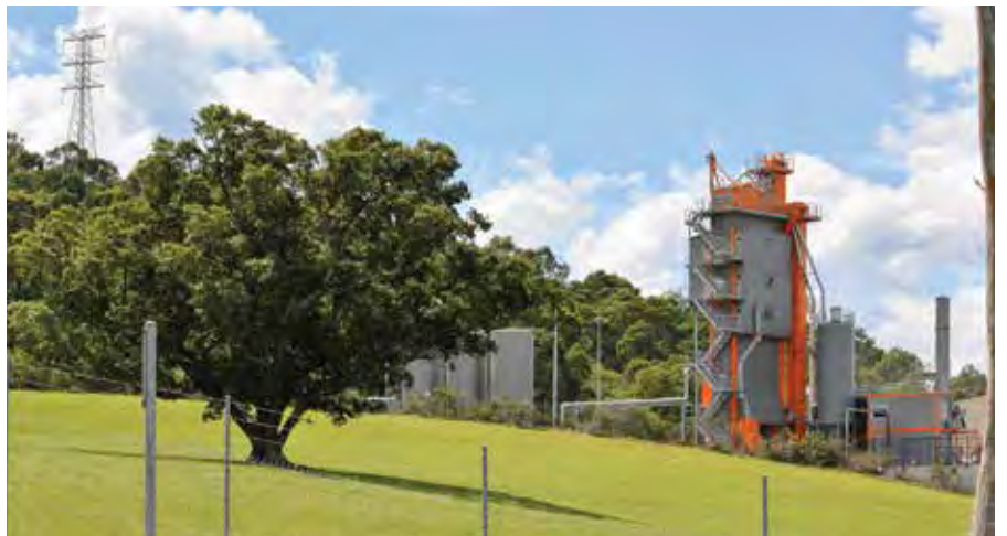
Above, below and bottom: Roadworx has commissioned an Ammann ABA UniBatch asphalt-mixing plant in Wollongong, Australia. The plant has comprehensive environmental features, such as an ability to use recycled asphalt (RAP) and options that dramatically reduce noise and odour.
