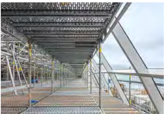
Above: Peri supported the scaffolding contractor with a comprehensive planning solution for the up to 20 m high load-bearing shoring and working scaffold up to 85 m long. Thanks to the lightweight system components, the scaffolding could be erected and dismantled without a crane.
