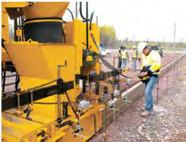
Above: Gomaco's Commander IIIx at work slipforming curb and gutter on a parking lot project.
