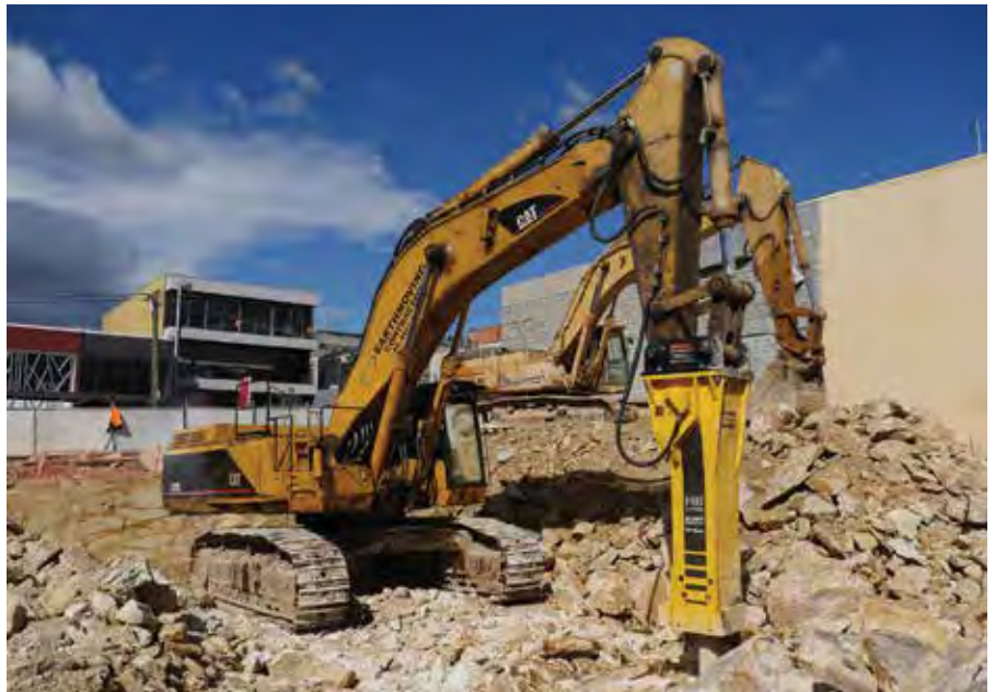
Above: EMC uses an Atlas Copco HB10000 hydraulic breaker for inner city bulk excavation work in Brisbane, Australia.
