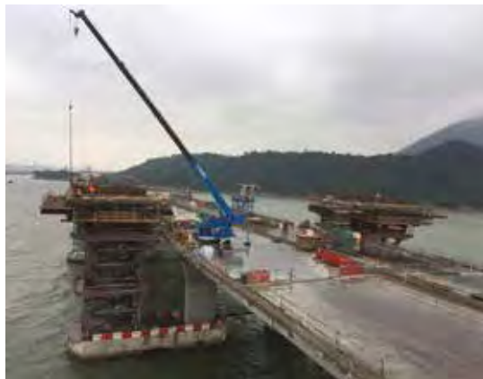
Top, above and right: For the latest phase of the HKZMB project, RMD Kwikform has supplied its formwork and shoring solutions to support the construction of the turnaround facilities in the water, over the marine viaducts.
