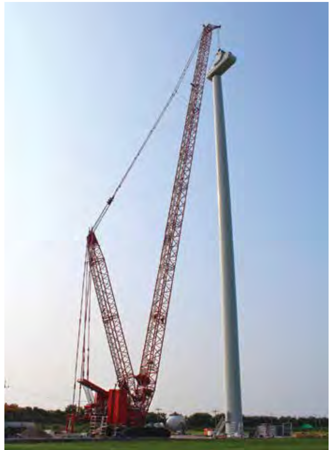
Manitowoc MLC650 crawler crane assembles turbines and lifts heavy components on a new wind farm in South Korea.
