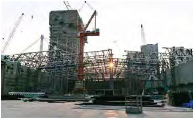
Above and left: To create such long column-to-column spaces, Aurecon designed a support system for the roof structure. This design has the main roof truss supported by fore stays on each side, with these cables then supported on masts around the edge of the building.
