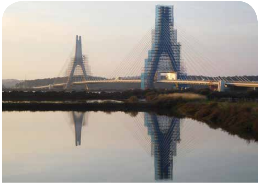
The towers as seen during upgrading work.
