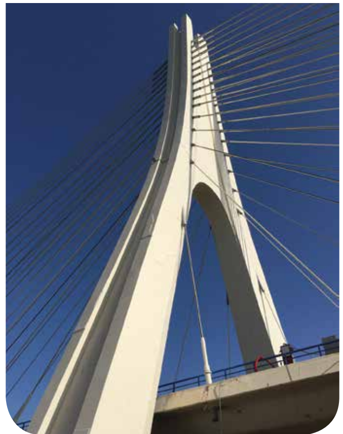
Top: A view of the River Arade Bridge.
