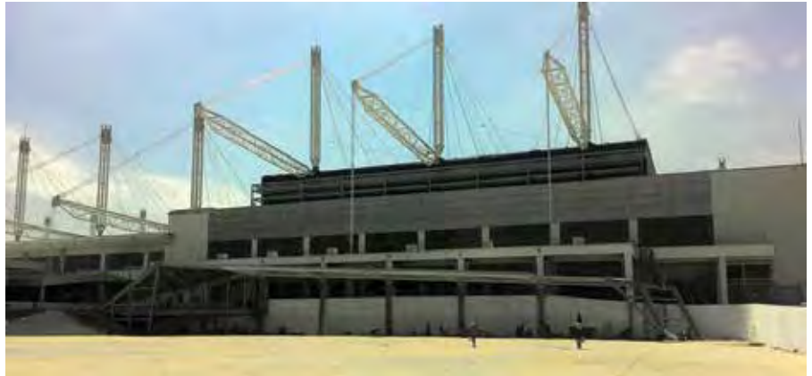
Above: The renovated facility features a new, innovative roof. It is currently believed to be the largest column-free exhibition space in Thailand.
