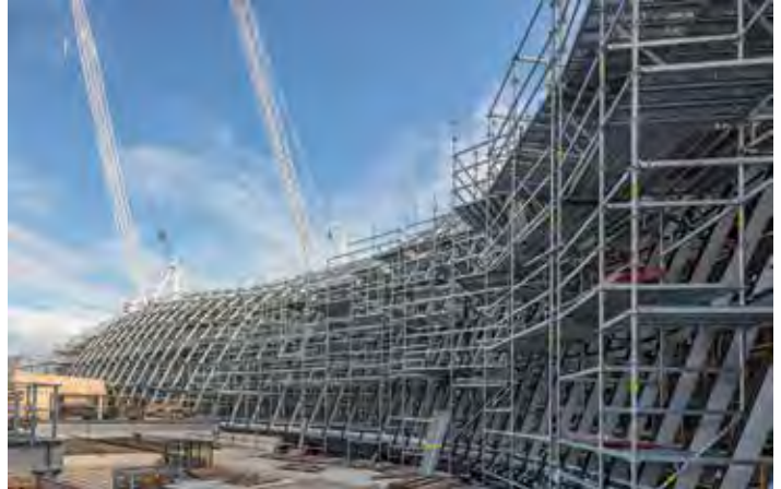
Above: Peri supported the scaffolding contractor with a comprehensive planning solution for the up to 20 m high load-bearing shoring and working scaffold up to 85 m long. Thanks to the lightweight system components, the scaffolding could be erected and dismantled without a crane.
